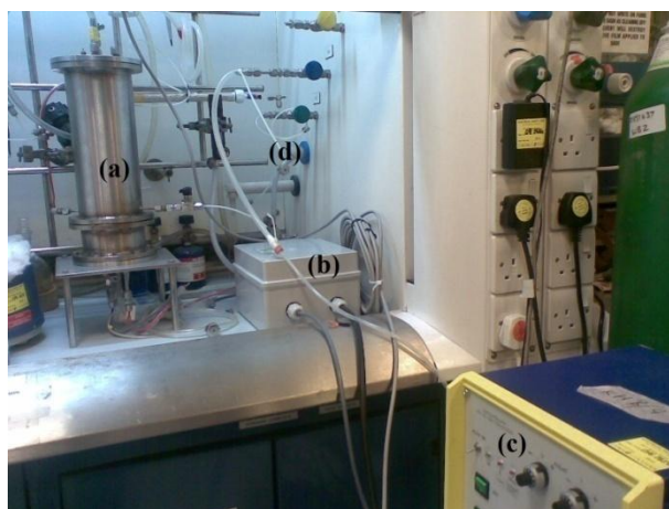
Figure 3.1 General view of reactor (a) with transformer (b), power supply (c) and flow network (d)
