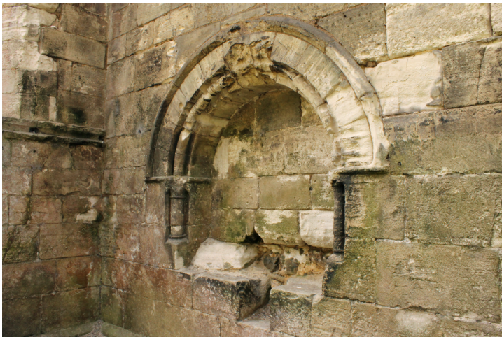
FIGURE 4-11. The recess in the wall of the chapel off the north transept of Roche Abbey, North Yorkshire.
