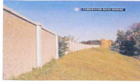
(b) Precast concrete barrier
