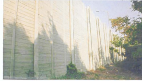
(b) Horizontal noise barrier
