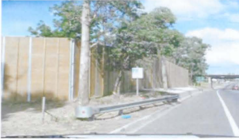
Figure 2.3 (a): Timber noise barrier
