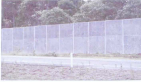
Figure 2.4 (a) Concrete barrier
