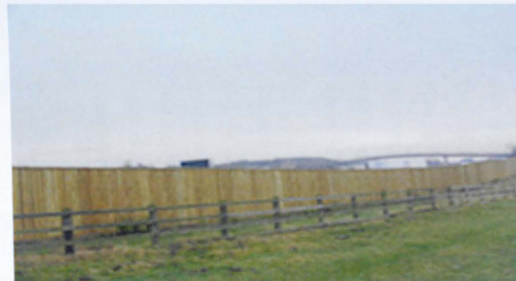
(b) Timber Absorbent Barrier (J27 Northbound M1).
