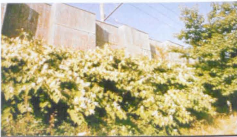
Figure 2.11 Plywood barrier with planting (Source: FHWA)
