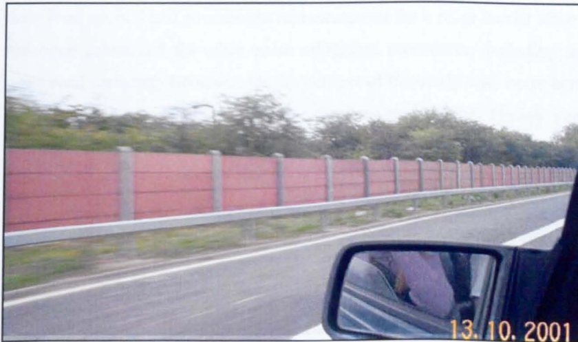
Figure 4.1 Tinsley noise barrier, as seen from M1.
