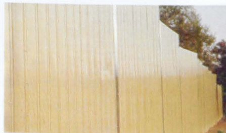
(b) Aluminium noise barrier
