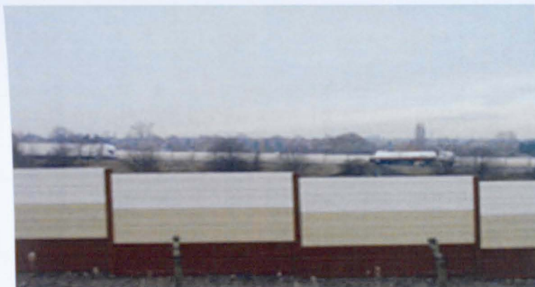
(a) Metal Absorbent Barrier (J27 Southbound M1).
