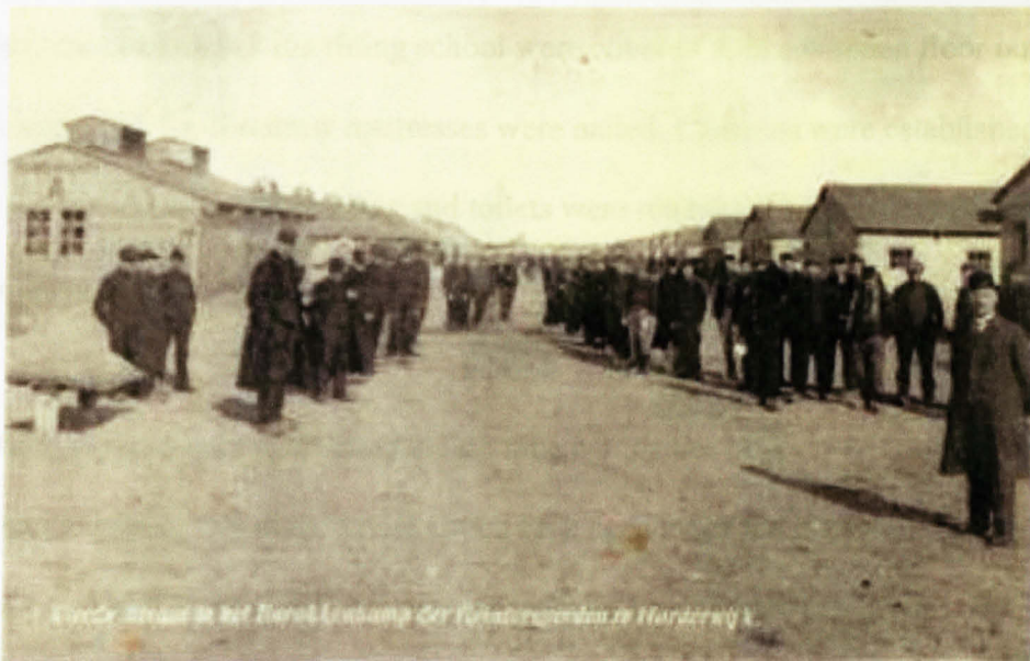
Harderwijk after the construction of permanent accommodation. 31
