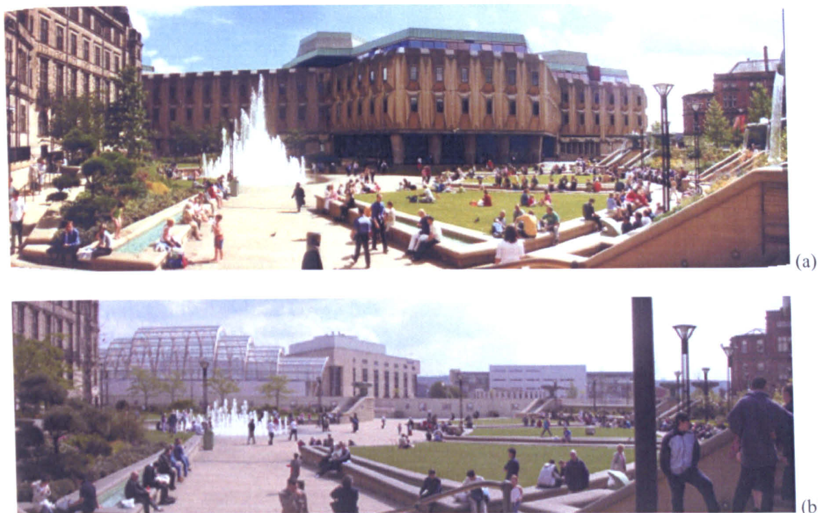
Figure 3.9 The Peace Gardens (a) before demolition of the Town Hall Extension (b) after demolition of the Town Hall Extension
