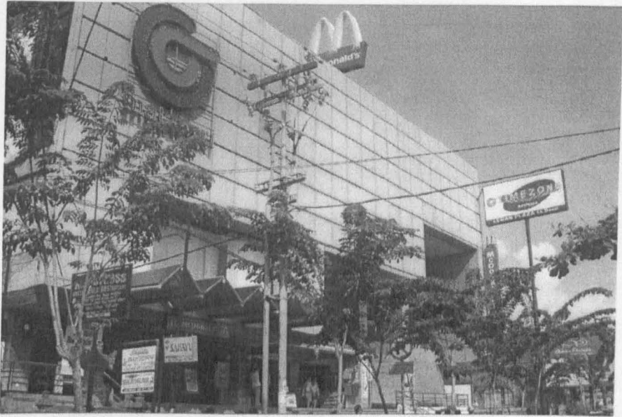
Figure 6.14. The later development of the shop, the architectural form that is chosen does not respect the surroundings. Newer form of shops can disregard the contextual harmony, not respecting the traditional built form. This also represents a weakness in the building regulations
