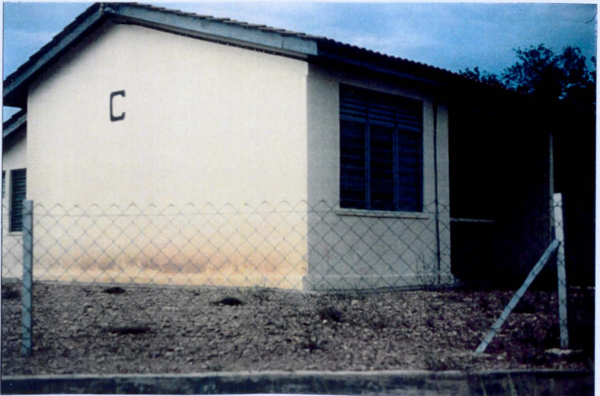
Photograph 8.1: Single Storey Public Low Cost House
