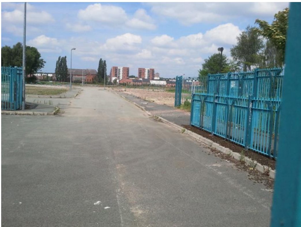
Figure 31: Housing Market Renewal clearance site – Author's own photo
