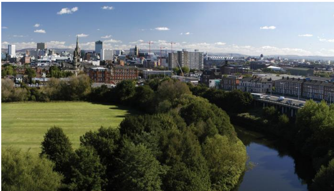
Figure 33: New Broughton Riverside, Aerial view. Source – Countryside properties
