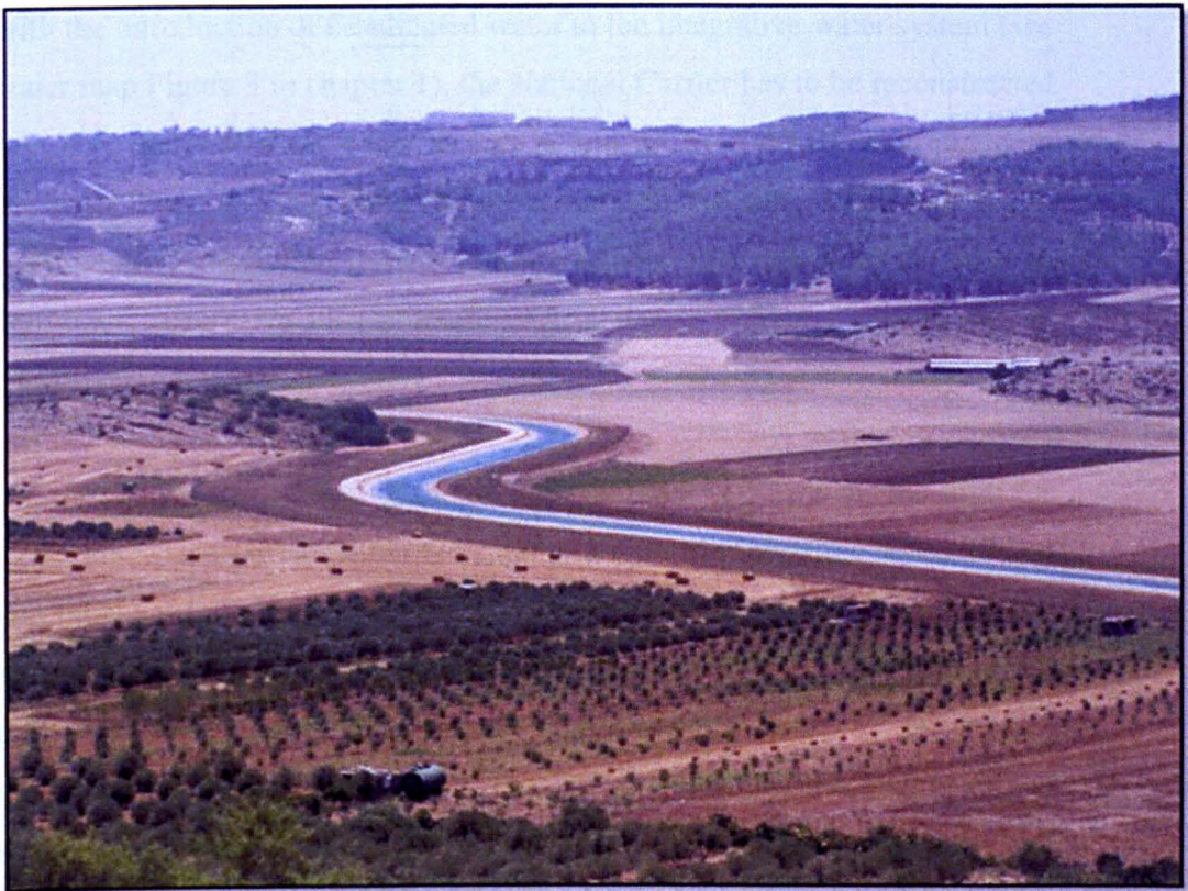
Picture 1 The National Carrier (Northern open section)
