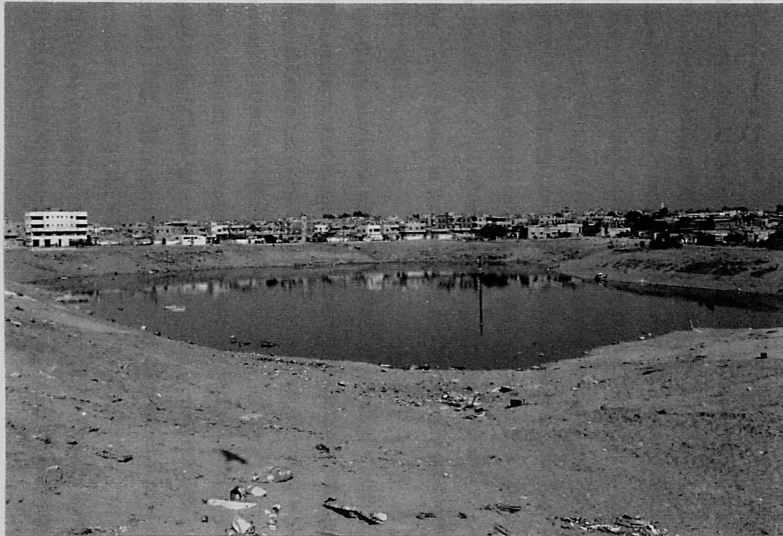
Plate 7.2: Sheikh Radwan project: household sewage water is collected by underground sewage disposal system to the above shown open pool in the north of the project.
