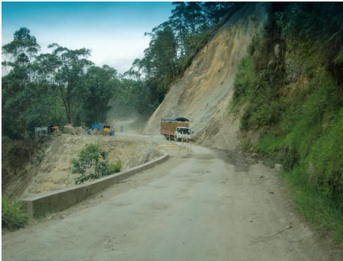
A landslide on the Circumbalar road between Consaca and Sandona (Author, 2012)
