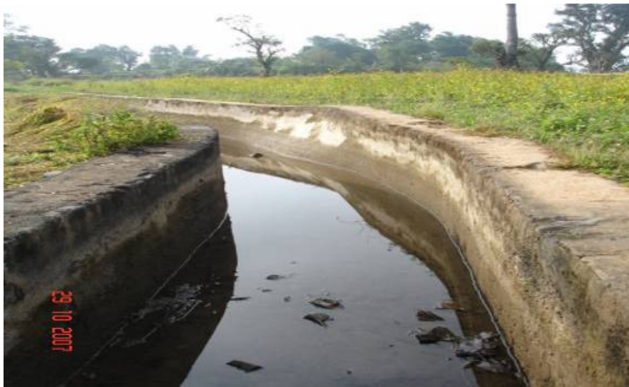
Photo 3.6 Canal Cross Section of JMIS
