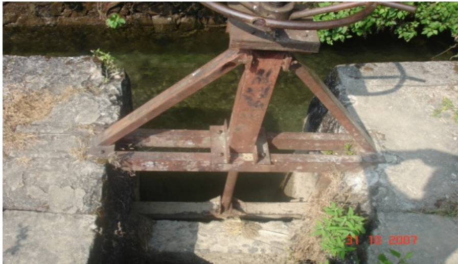
Photo 3.5 Headwork of JMIS
