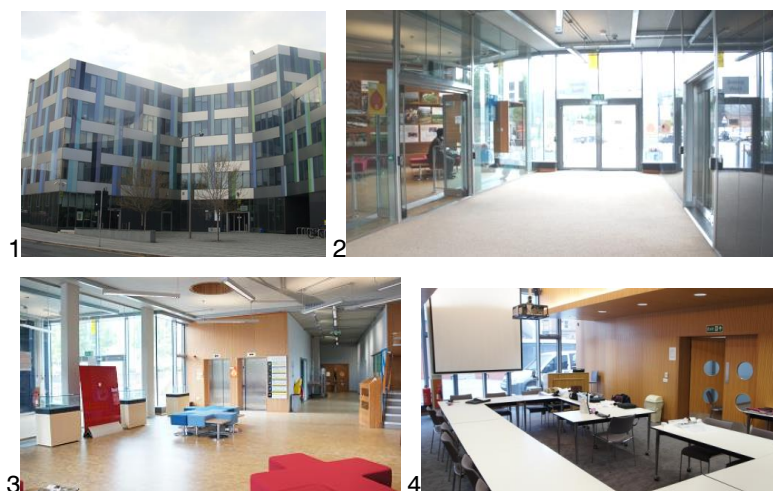
Figure 3-11 Jessop West Building:1) exterior, 2) entry doors (draught lobby), 3) circulation space, 4) seminar room
