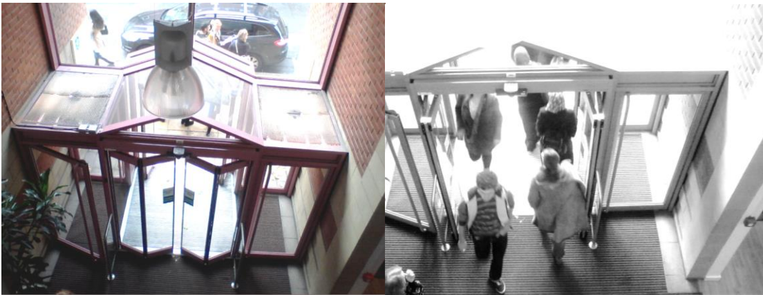
Figure 2-14 Transitional space Type 1, lobby area connecting the exterior and interior environment. Sr Henry Stephenson Building, The University of Sheffield, UK.
