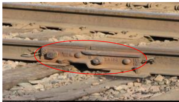
Fig. 1:9- Compromise Joint Bar [19].
