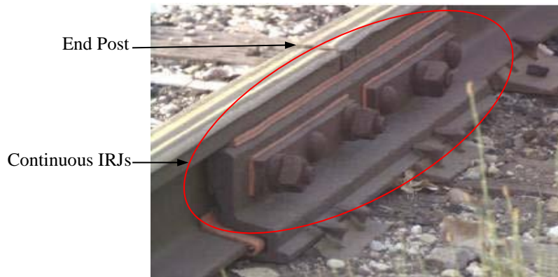
Fig. 1:17- Continuous Insulated Rail Joints [14].
