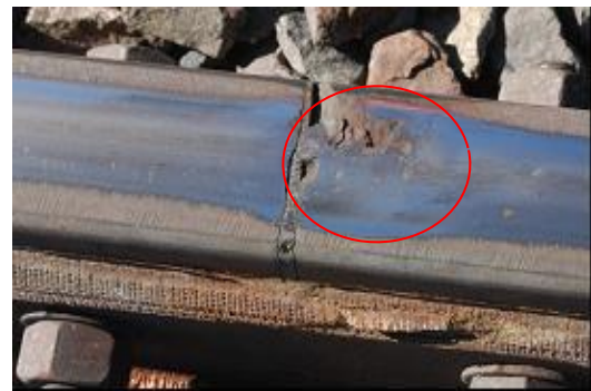
Fig. 1:20- Rail End Battering [32].
