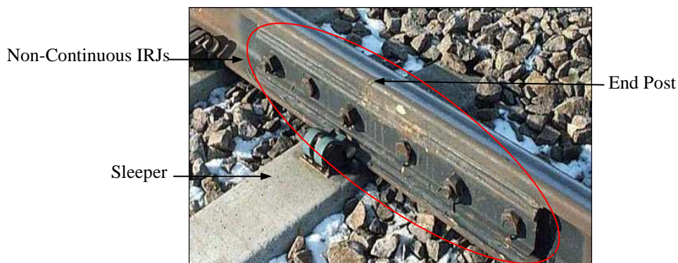
Fig. 1:18- Non-Continuous Supported IRJs [28].
