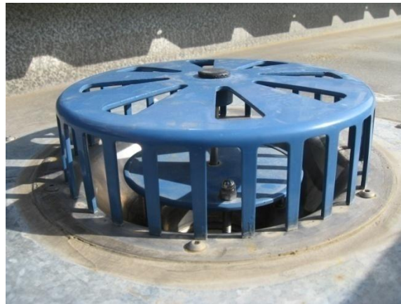
Figure 3.9 Siphonic Outlet Installed within the Gutter
