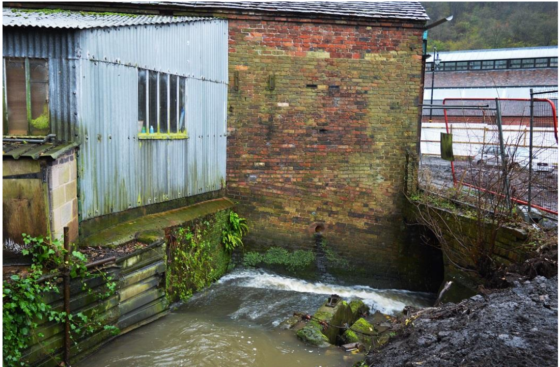
Fig. 6.07. Coalbrookdale Lower Forge. A view south along the watercourse where it turns sharply east to return to the Coalbrook. The nineteenth-century brick building occupies the footprint of earlier structures shown on historic mapping. On the near bank in the foreground is the twentieth century hydro-electric emplacement. Source: Clwyd-Powys Archaeological Trust, photograph 3931-0036.
