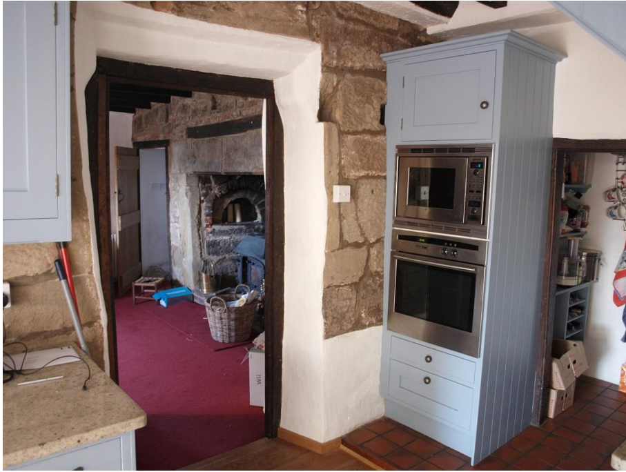
Fig. 5.13. The Lodge: possible original external door in the east wall. Source: author.
