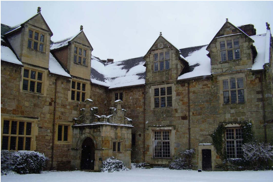
Fig. 5.03. Madeley Court: courtyard elevations of the north (left) and east (right) wings, showing Phase 2 windows and Phase 3 porch.
