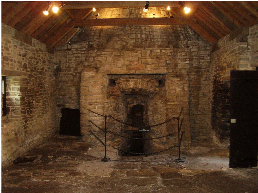
Fig. 7.08. Derwentcote steel furnace: the entrance to the reverberatory chamber, with the stokehole below and the ashpit beneath that. Source: author.
