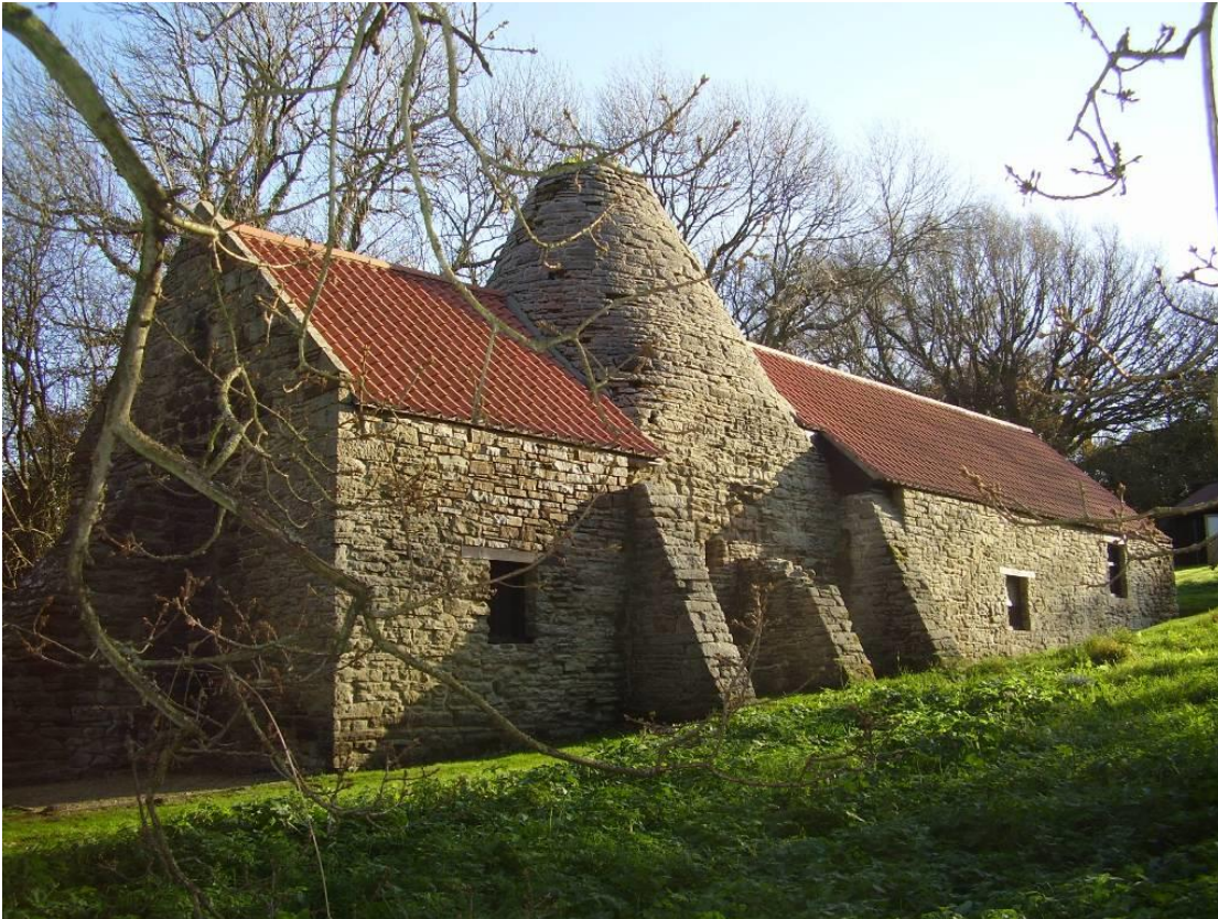
Fig. 7.05. Derwentcote steel furnace: the stone-built cementation furnace and ancillary buildings of 1733, echoing the earlier arrangement at Madeley. Source: author.
