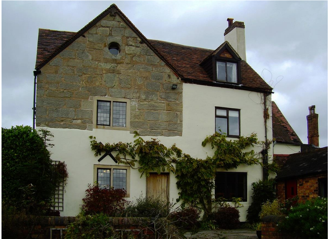
Fig. 5.11. The Lodge: south-facing elevation. Source: author.
