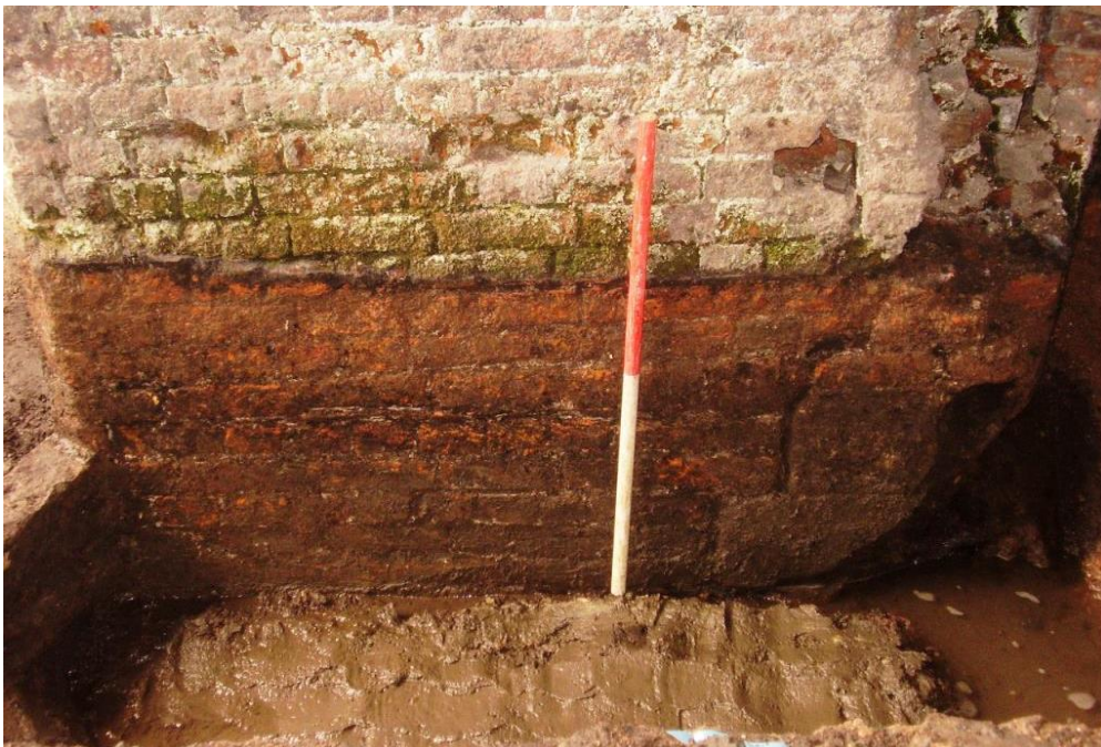
Fig. A3.04. Archaeological excavations at the Coalbrookdale Old Furnace in 2009. Trench 4, showing the below-ground foundation of the 1658 furnace structure. For location see Fig. A1.05 on the following page.
