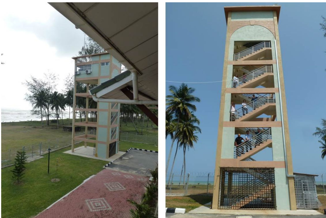
Figure 5.10: Photo of the location of the tower with respect to the main building and sea (left) and a full image of the tower (right)
