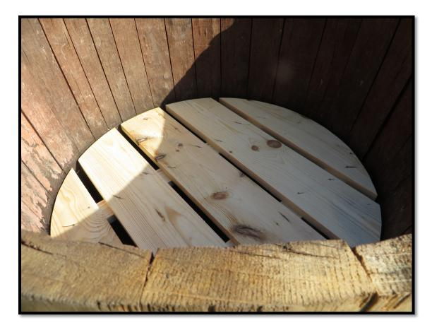
Figure 5: wooden boards to prevent tap blockage
