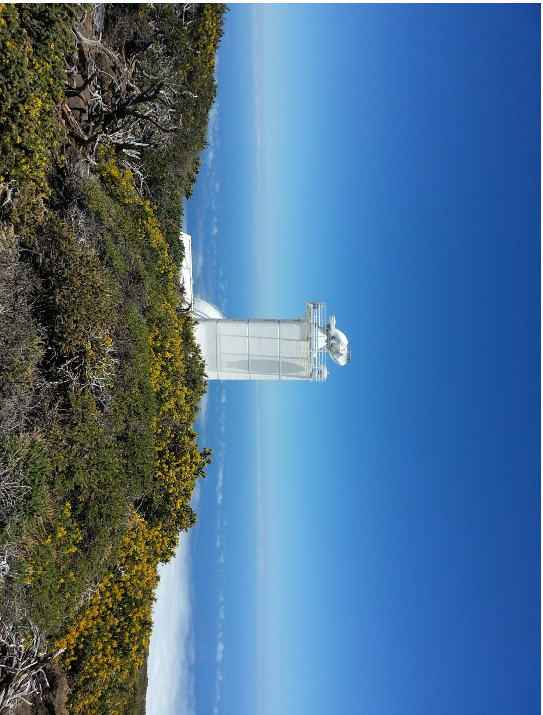
Fig. 2.1 An image of the Swedish Solar Telescope taken from a ledge near the caldera on the island of La Palma that is part of the Canary Islands. The primary mirror housing can be seen at the top of the image, while the tower that conceals the vacuum tower can be seen beneath it. Copyright goes to the author.
