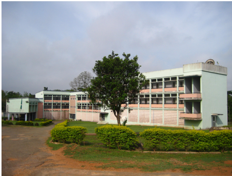
Figure 2: Photo of Nigerian National Archive, branch Ìbàdàn
