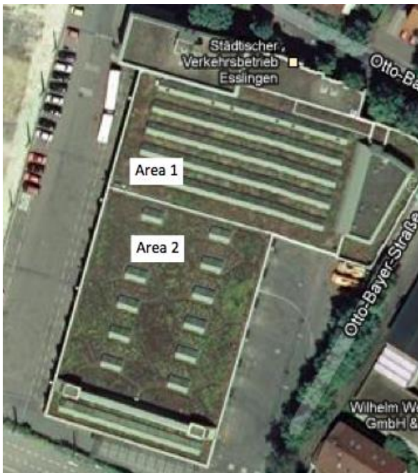
Figure 2.5. Aerial view of the two roofs at Esslingen Verkehrsbetrieb. Image courtesy Google Maps.
