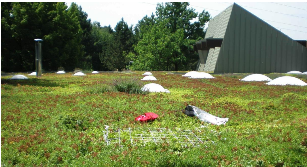
Figure 2.4. Facing north on the roof at Pliensaufriedhof.
