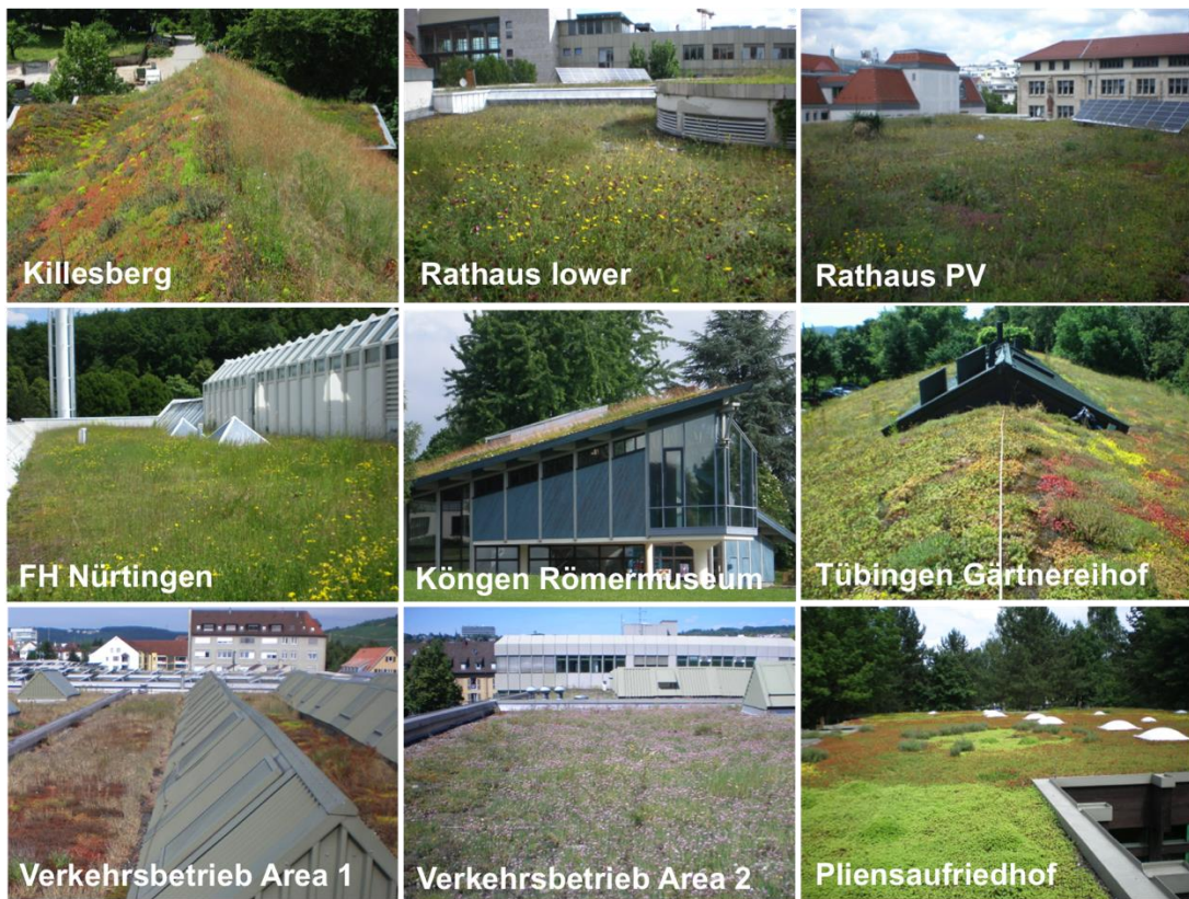
Figure 2.3. The nine EGRs sampled in southwest Germany were constructed between 1977-1991 and are arranged in order of increasing age from the top-left.
