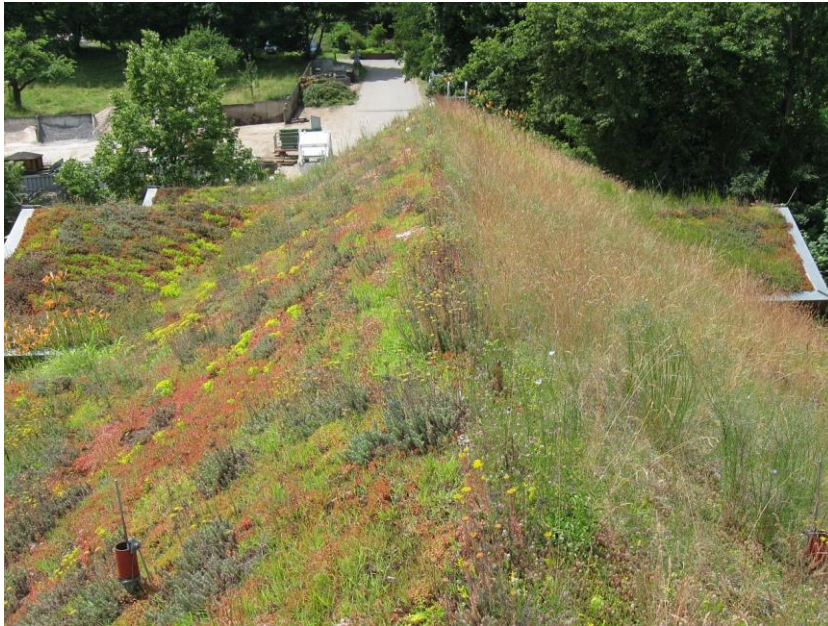
Figure 2.10. The roof at Killesberg features a clear north-south gradient.
