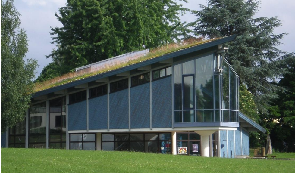
Figure 2.7. The Römermuseum in Köngen features a south-facing roof (left) and a smaller, lower roof facing north (right).
