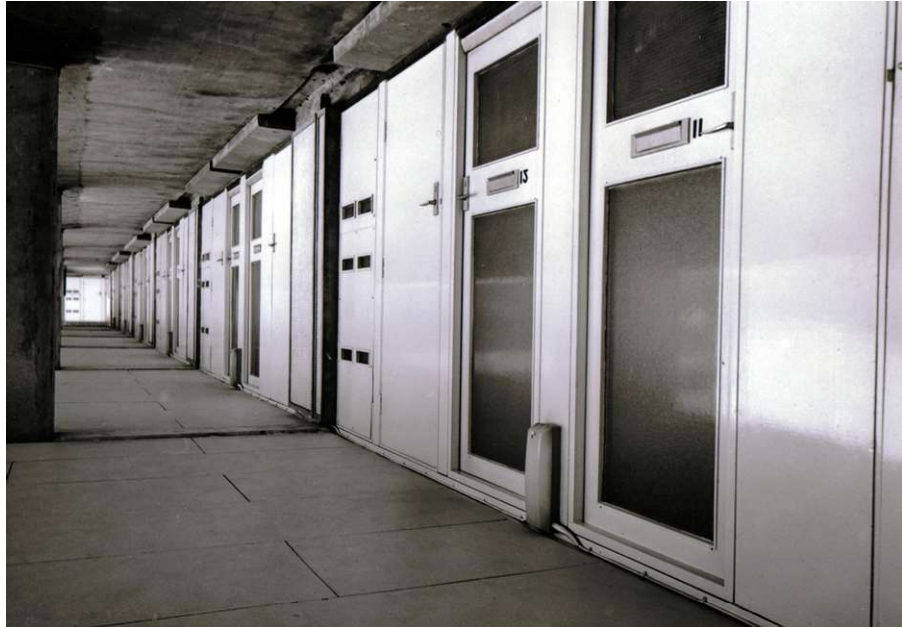
Fig. 1.5 One of the raised walkways at Hunslet Grange in 1968, showing the entrances to the flats. [Clifford Stead, flickr, https://www.flickr.com/photos/cliffordstead/albums , 15 September 2015]
