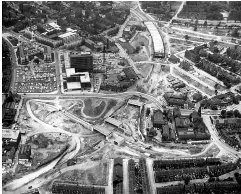
Fig. 3.4 The construction of the inner ring road on the northern fringe of central Leeds in the late 1960s. The Civic Hall and Leeds General Infirmary can be seen in the top left. To the left of the line of the inner ring road is the site of Leeds Polytechnic, while to the right is the expanding Leeds University precinct. Woodhouse Lane, the beginning of the A660, crosses the ring road on the bridges in the centre of the image. [Leeds Library and Information Services, http://www.leodis.net/ , accessed 17 February 2015]
