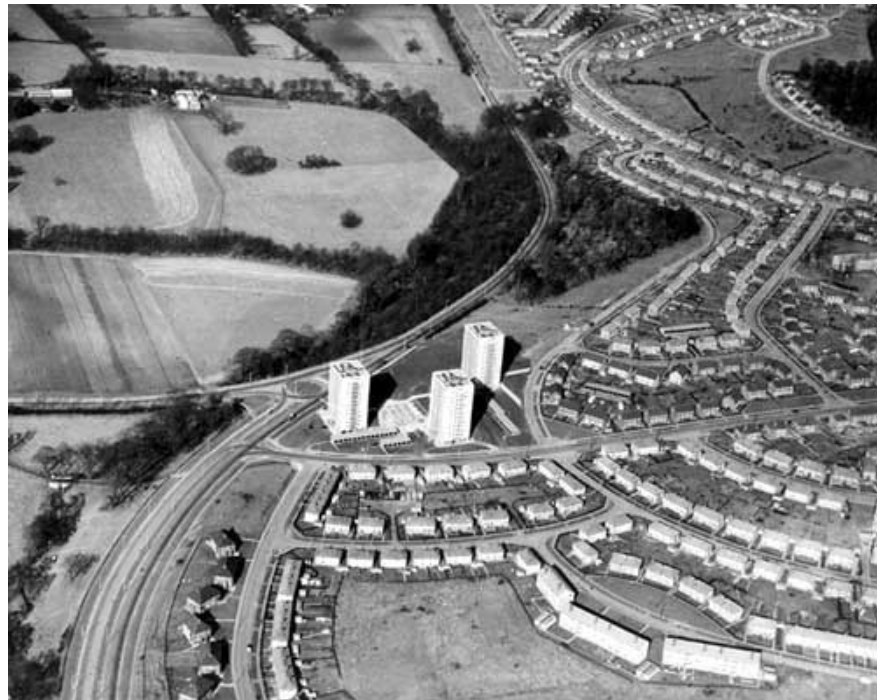
Fig. 2.3 Part of the council's Seacroft estate abutting open countryside on the edge of east Leeds in 1963. [Leeds Library and Information Services, http://www.leodis.net/ , accessed 10 September 2015]
