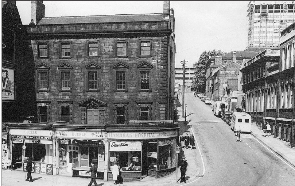
Fig. 3.3 North Street and Hartley Hill on the edge of Leeds city centre. Almost all the buildings in this image (except the old public dispensary on the far right) were demolished for the construction of the inner ring road and car parking [‘Leeds Back in the Day,’ Facebook group, https://www.facebook.com/LeedsBackInTheDay/photos_stream , accessed 10 September 2015]
