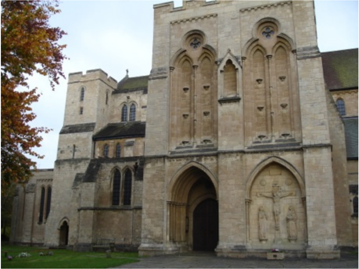
Figure 2.29- North transept (exterior), St Wilfrid's, Harrogate
