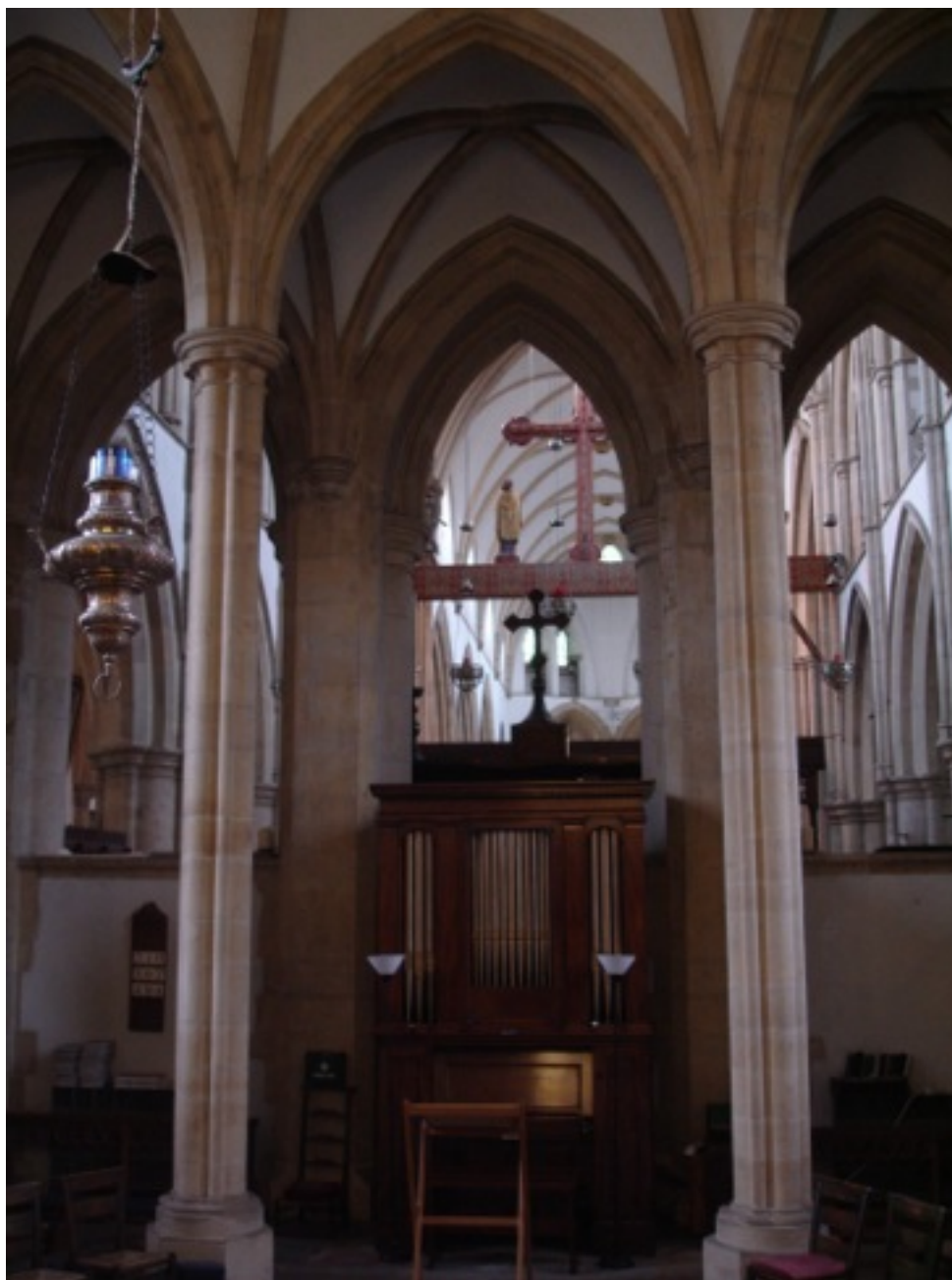
Figure 2.33- 'Feretory', Lady Chapel, St Wilfrid's, Harrogate 'The use of tall thin piers creates a feretory just behind the high altar and one can imagine an elaborate reliquary being enshrined behind it, the Lady Chapel providing a processional route through the building.'
