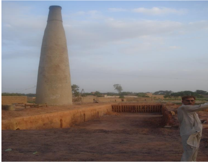
Figure 4.5: Chimney in the middle of the trench
