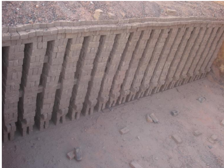
Figure 4.4: Stocking of bricks inside the trench before firing
