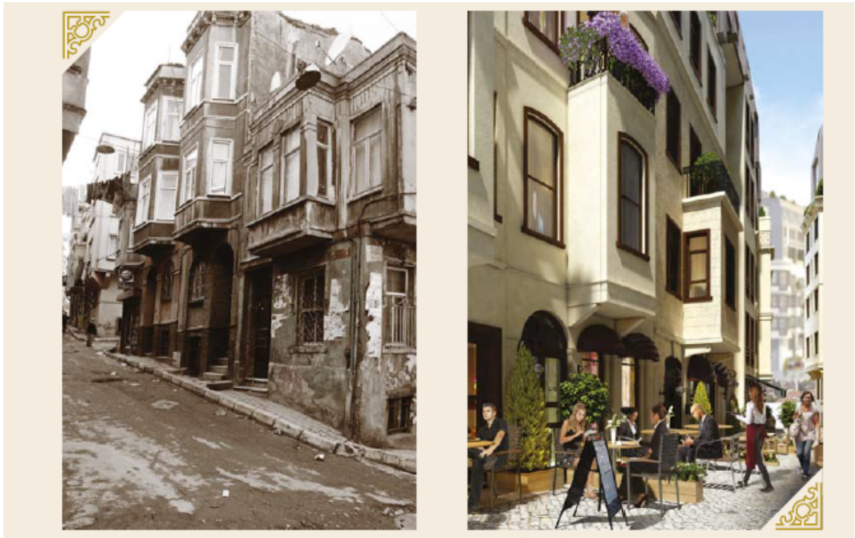
Photo 8.8: Comparison between current and project Tarlabasi, Eski cesme Street, Tarlabasi Urban Renewal Project Leaflet, prepared by Gap Insaat, 2013
