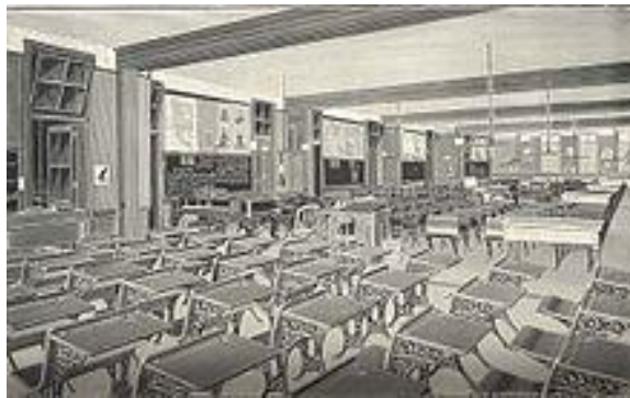
Figure 4: Classrooms in 1897 at the Francis M. Dre 1
