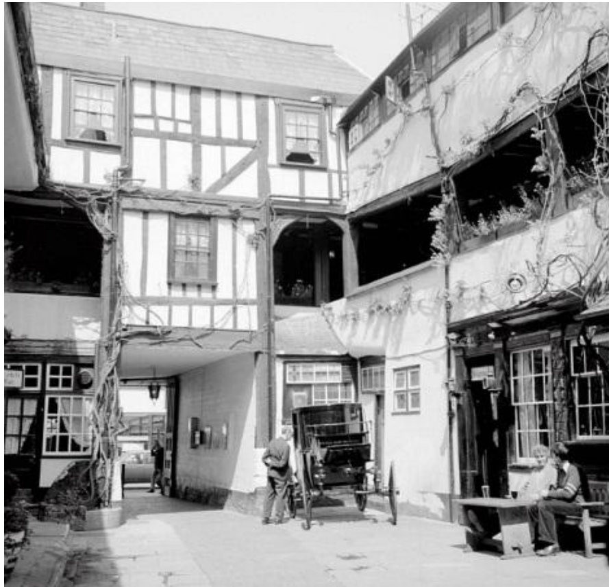
Fig. 9 A first-floor gallery at the New Inn, Gloucester, c.1973 506
