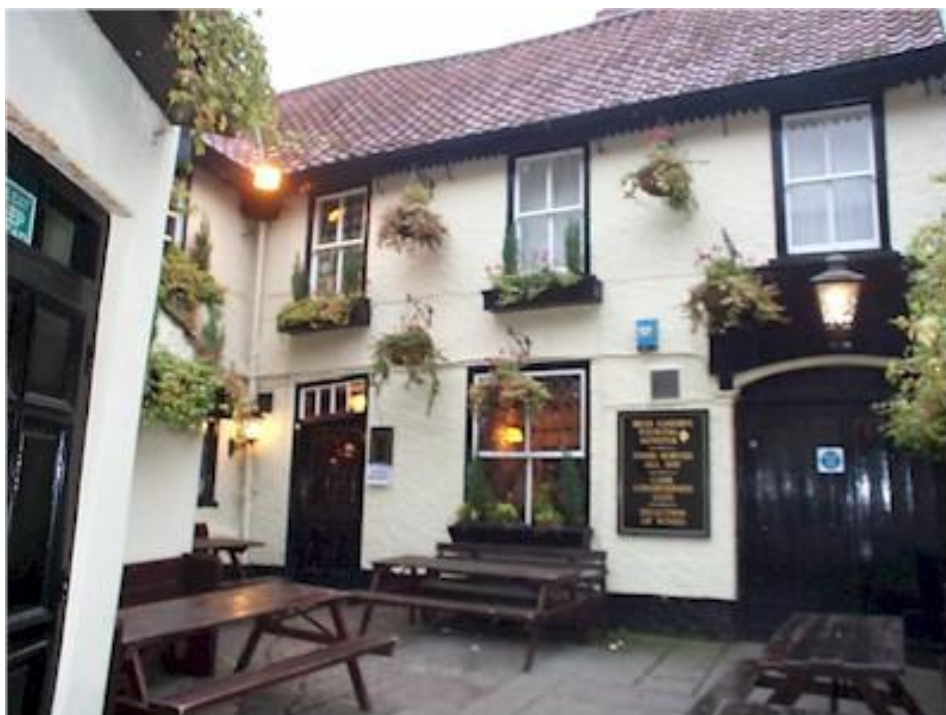
Fig. 8 The two right-angled ranges of the “Starre Inne”, situated around its courtyard 505
