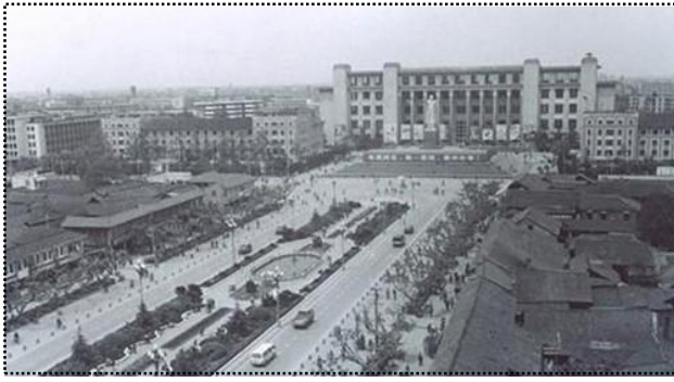
Figure 3.20 Photograph of Tianfu Square in Chengdu in 1985 (Huang, 2008)
