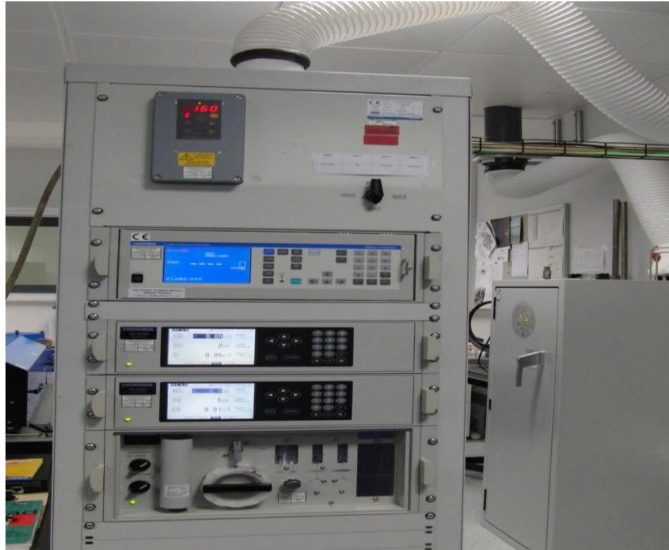
Figure 3.5 The photograph of the rack-mounted HFID, VA-3000 and the VS-3000 systems.
