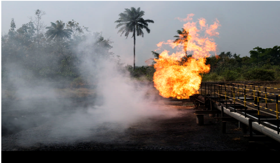
Figure 1.2 Photograph of a ground flare (Lohuizen,2008).
