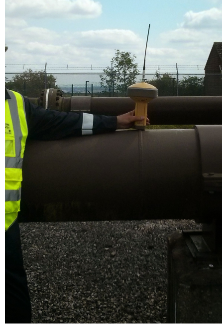
(b) Locate a weld by the rover.
