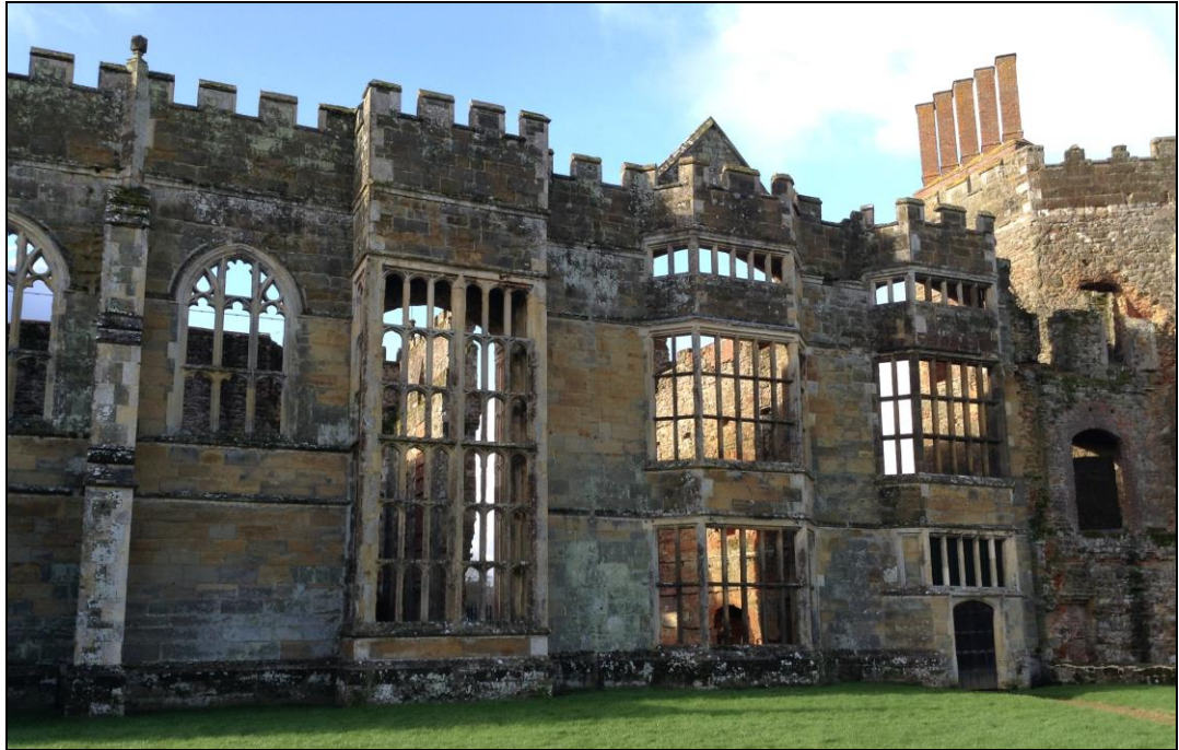
Figure 6: Eastern Range, windows from the great hall.
