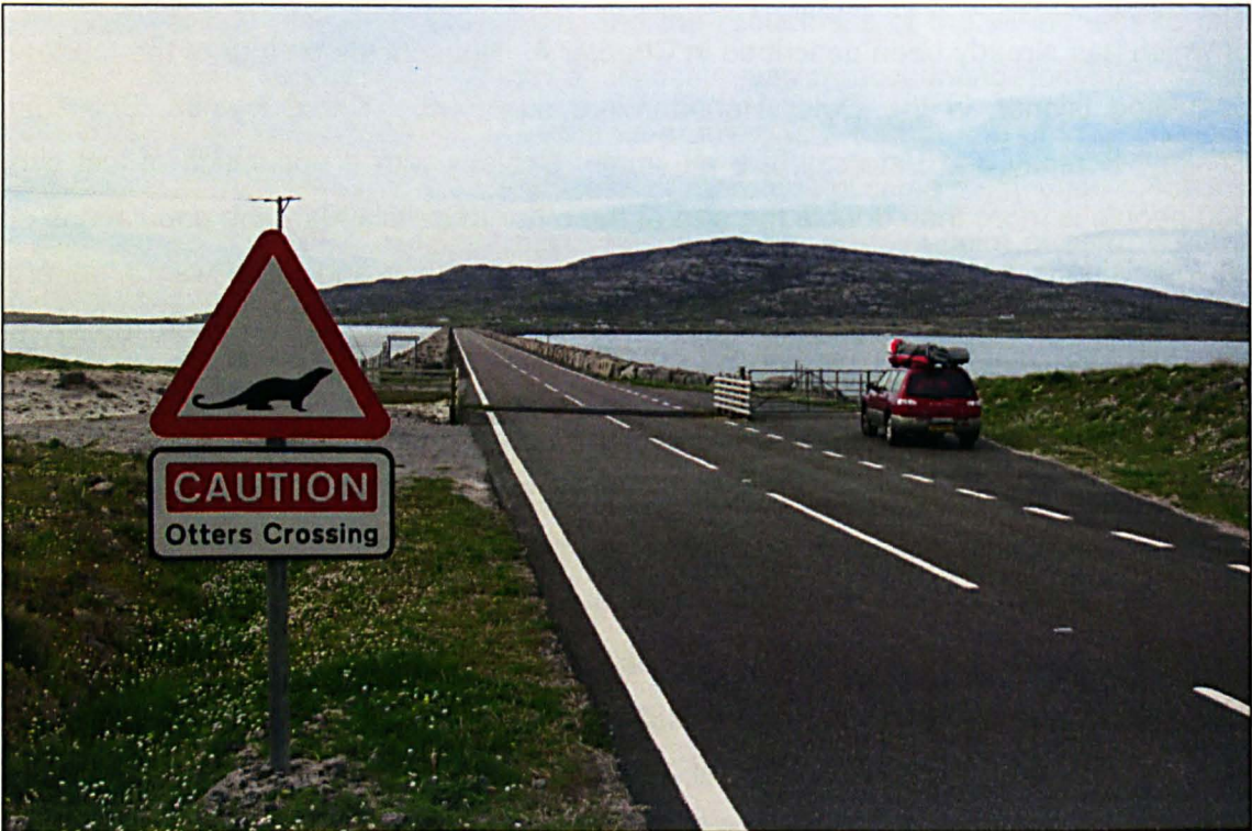
Figure 6.2: Eriskay Causeway (from Eriskay looking north towards South Uist)
