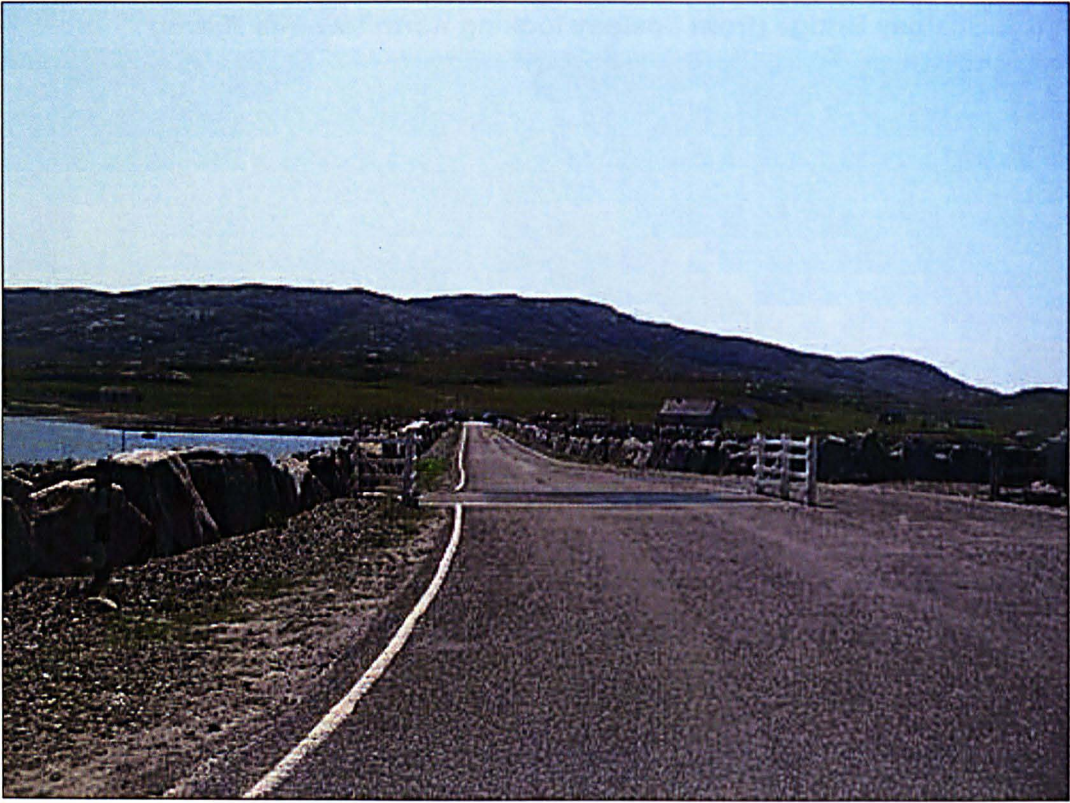
Figure 6.4: Vatersay Causeway (from Barra looking south towards Vatersay)
