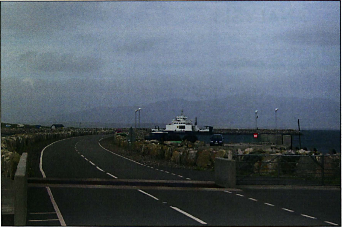
Figure 6.1: Berneray Causeway and Sound of Harris Ferry (from North Uist looking north towards Berneray)
