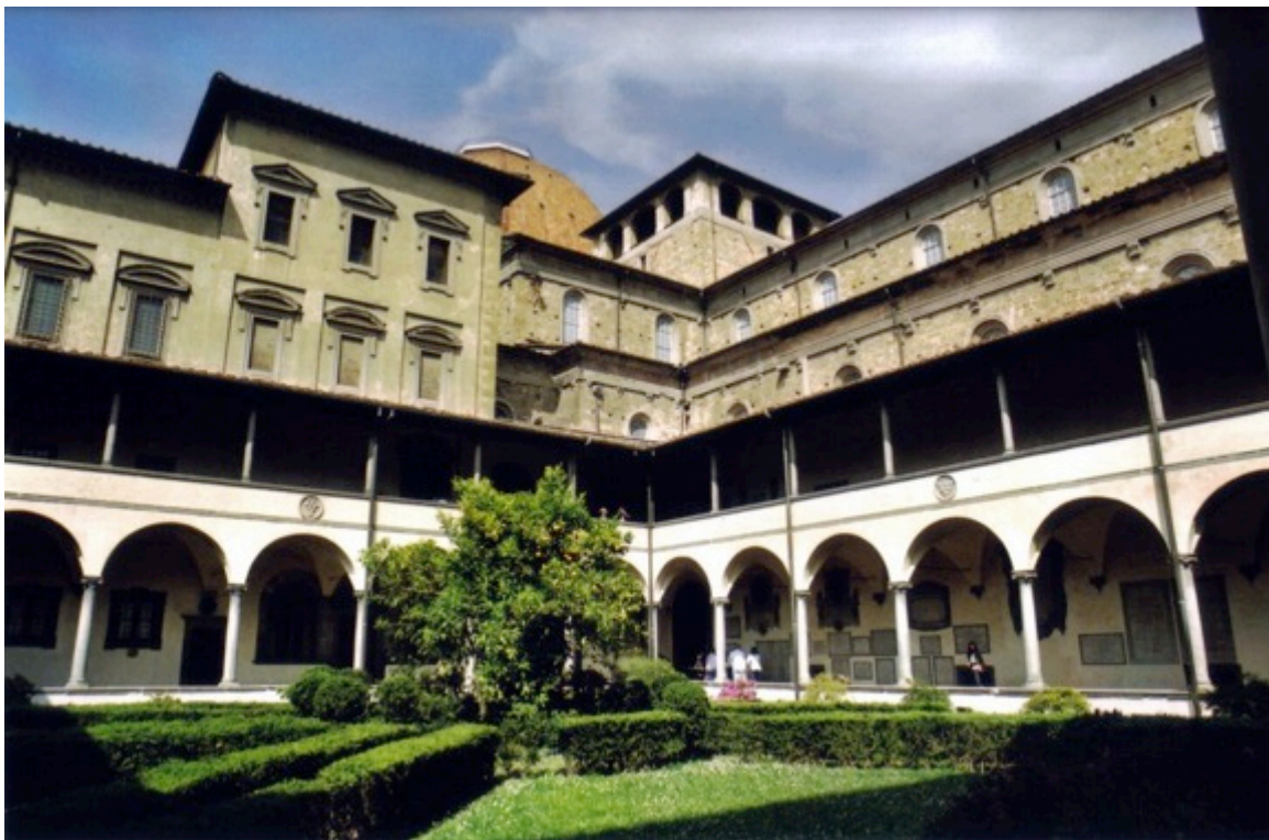
Figure 77: Cloister, San Lorenzo, Florence
