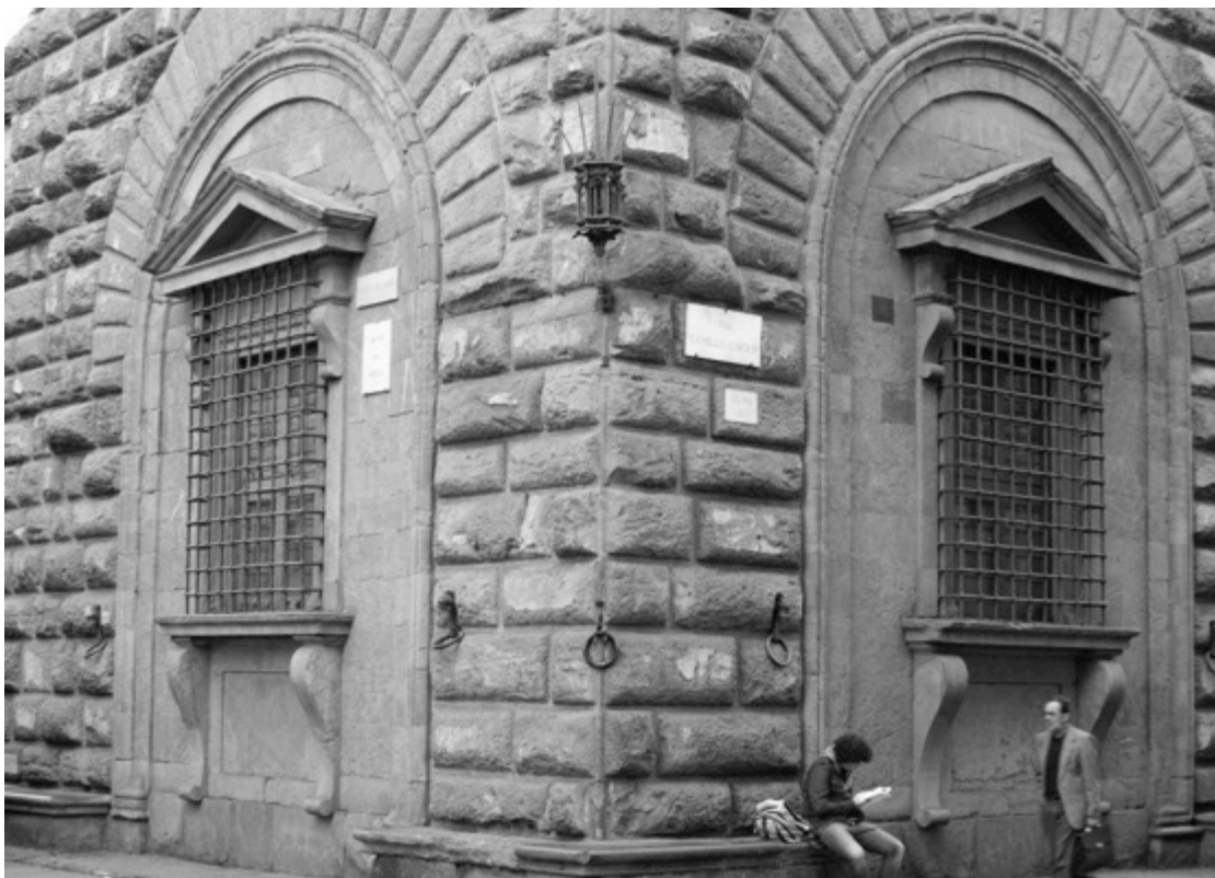
Figure 71: Corner loggia, Palazzo Medici, Florence, c. 1444
