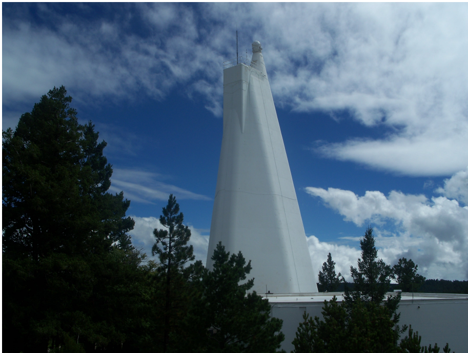
Figure 2.3: The tower section of the DST. The telescope also consists of an underground section, which goes deeper than the height of the tower.
