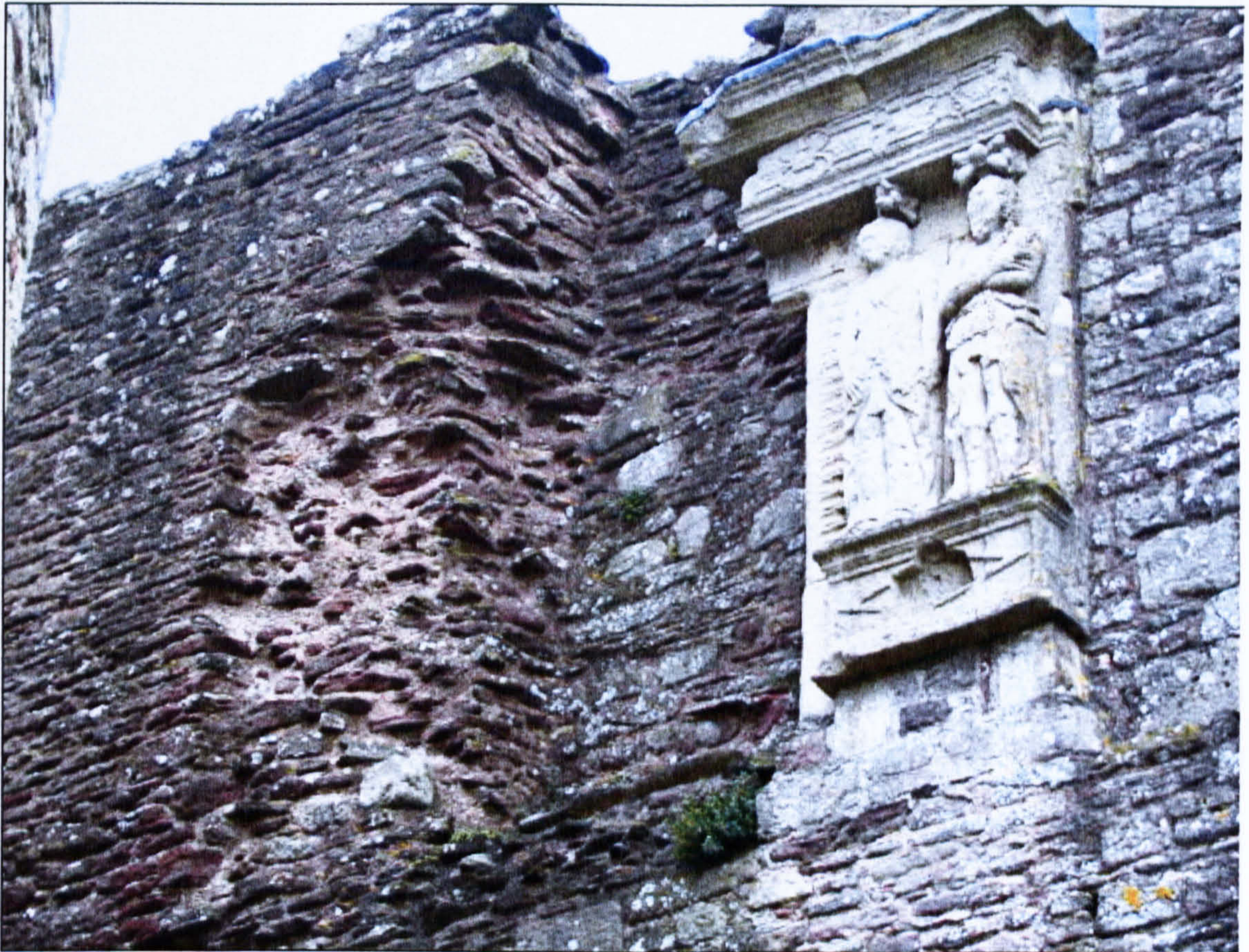
Figure 4.52 Remnants of a fireplace still in situ in the Long Gallery, Raglan Castle (Wales).
