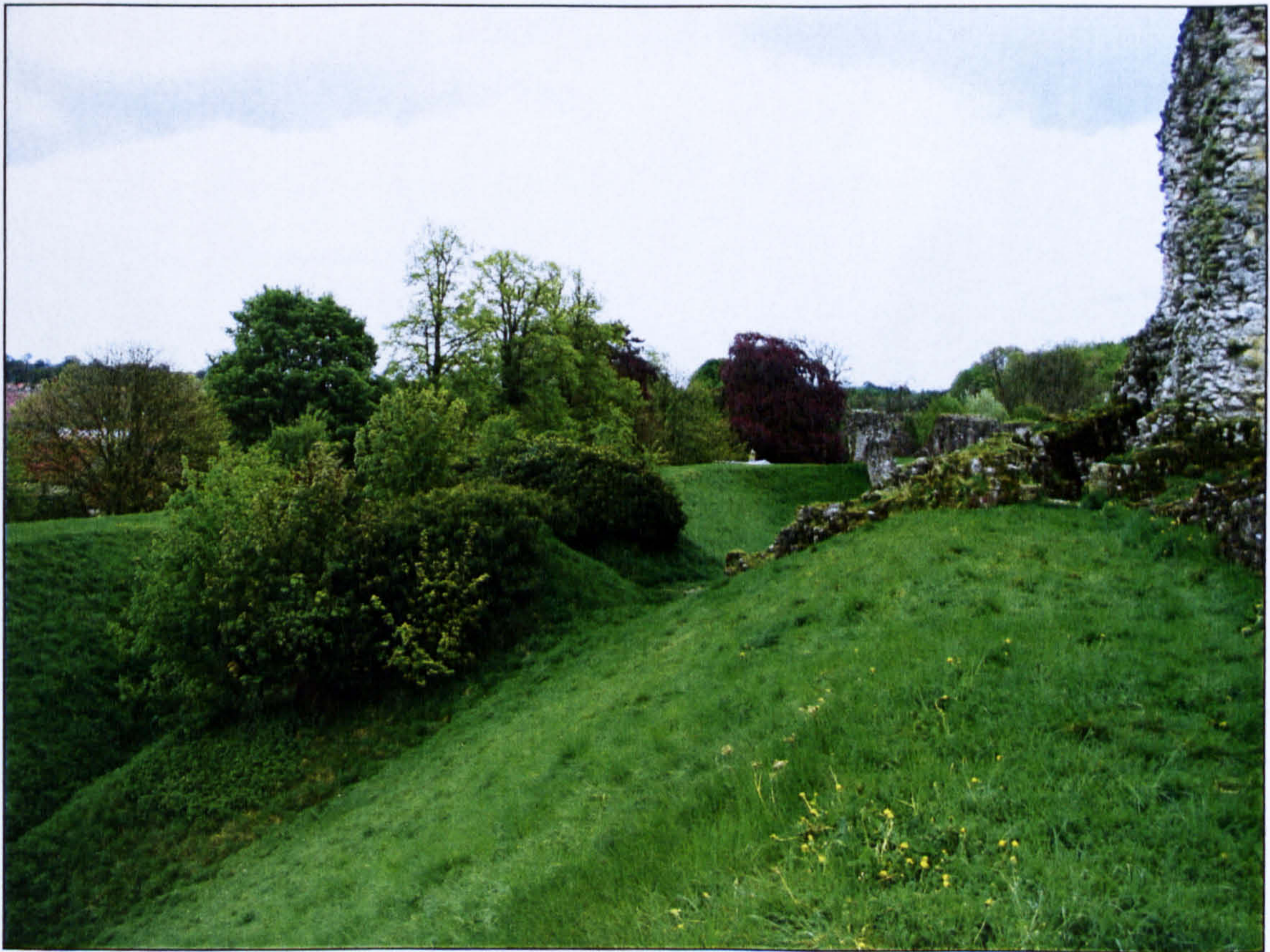
Figure 5.51 Vegetation covered debris at the foot of the East Tower.
