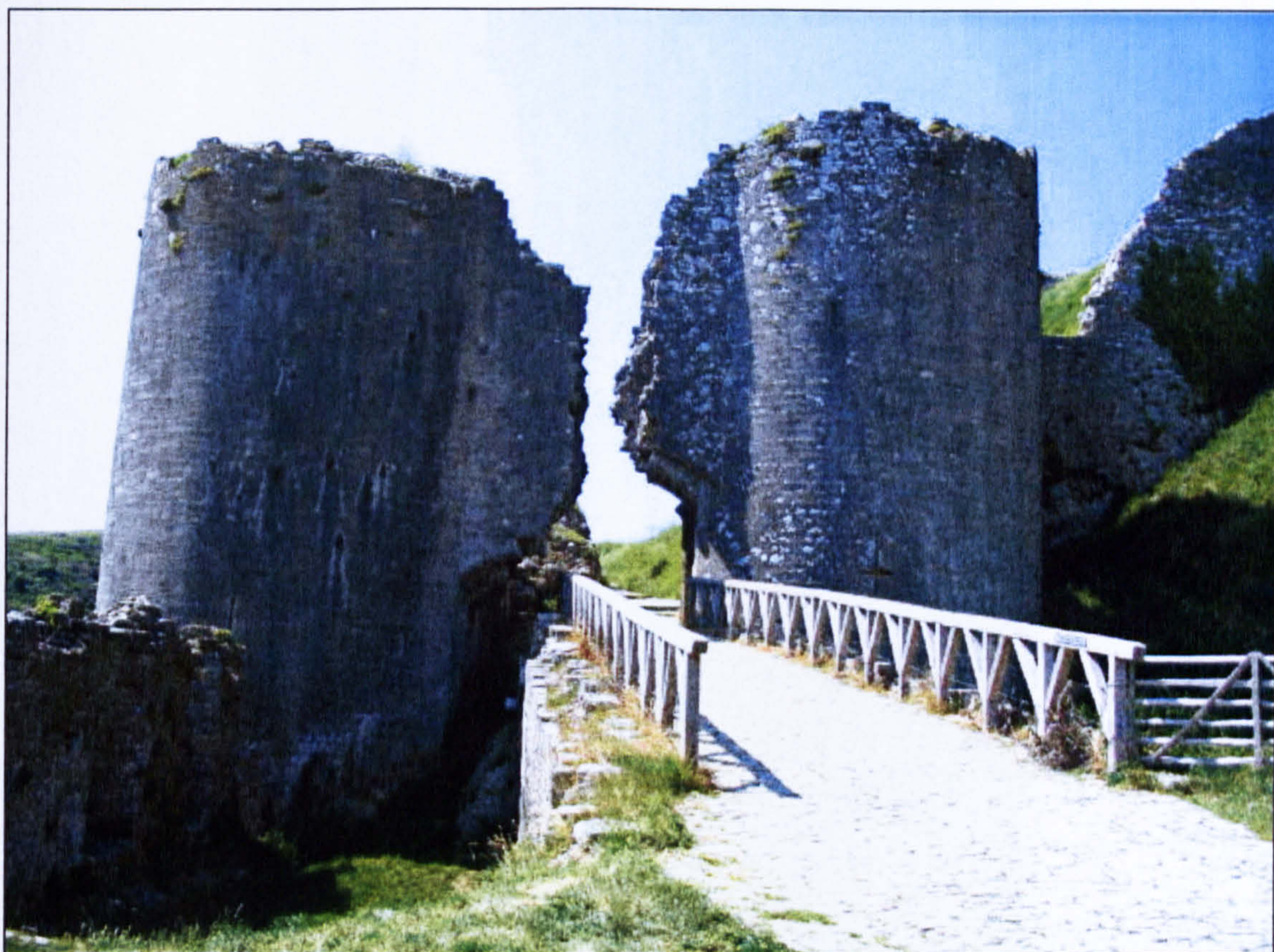
Figure 5.18 Southwest Gatehouse, looking northwest.
