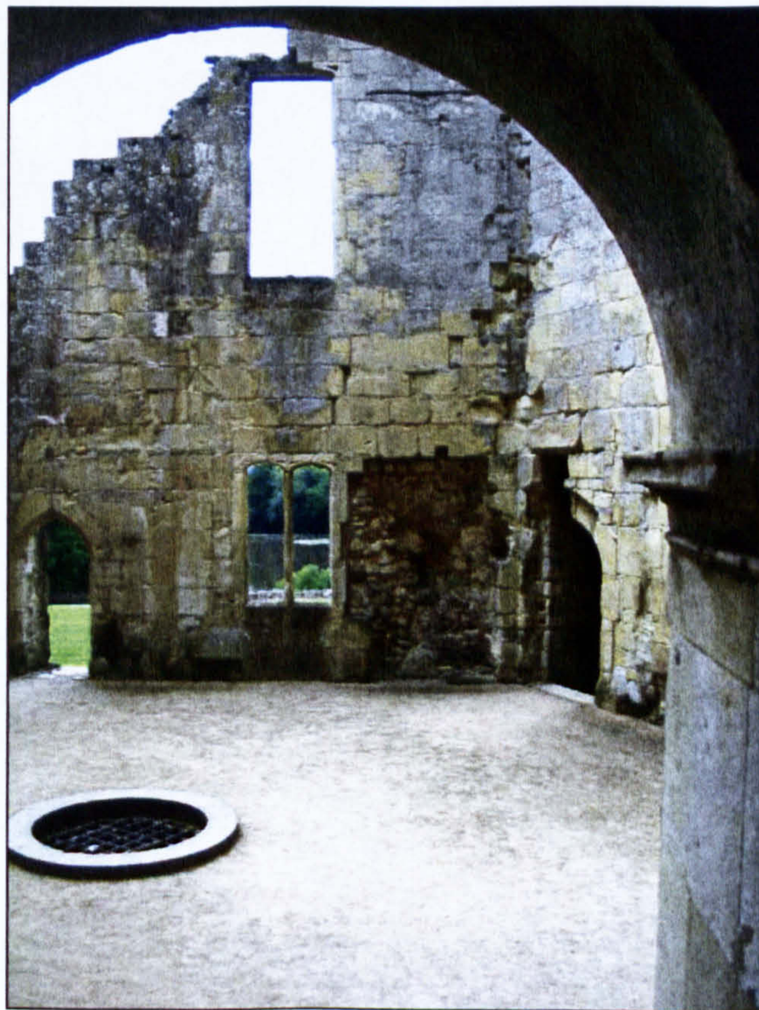
Figure 4.60 View from the Great Hall staircase of secondary damage pattern at Old Wardour Castle (Wiltshire).
