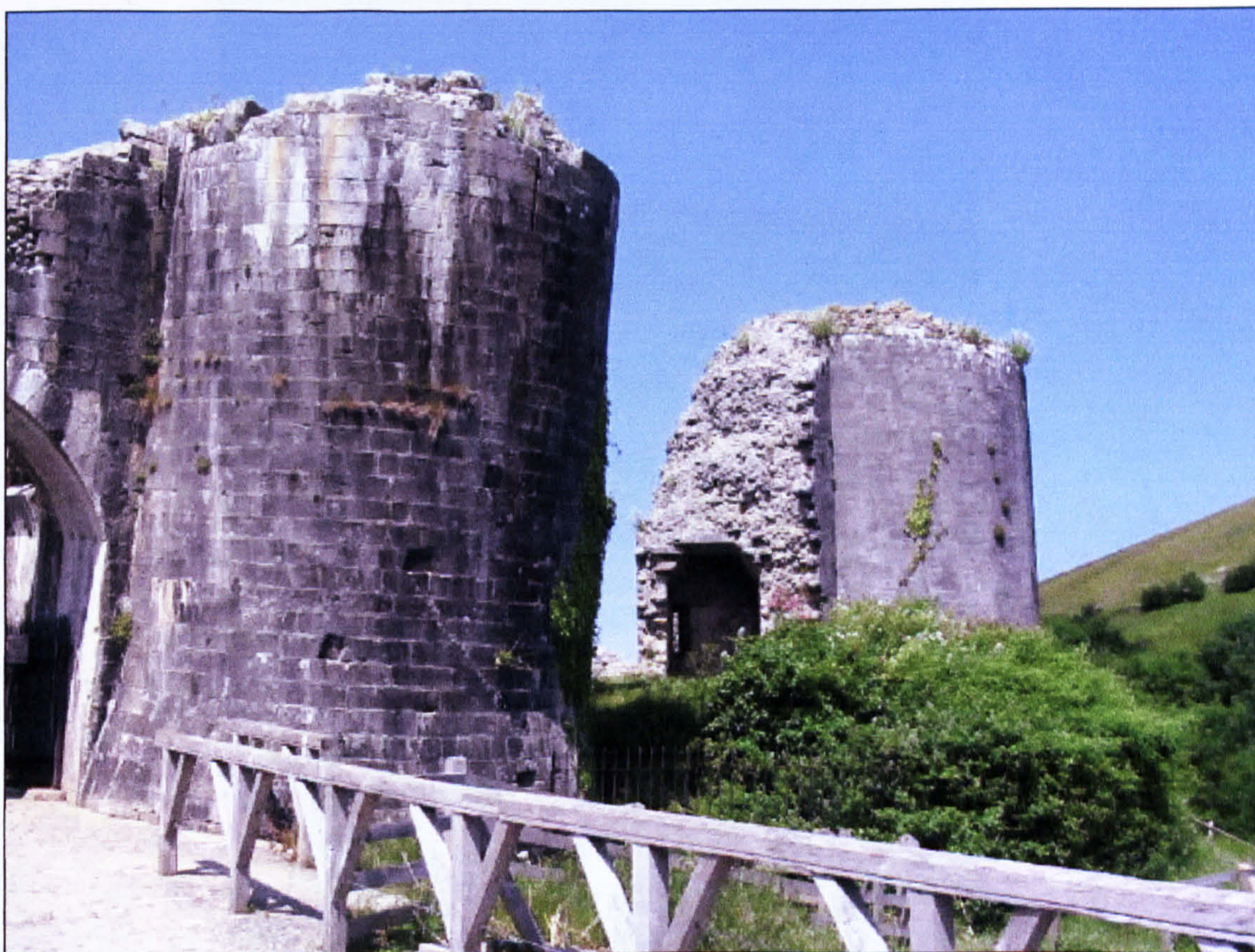
Figure 5.5 The eastern half of the Outer Gatehouse [13] and Horseshoe Tower [12], looking northeast. Vegetation covered debris to right.
