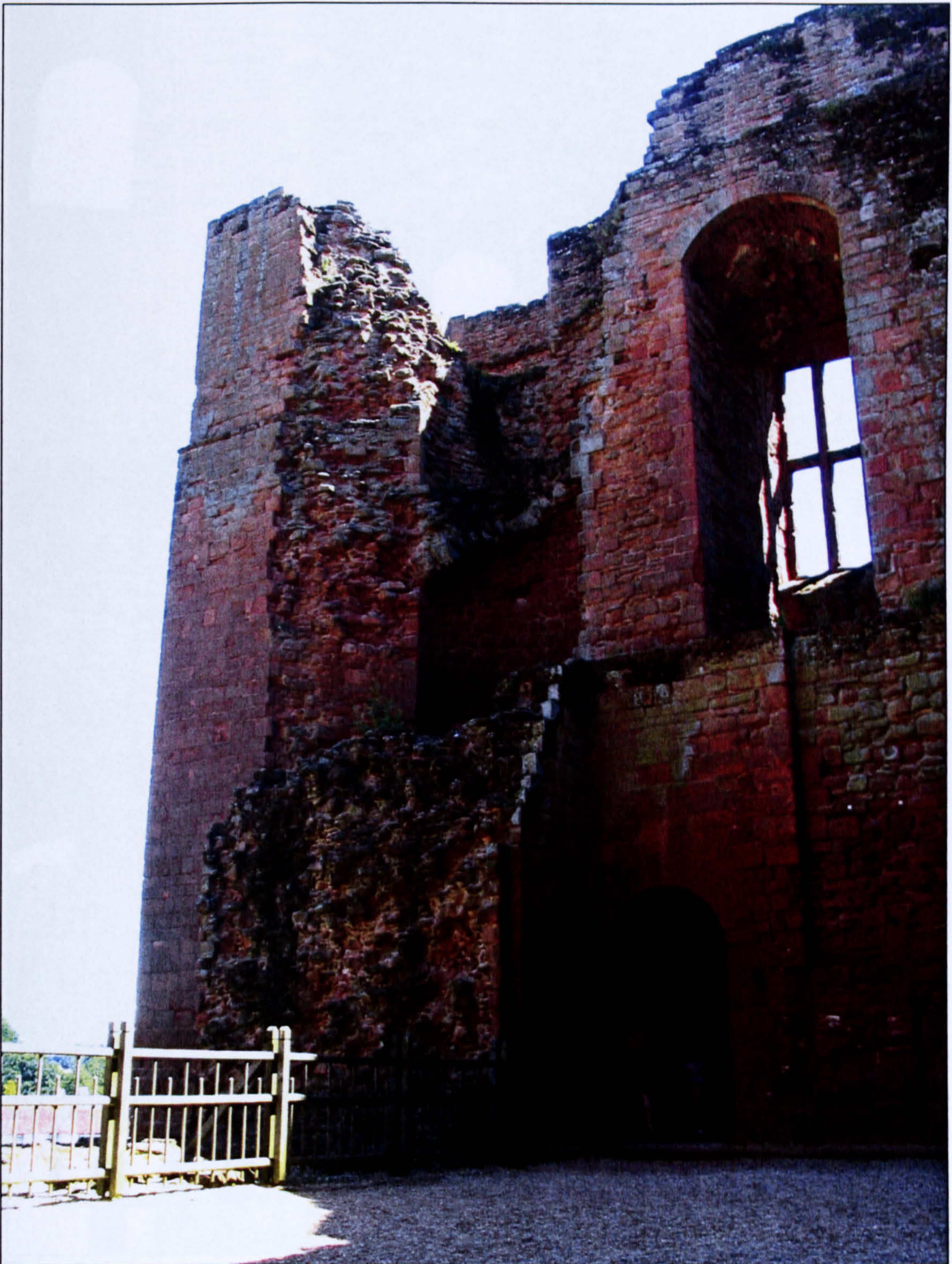
Figure 6.29 The northeast corner of the keep, showing the remnants of an upper floor stairwell.
