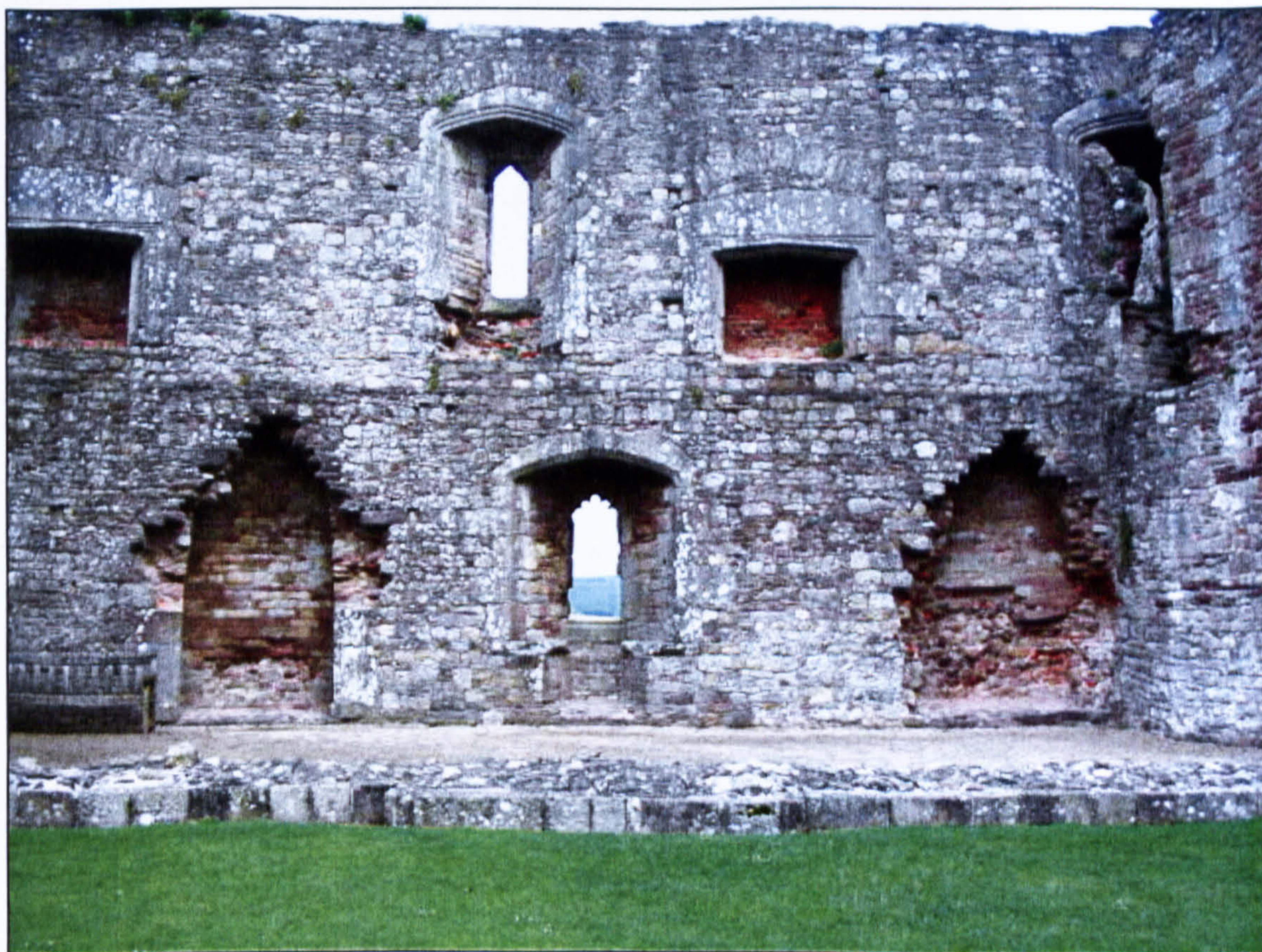
Figure 4.49 Removed fireplaces from the apartments block, Raglan Castle (Wales).
