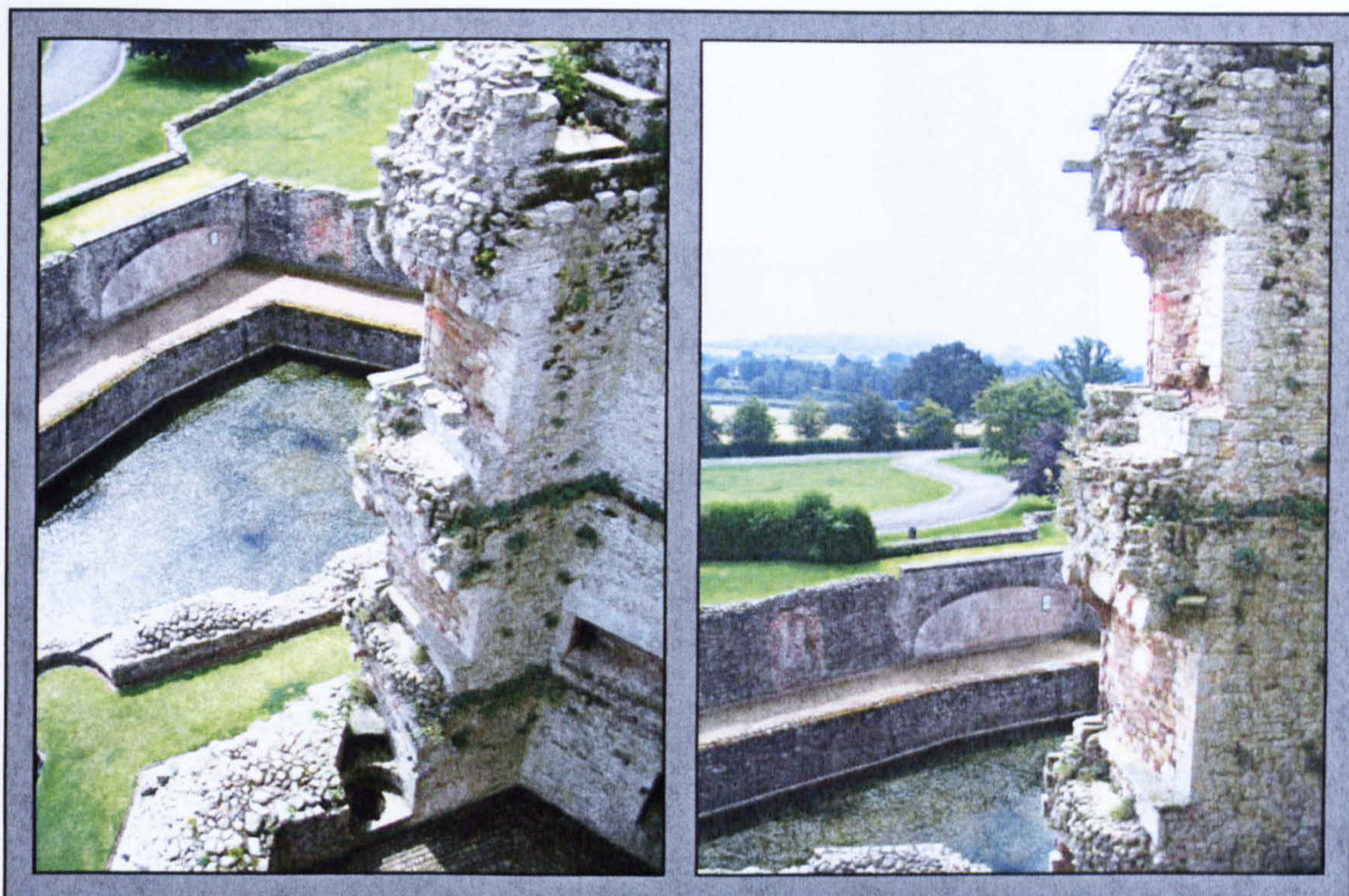
Figure 5.45 Left: The vertical destruction pattern in the southeast wall. Right: A close-up of two of the bisected windows in the wall.
