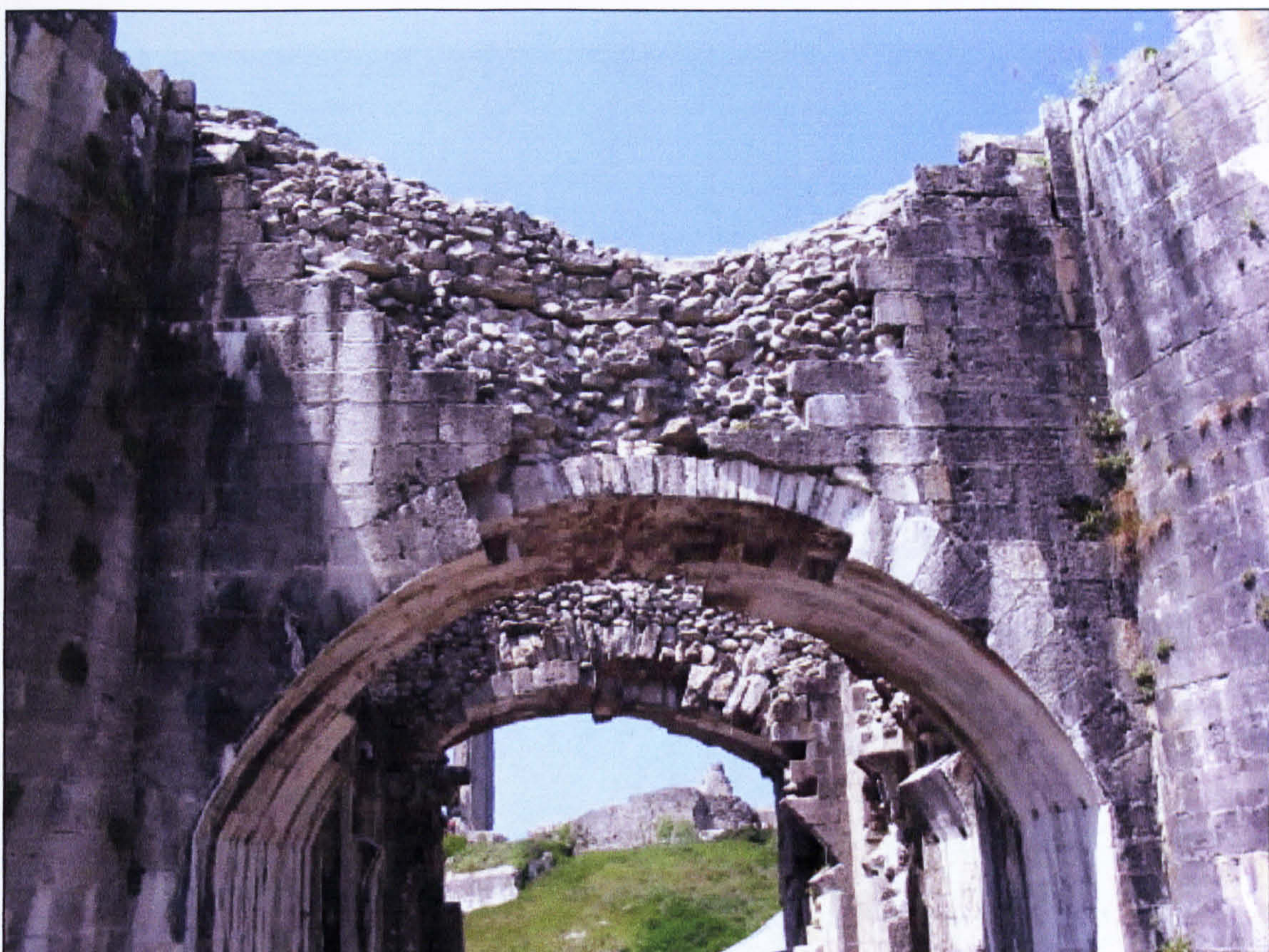
Figure 5.4 Close-up of the exterior archway of the Outer Gatehouse [13], looking north.
