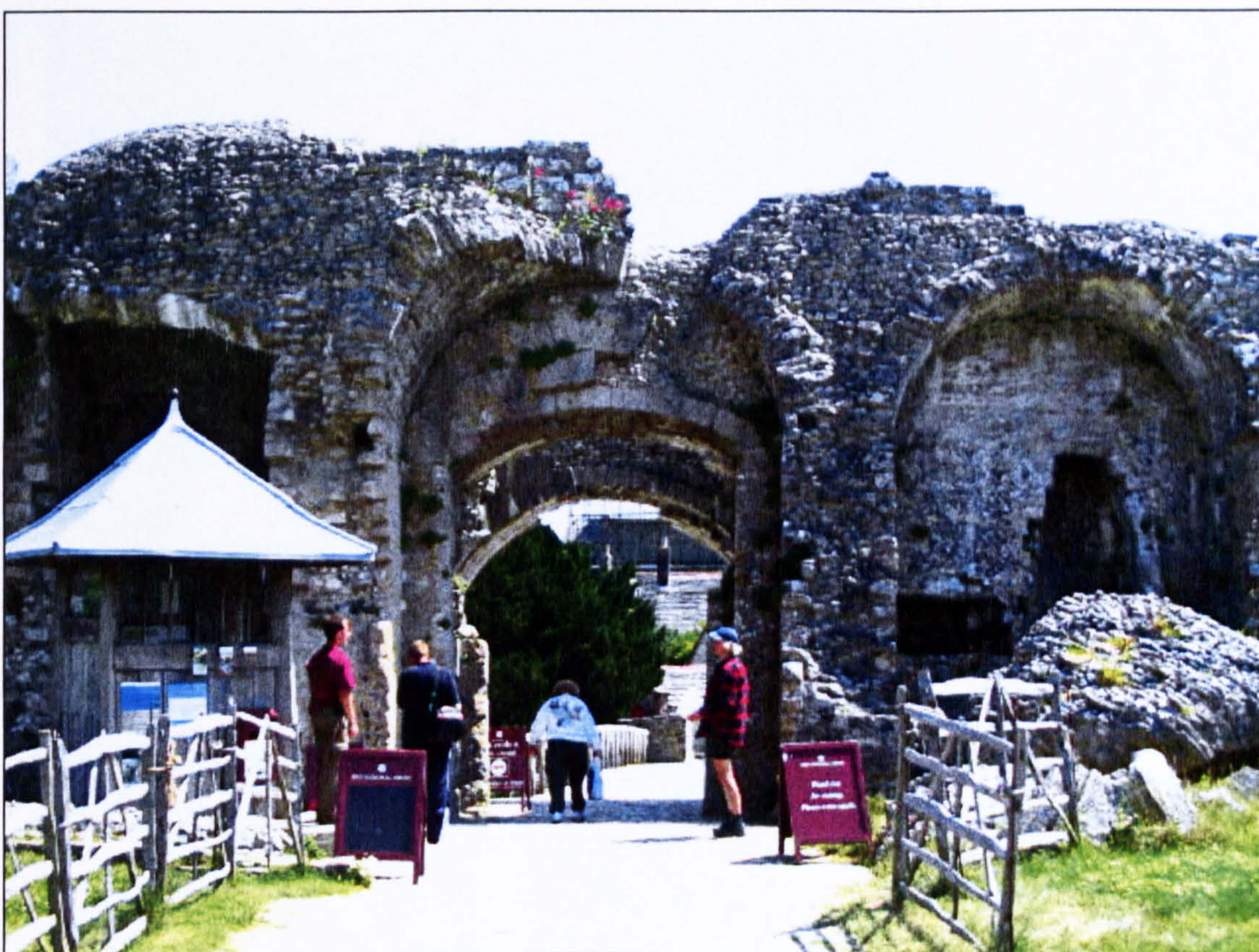
Figure 5.3 Interior of the Outer Gatehouse [13], looking south. Debris to the right.
