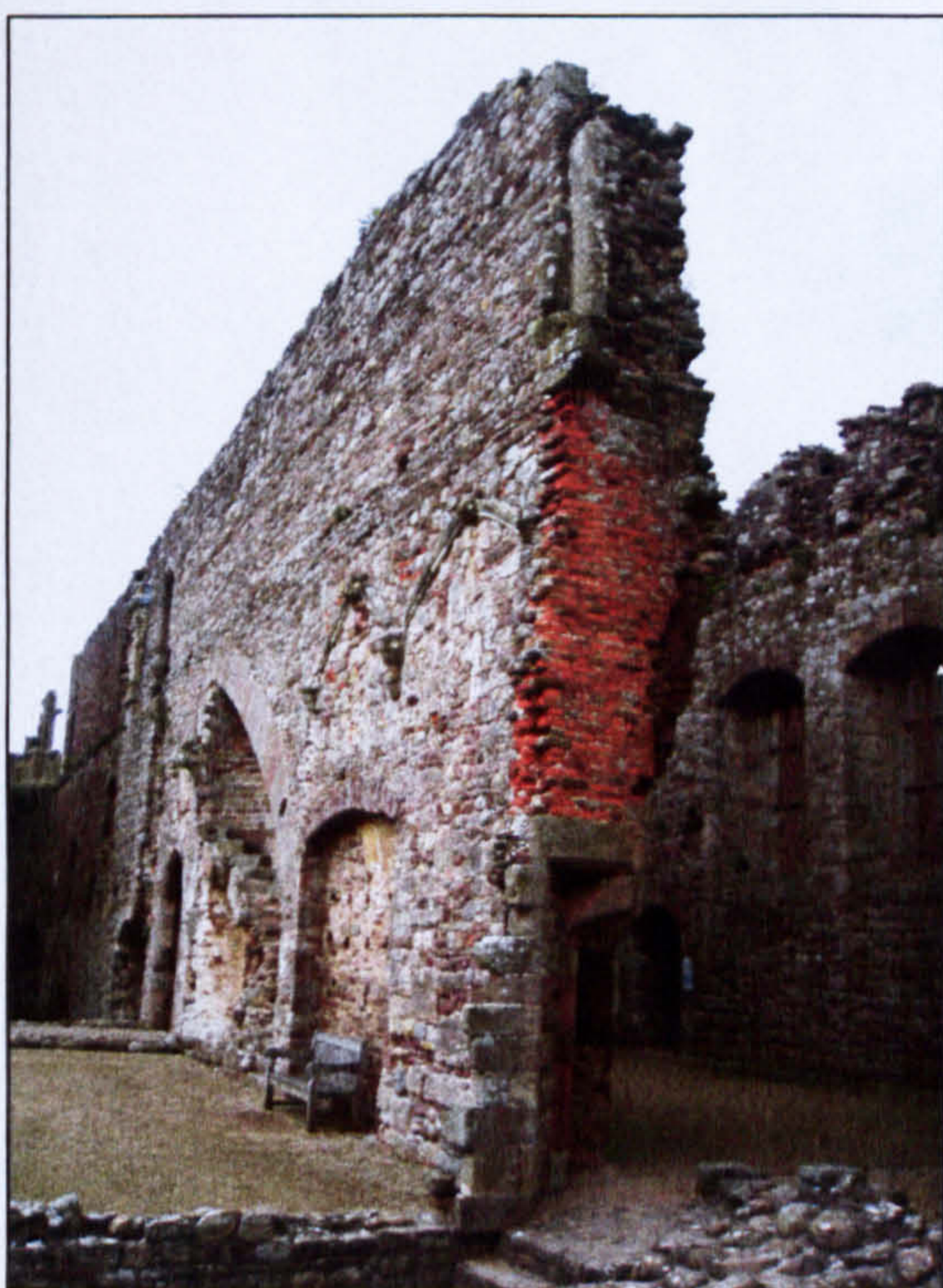
Figure 5.48 Evidence for repair work in the structural remains of Raglan Castle.
