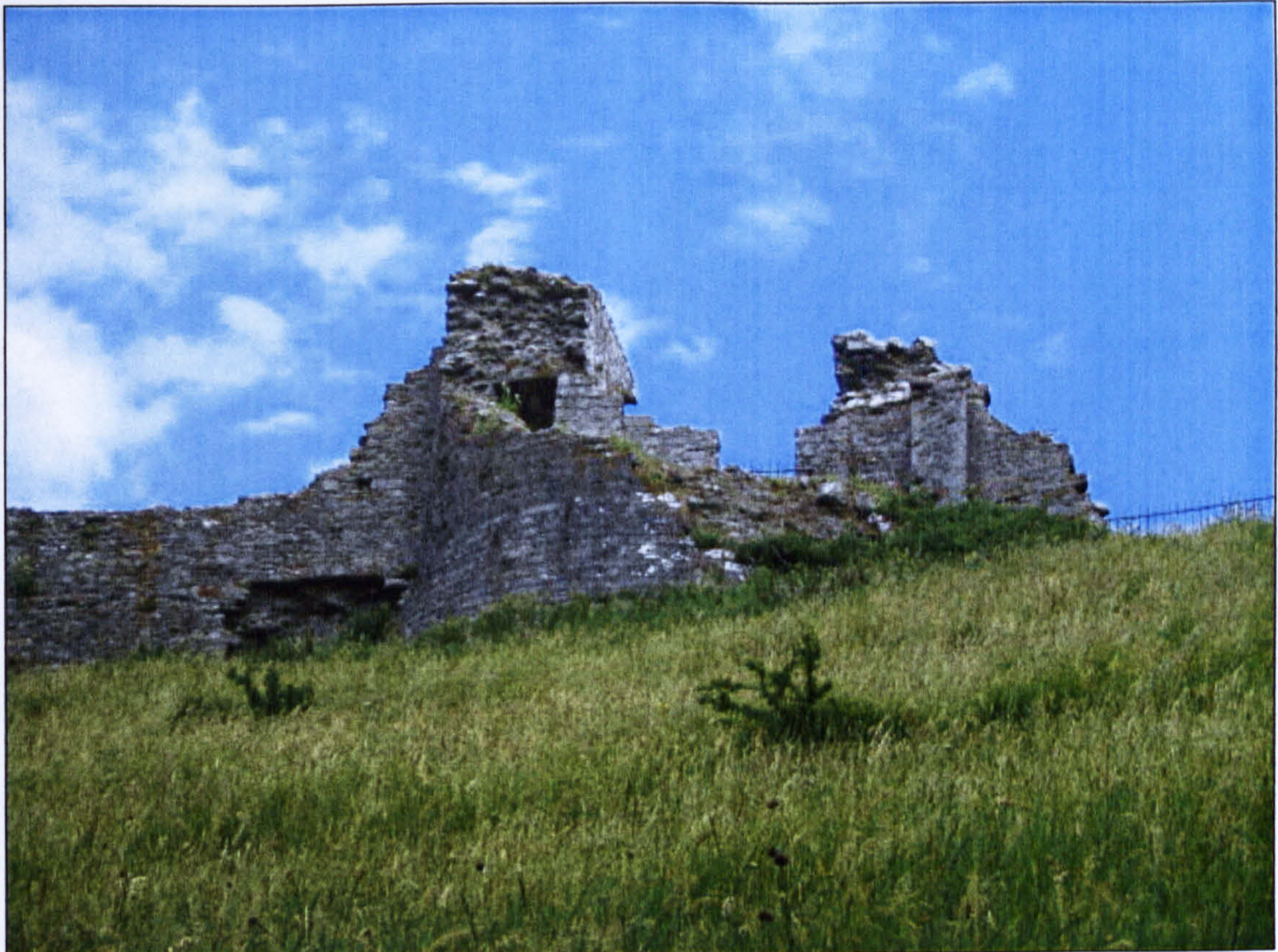
Figure 5.16 The South Tower [6], looking up and northeast.
