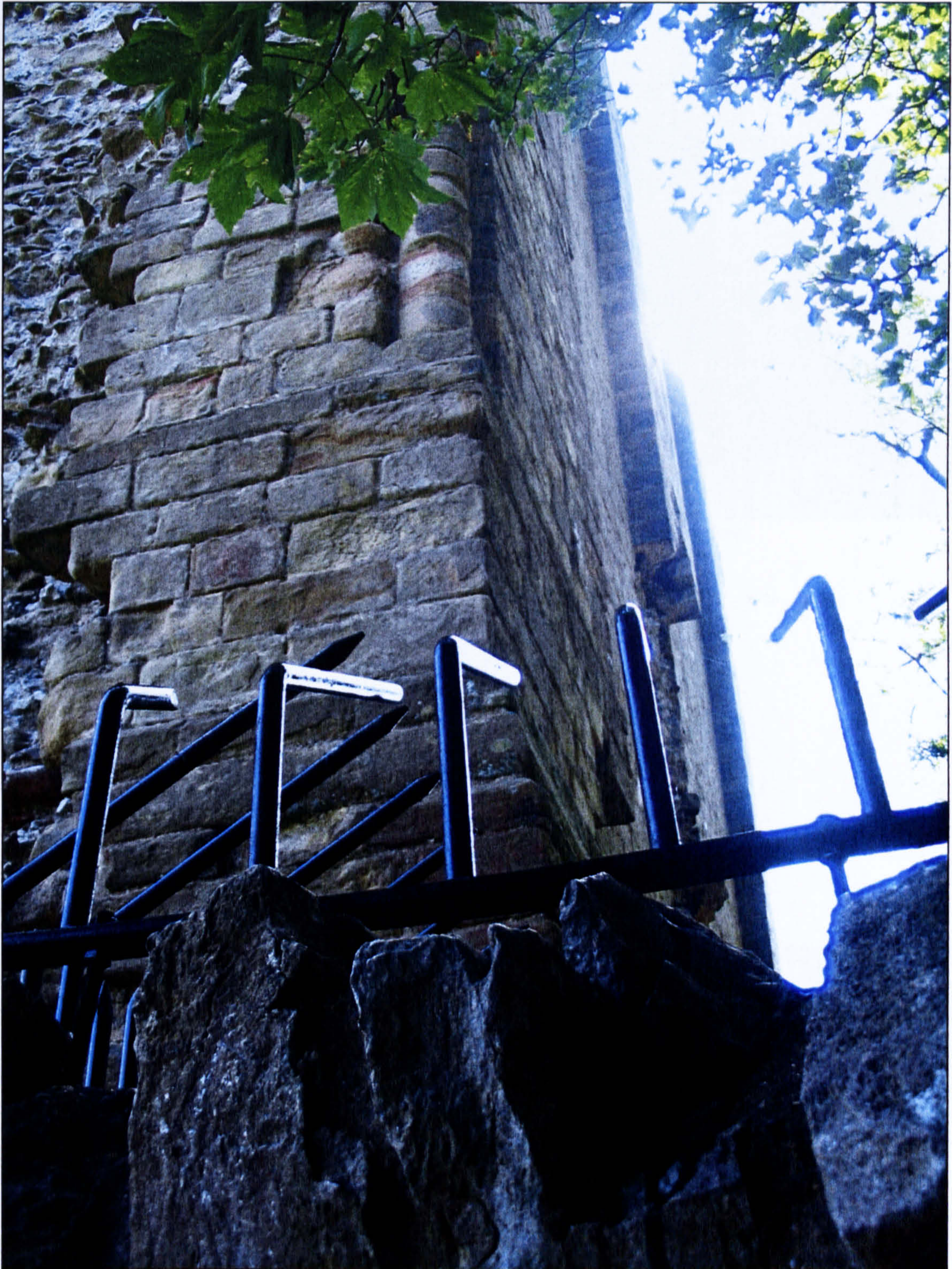
Figure 4.37 The southern corner of Peveril Castle Keep, showing how the inaccessible side of the castle has retained its facing stone.
