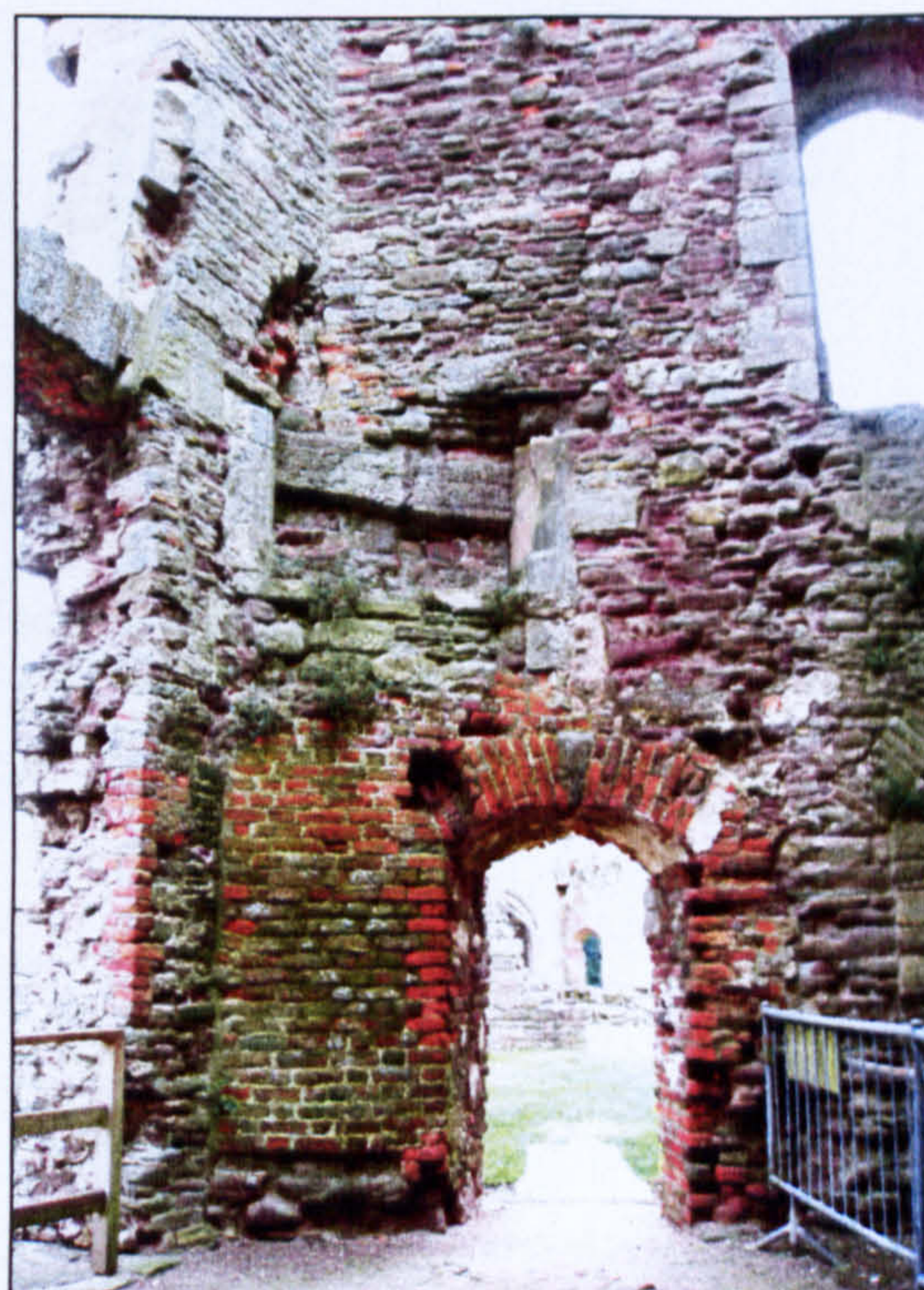
Figure 5.48 Evidence for repair work in the structural remains of Raglan Castle.
