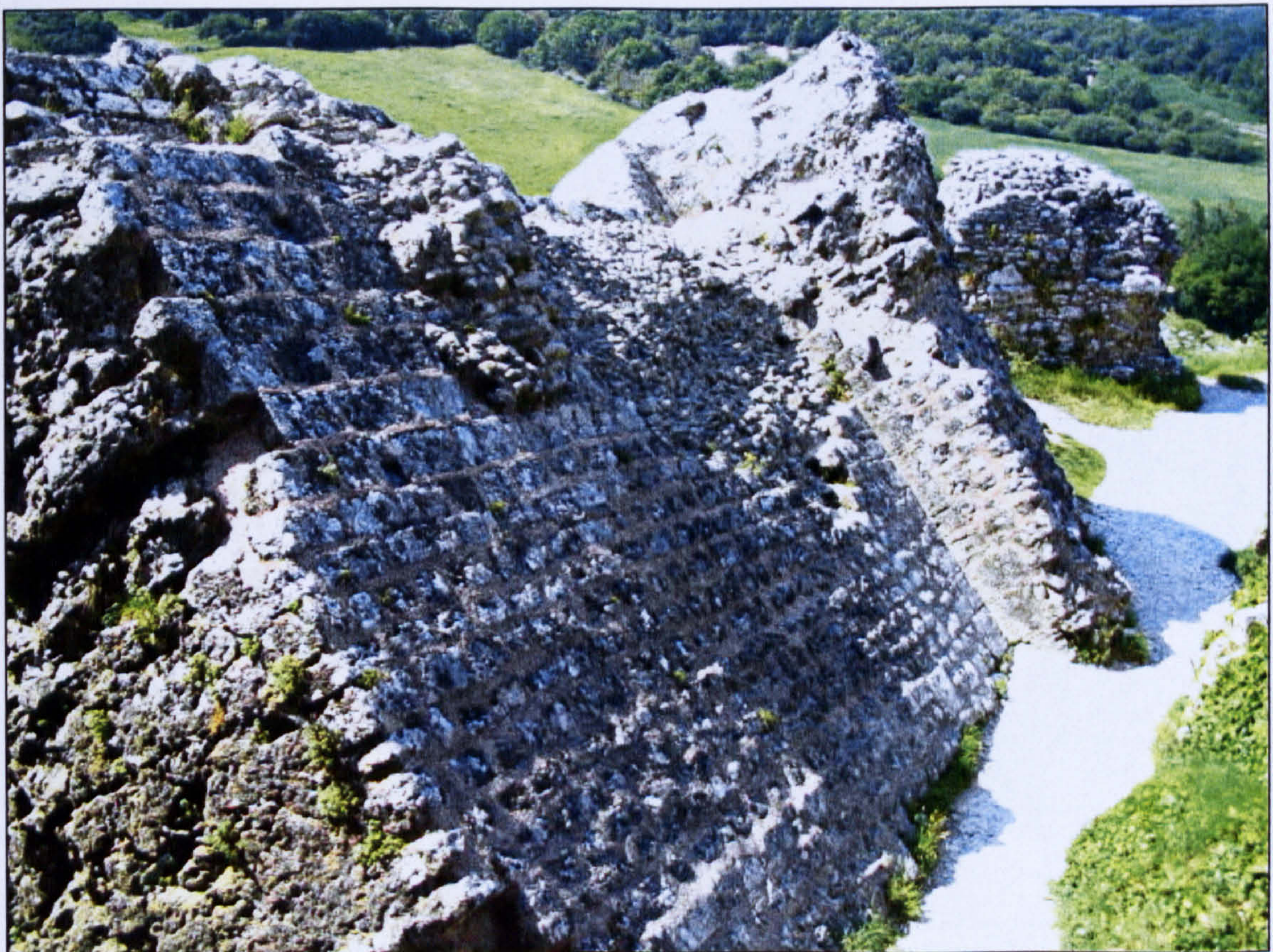
Figure 5.34 Leaning wall, west approach (View 3).
