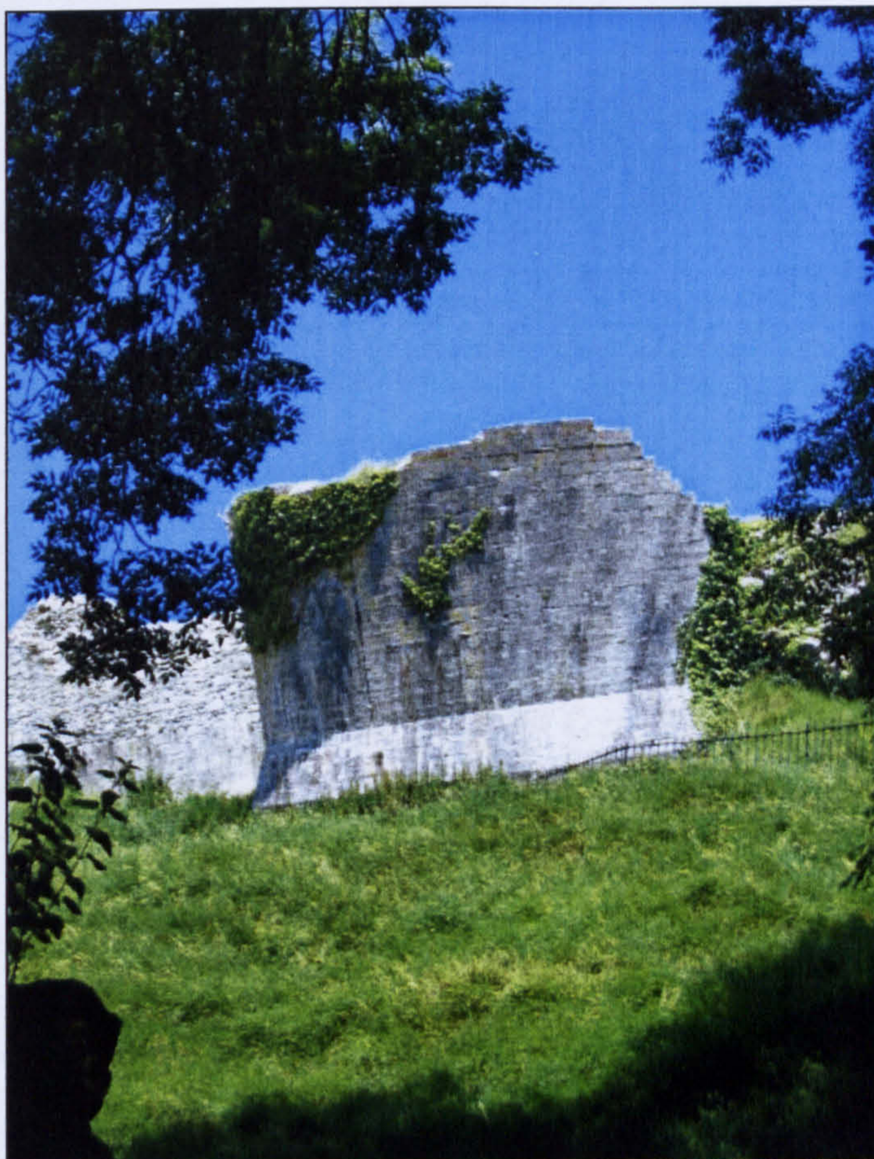
Figure 5.12 The Second Tower [2], looking up and east.
