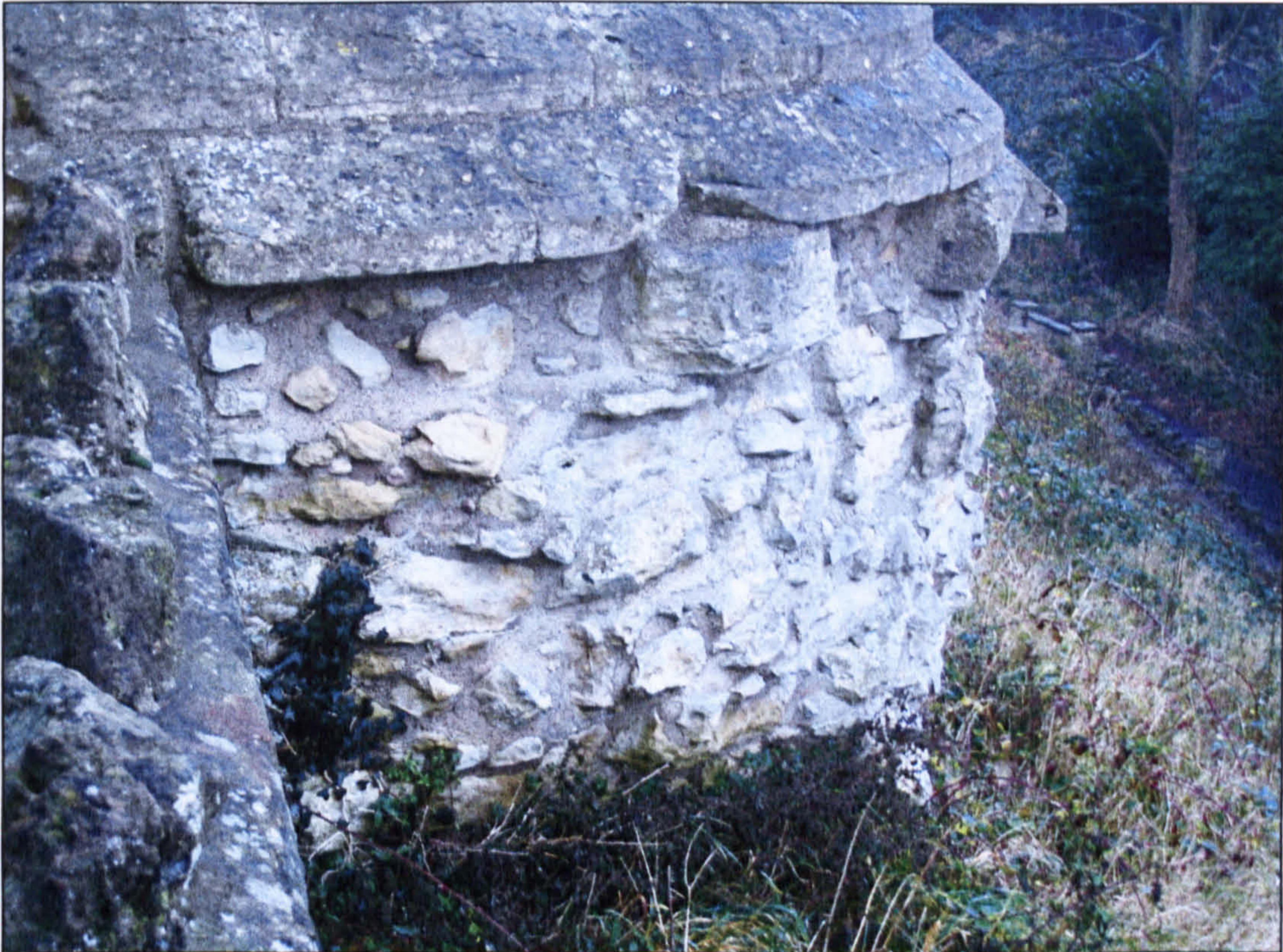
Figure 4.20 Plinth of T1, looking east.
