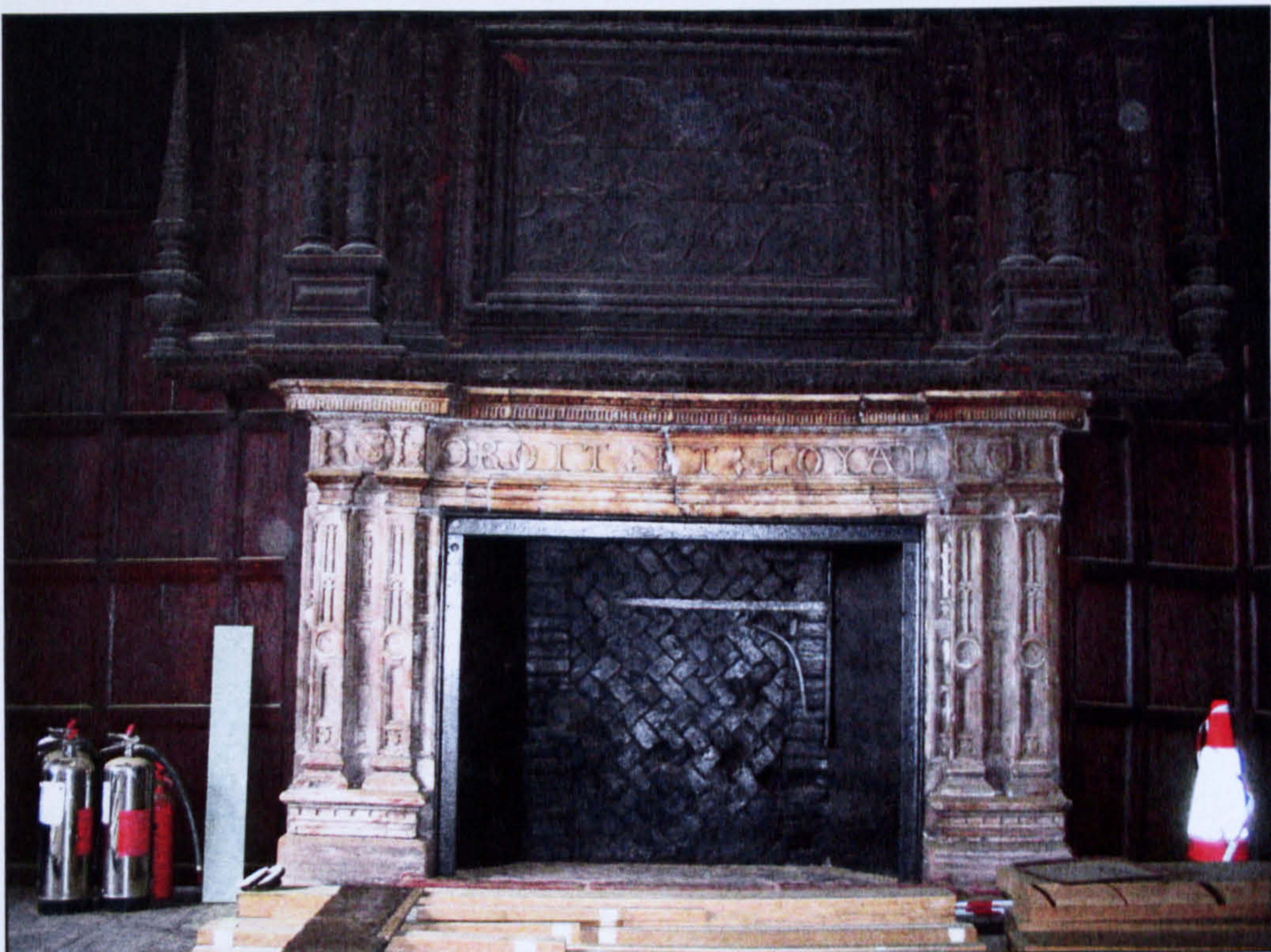
Figure 6.14 Leicester's alabaster fireplace, and above, oak panelling and fittings, all of which were removed from other buildings.
