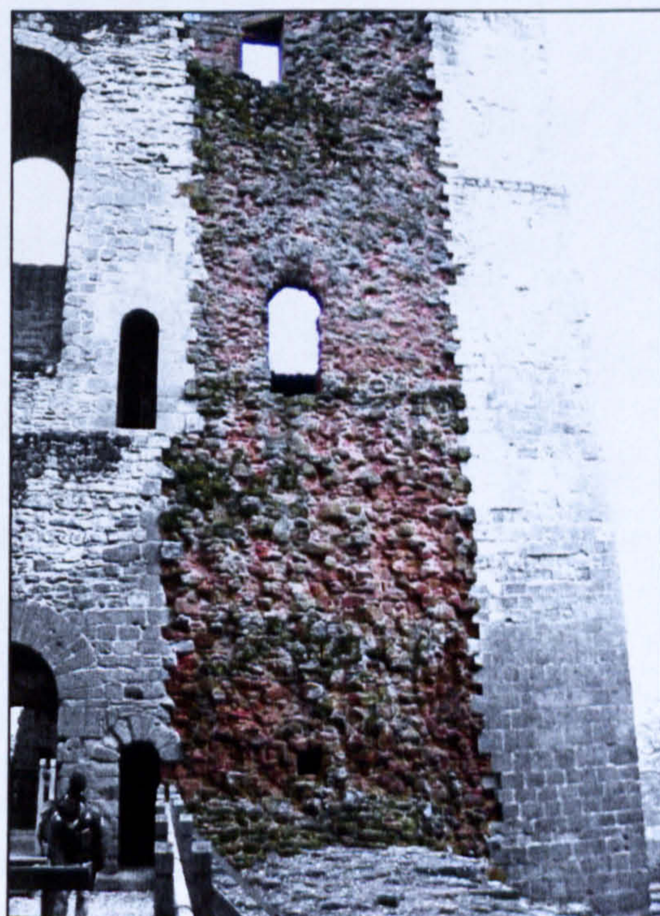
Figure 6.28 Left: The linear pattern of the exposed rubble core, northeast corner. Right: The linear pattern of the exposed rubble core, northwest corner.
