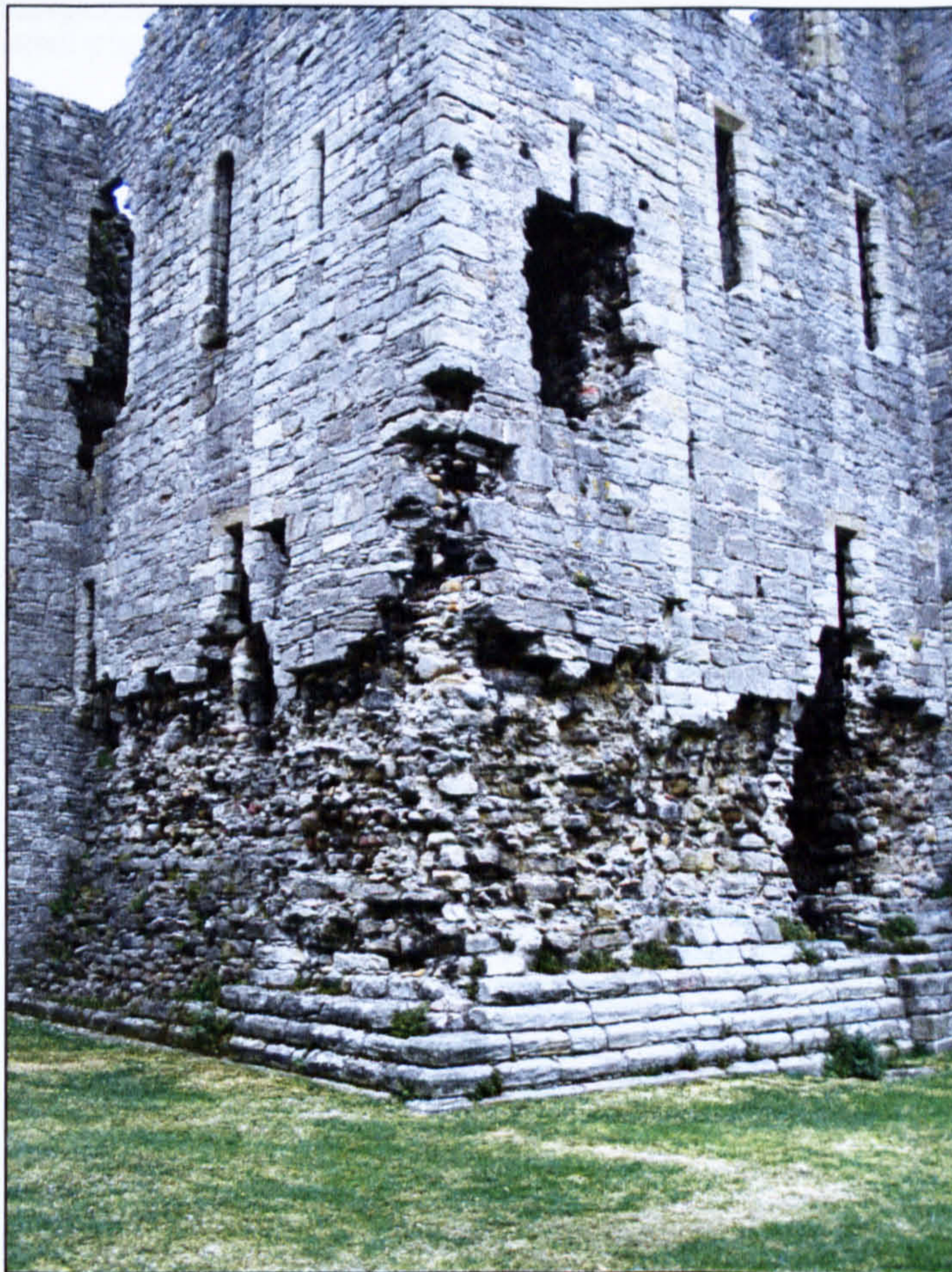
Figure 4.41 Secondary damage pattern in the form of removed facing stone at Middleham Castle (Yorkshire).
