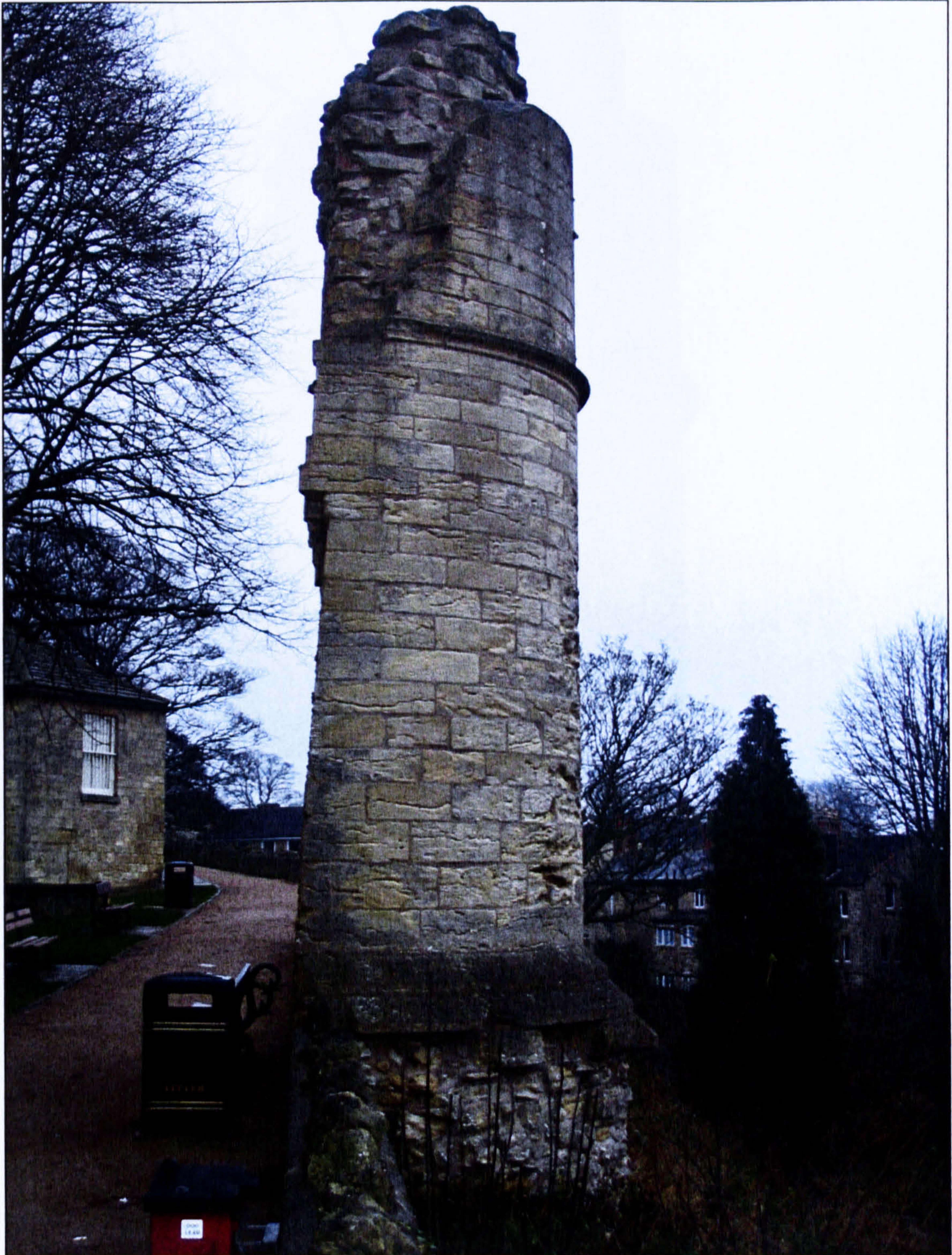
Figure 4.17 Side view of T1, looking east.
