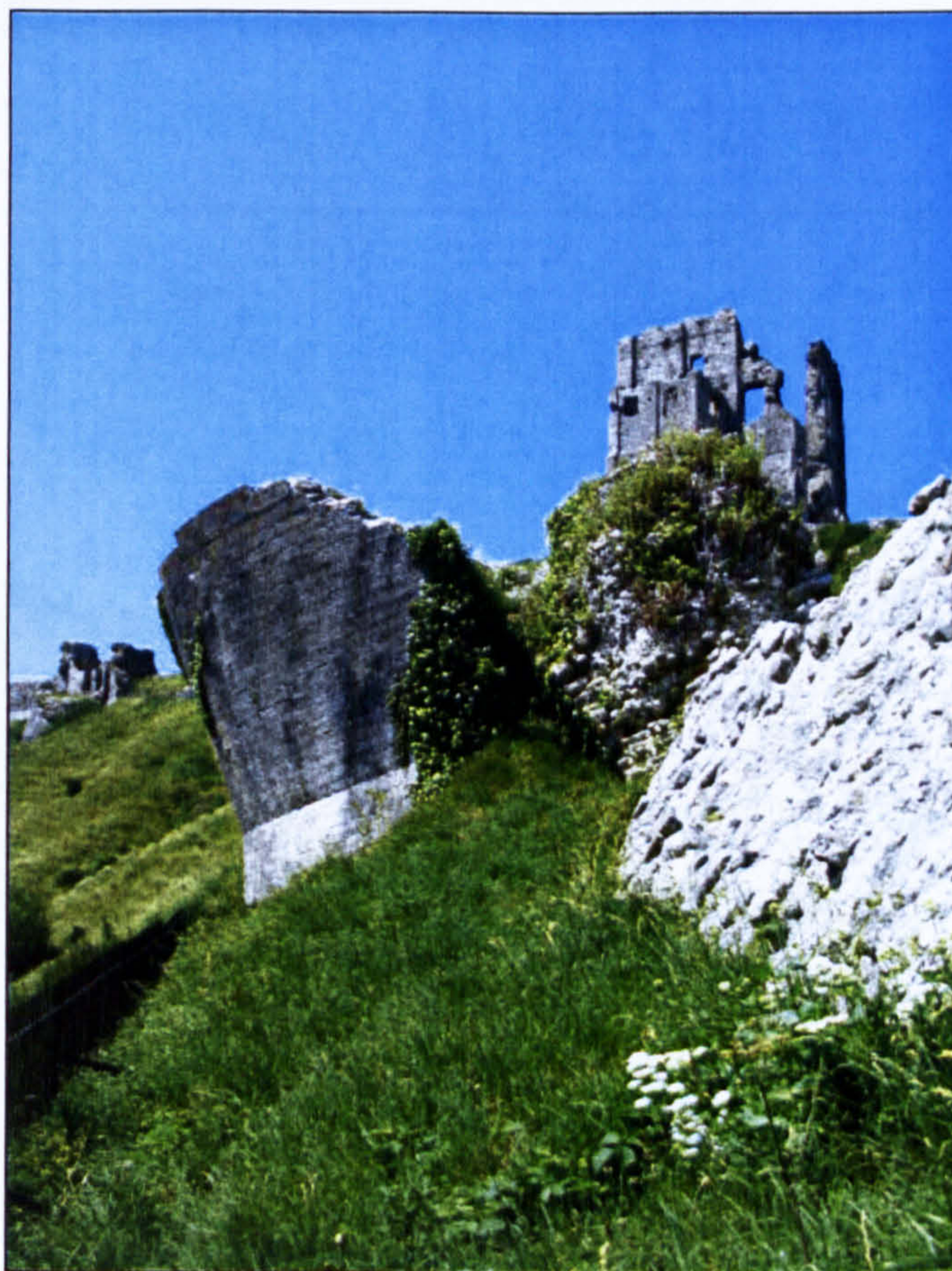
Figure 5.11 The Second Tower [2] and curtain wall to right, looking north (view 2).
