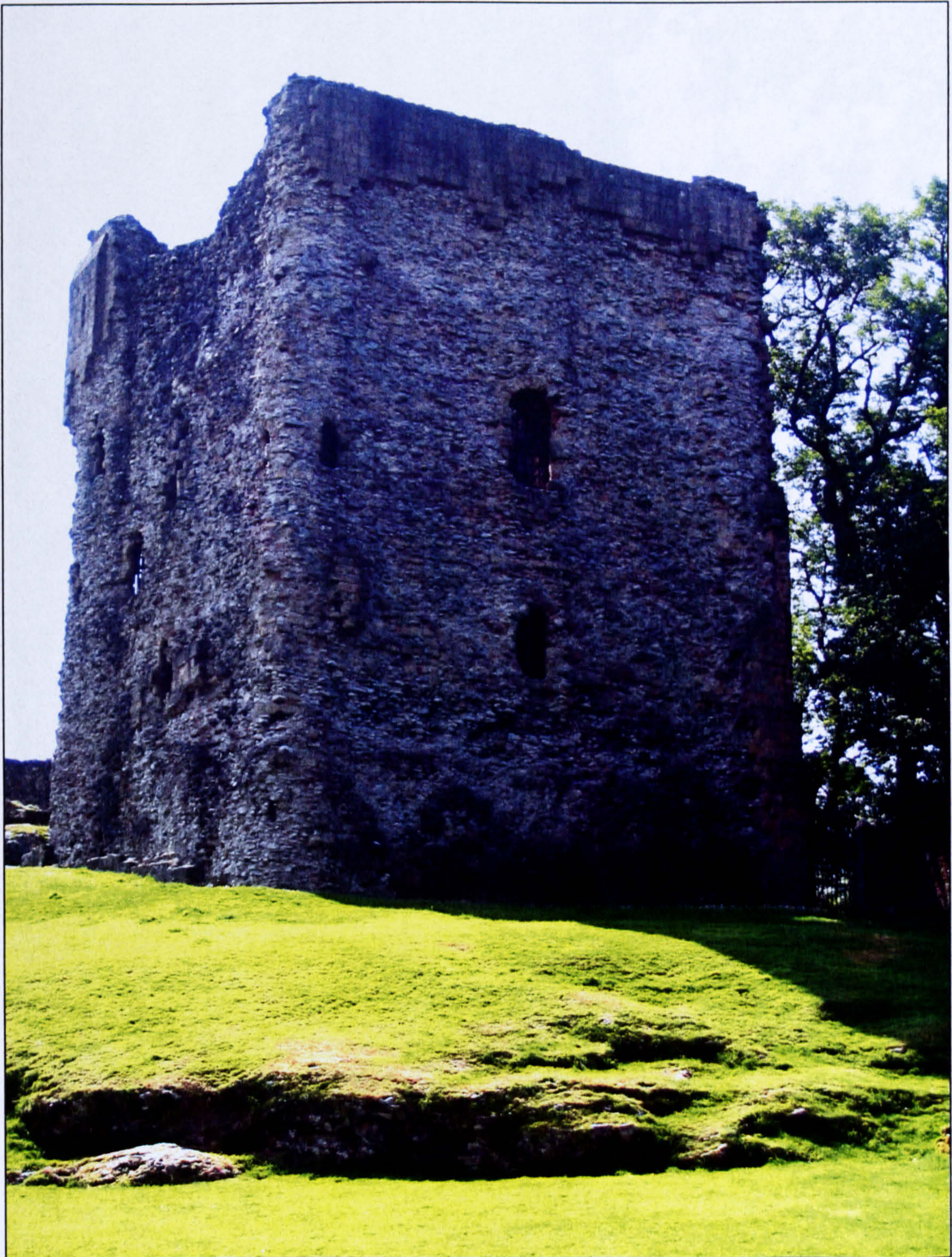
Figure 4.36 Peveril Castle Keep, looking east, showing the scale of secondary damage.
