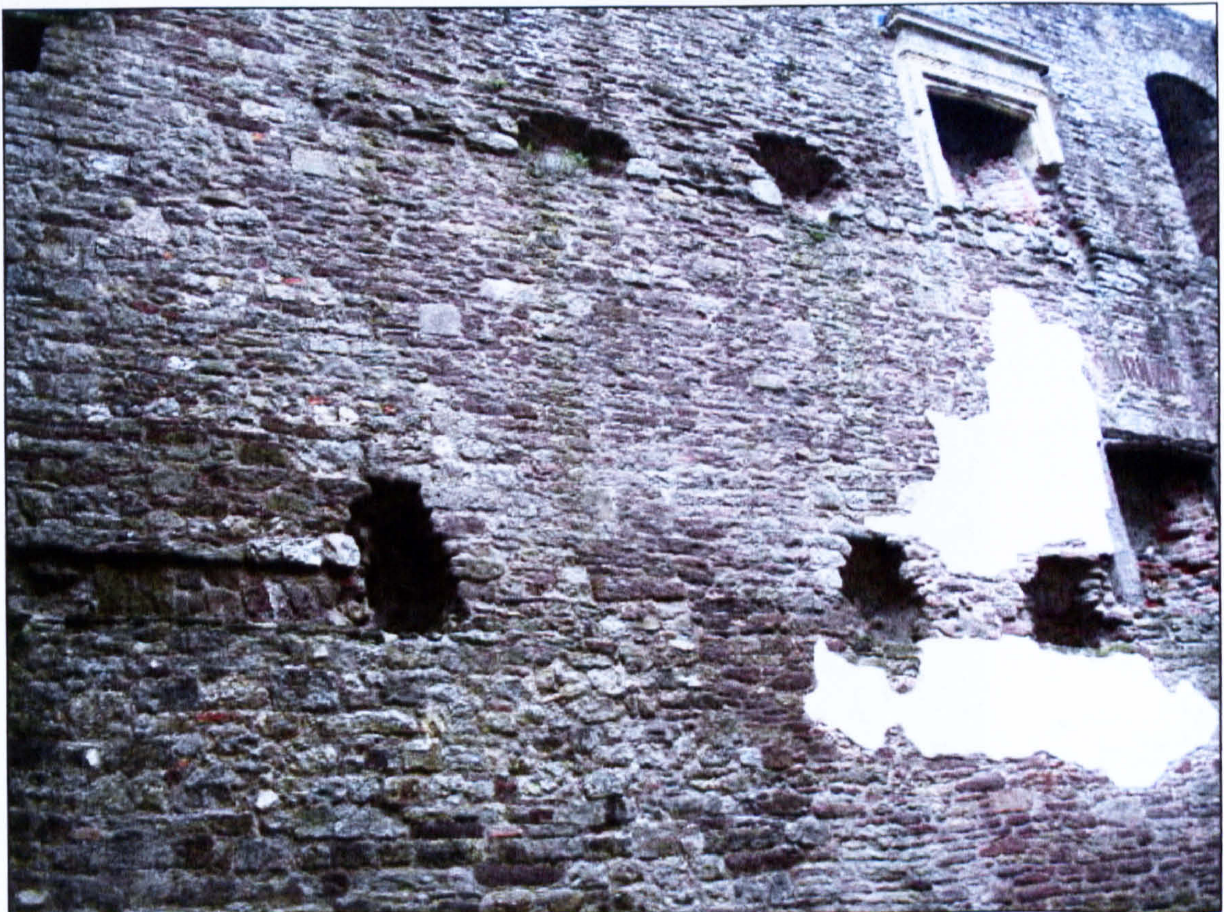
Figure 4.45 Joist hole placements in the buttery, Raglan Castle (Wales) (view 2).
