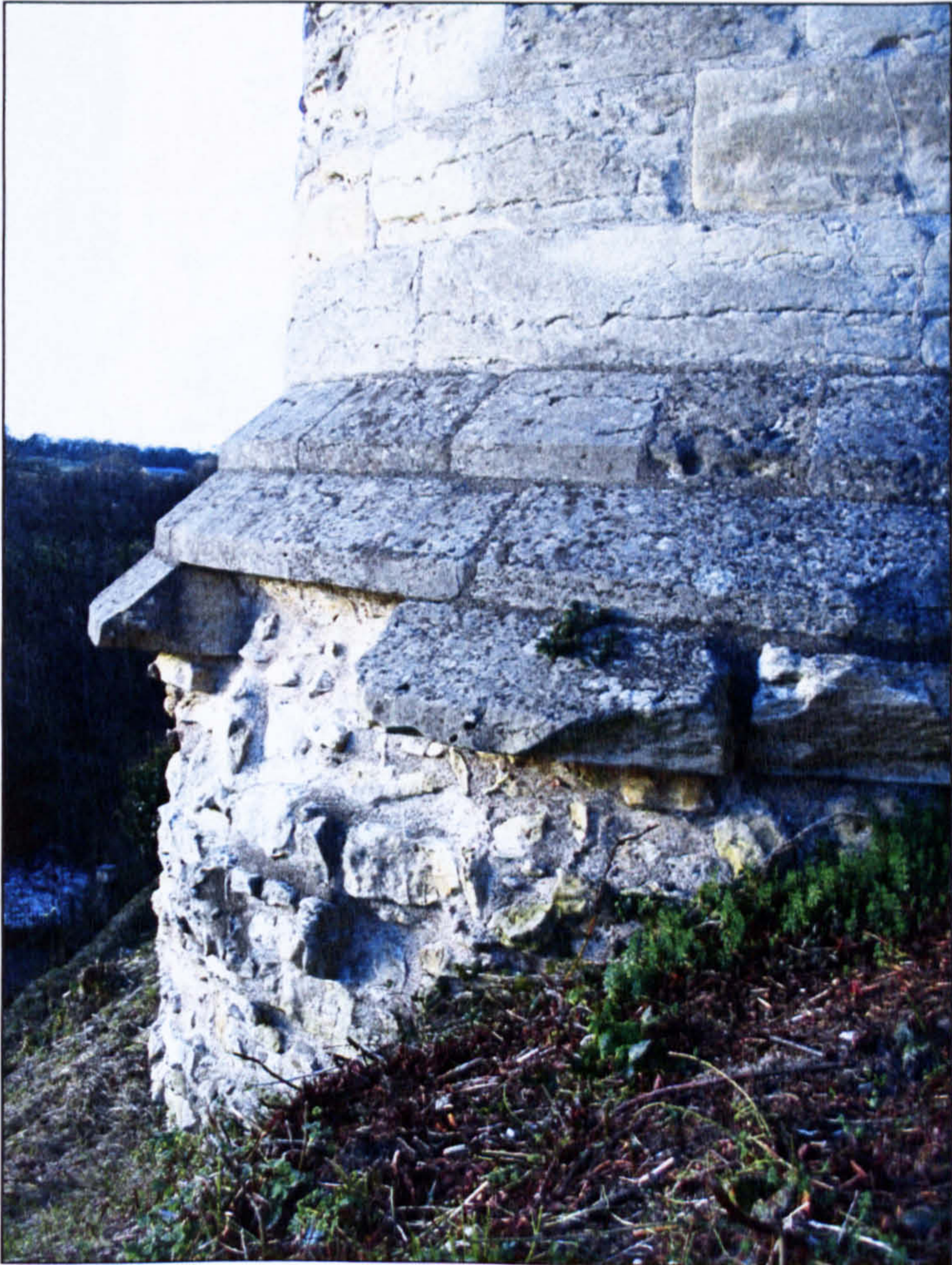
Figure 4.21 Plinth of T1, looking west.
