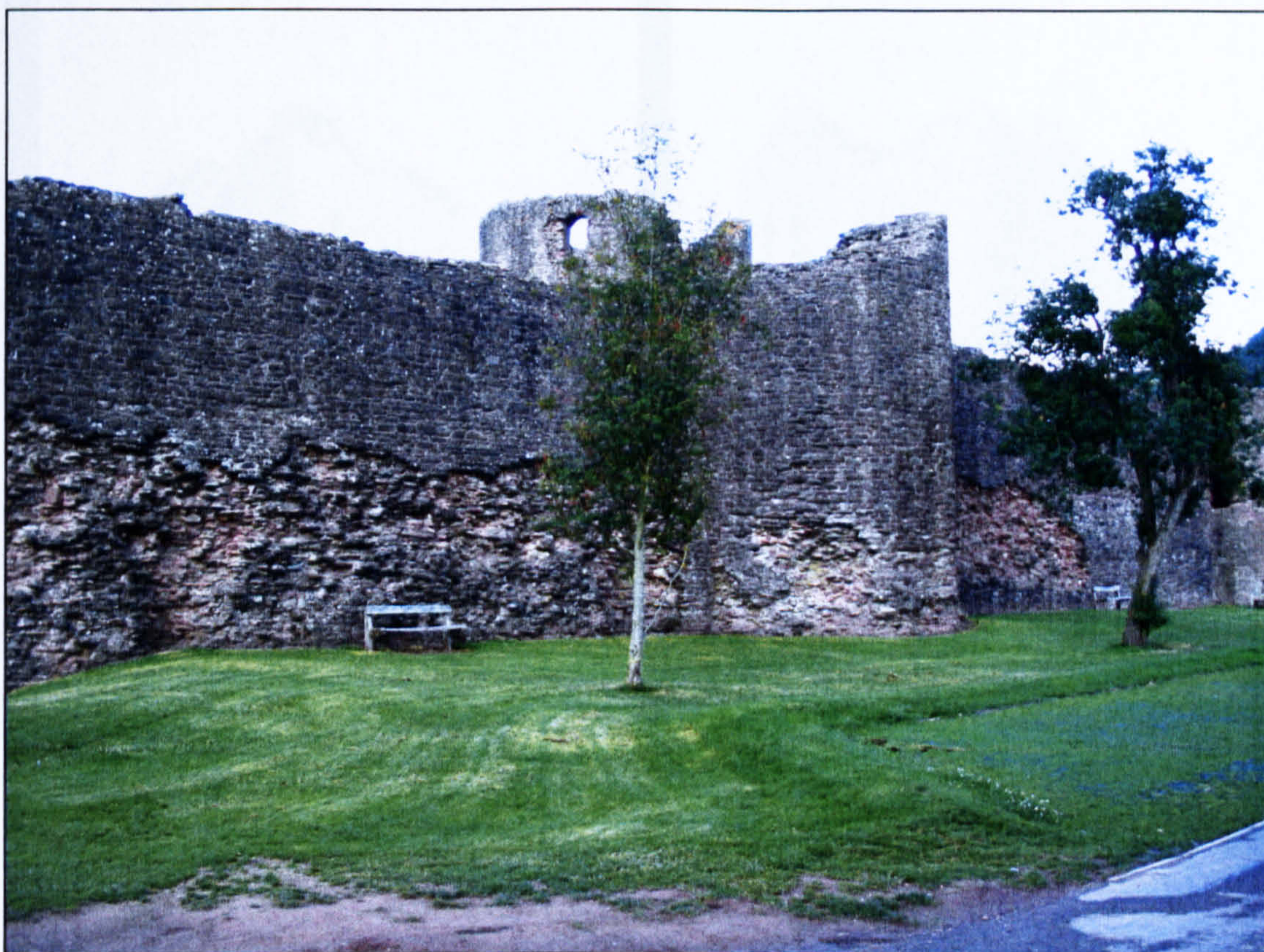
Figure 3.14 External wall of Skenrith Castle (Wales) showing robbed out lower half.
