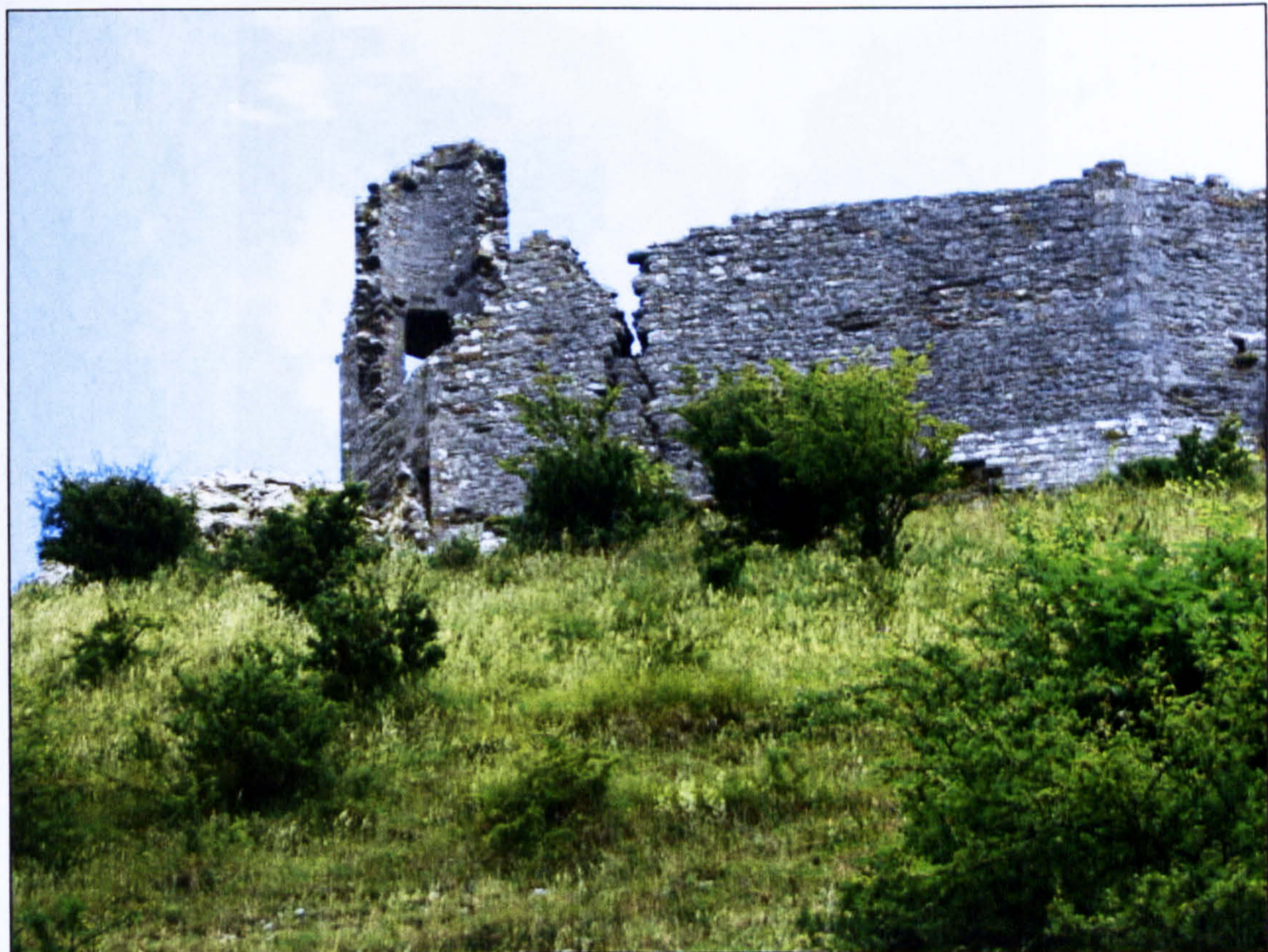
Figure 5.17 The Butavant Tower [7], looking up and northeast.
