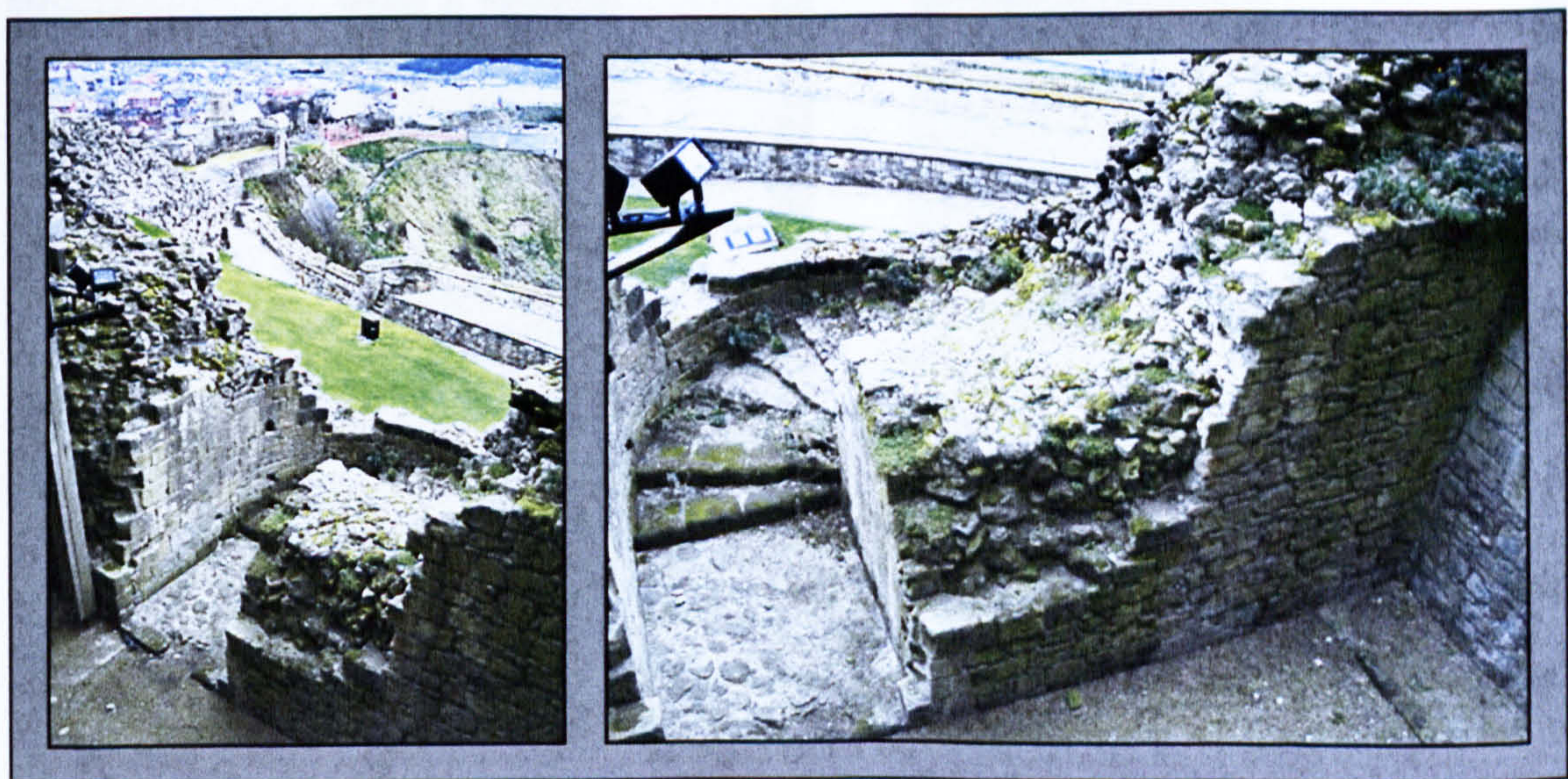
Figure 5.68 Left : Stairwell at Scarborough Castle Keep, looking southwest. Right : Scarborough Castle Keep looking northwest.
