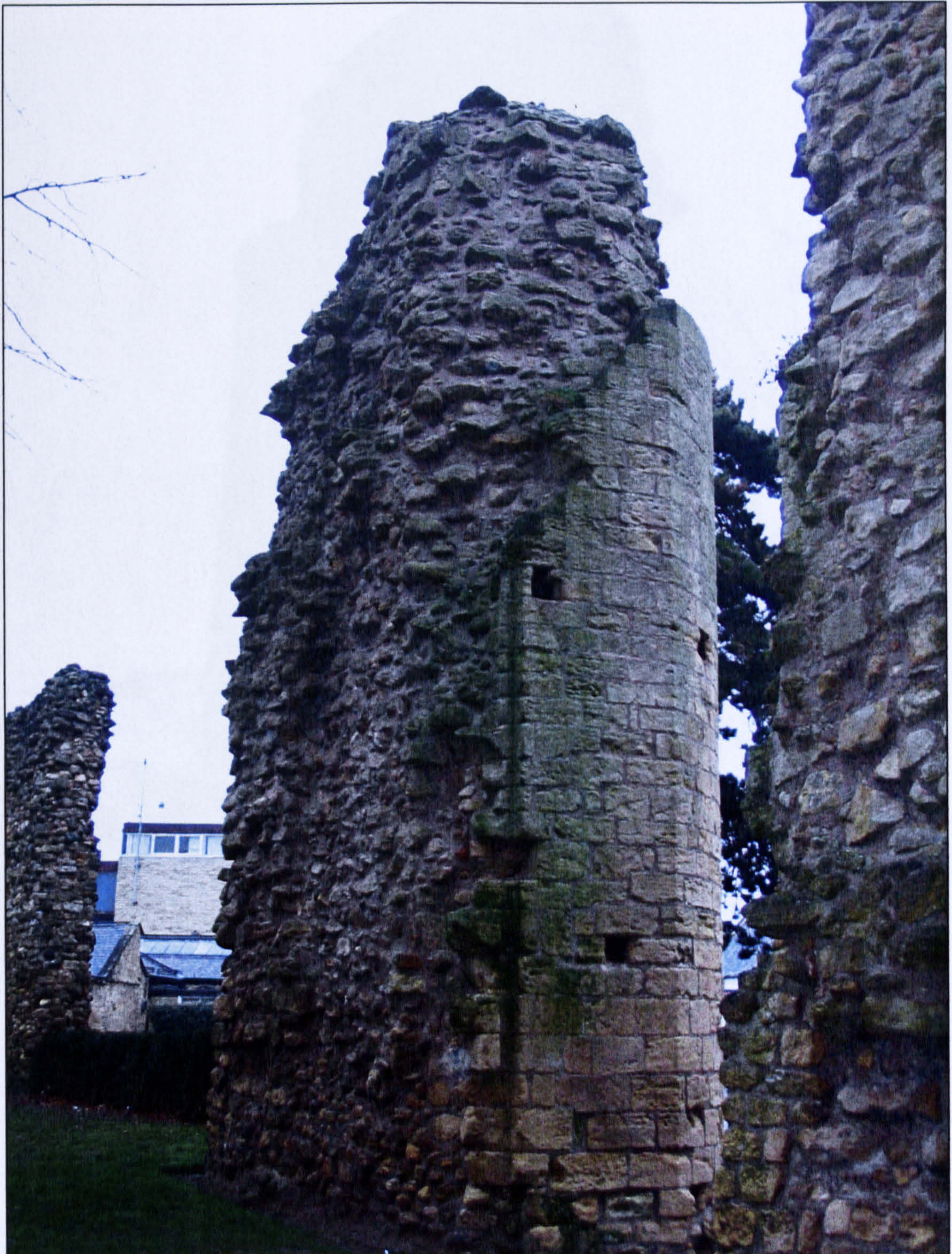
Figure 4.12 G2 with portcullis groove and putlog holes.
