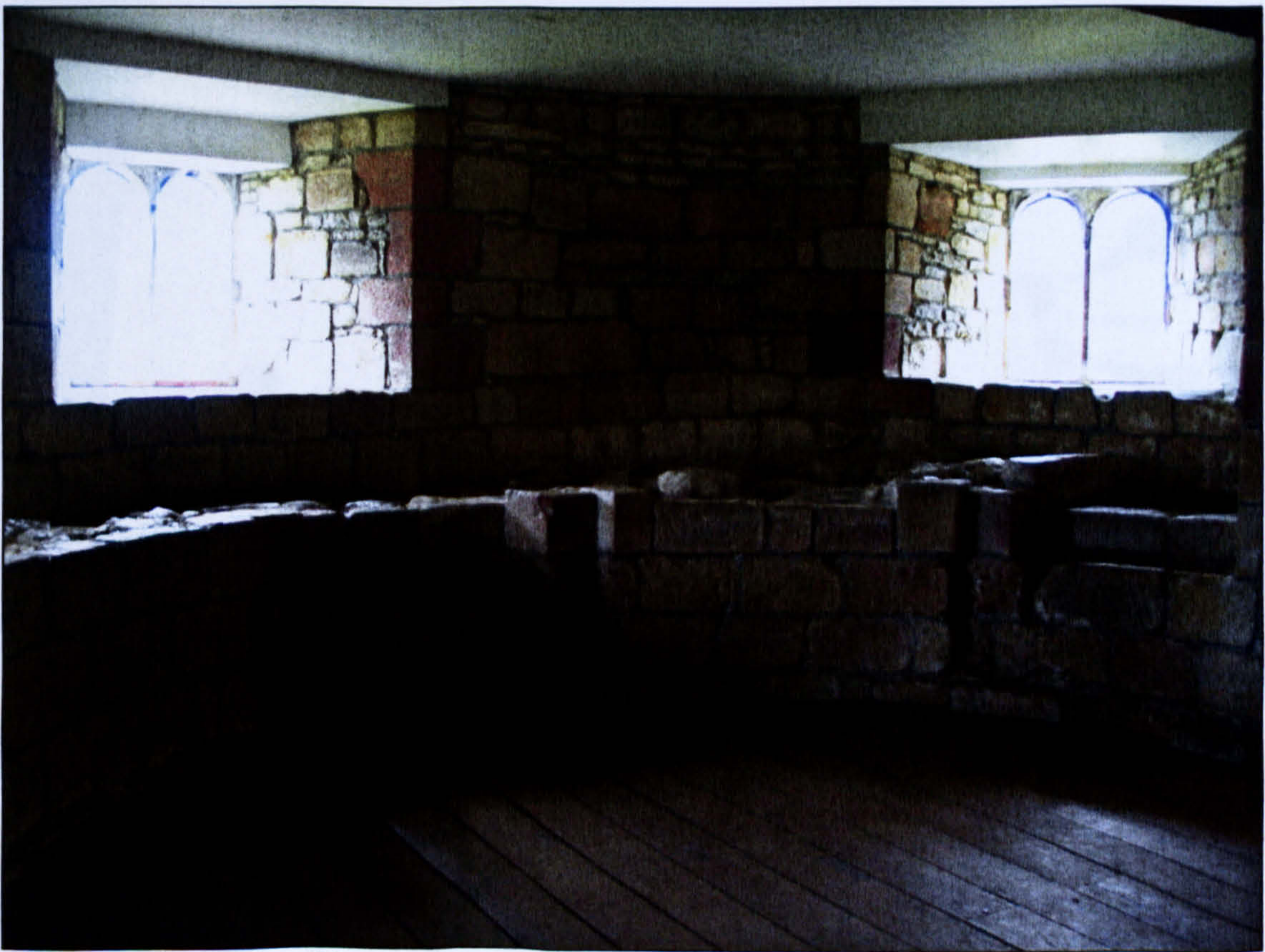
Figure 4.4 The interior of the watchtower, middle floor, Skipton Castle. Lower half shows the original medieval wall thickness, while the upper half is Lady Anne Clifford's rebuild.
