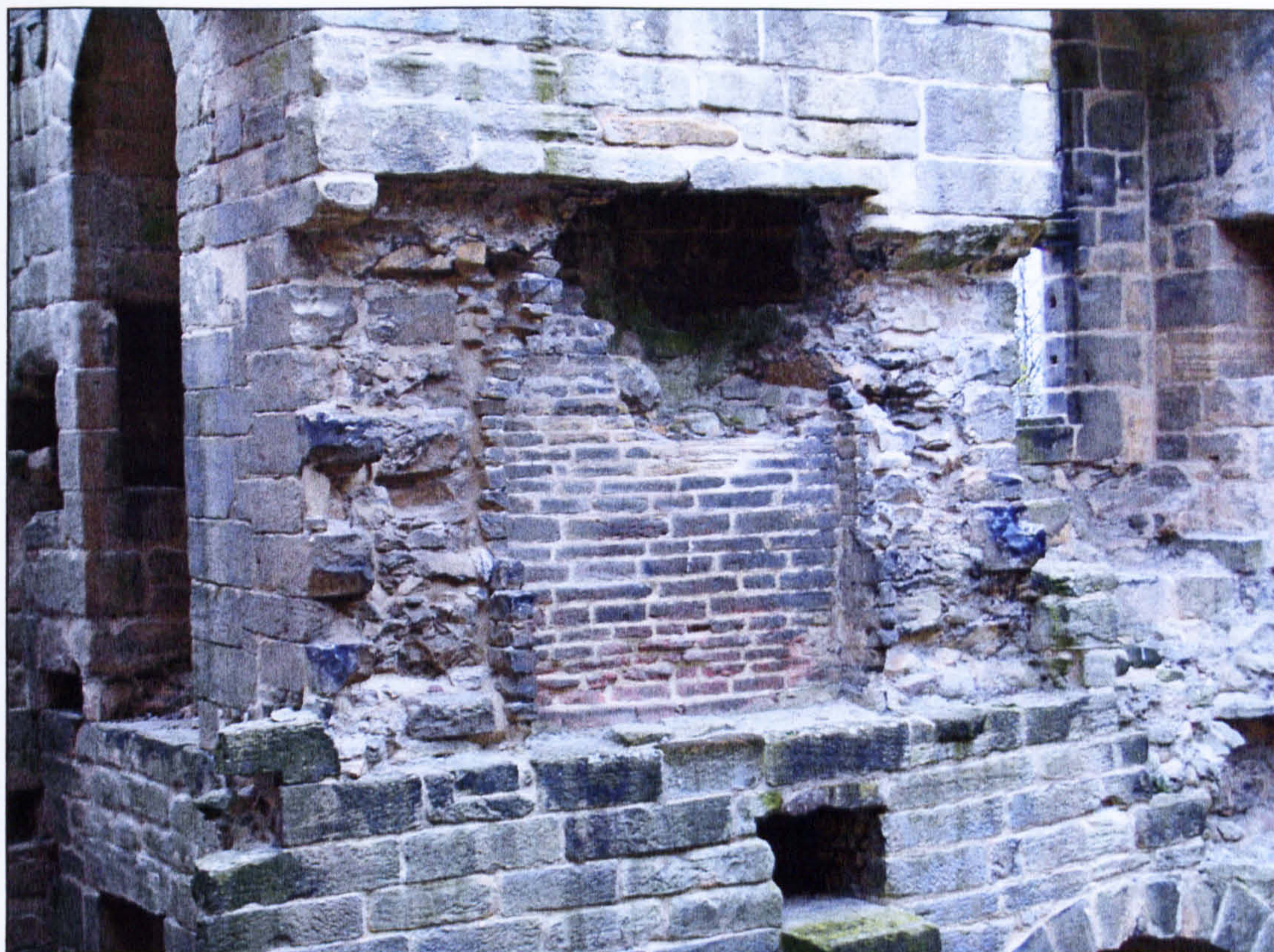
Figure 4.50 Removed fireplace from the Lower Hall, Harewood Castle (Yorkshire).
