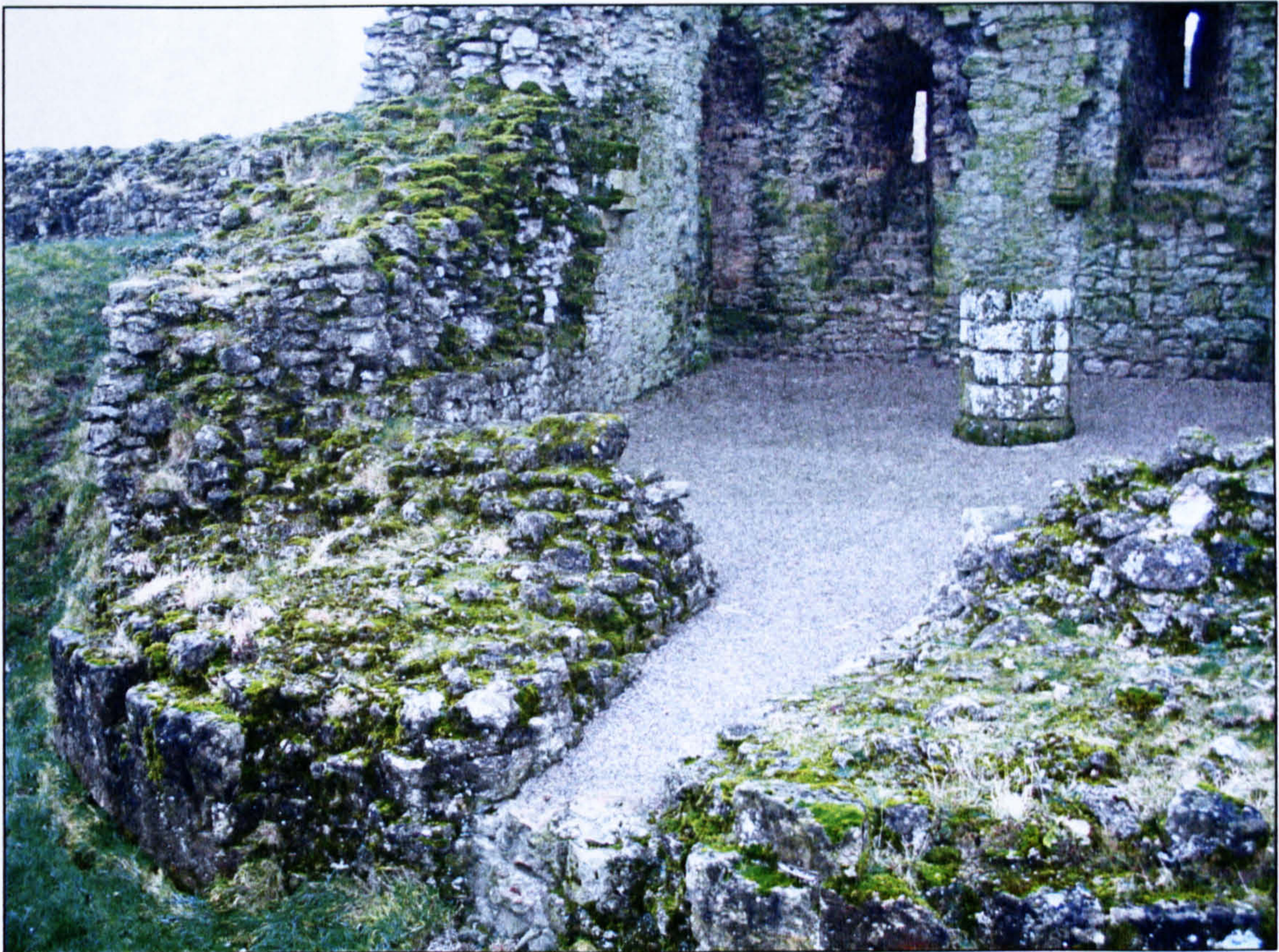
Figure 5.60 The northeast wall of the keep, looking south.
