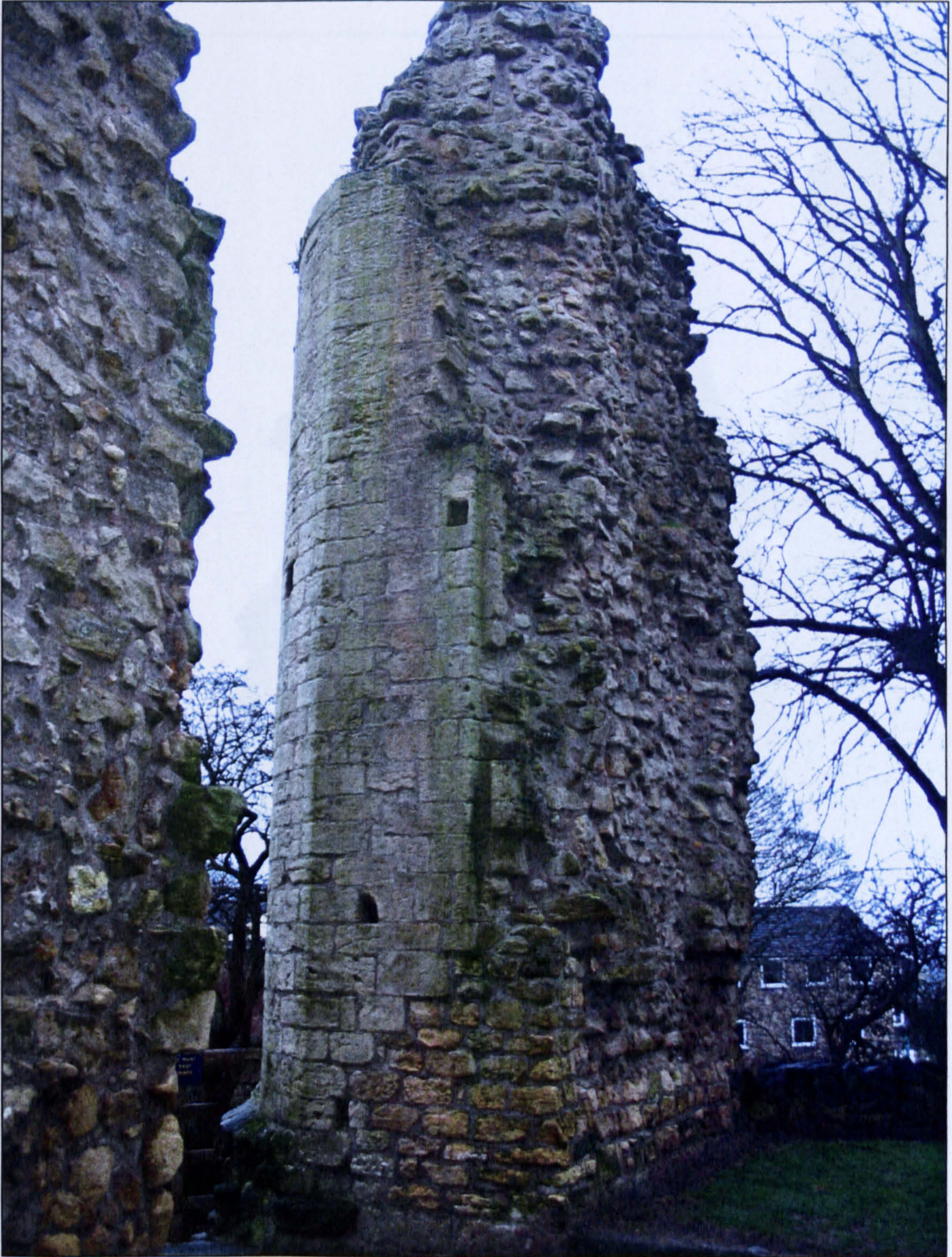
Figure 4.11 G1 with portcullis groove and putlog holes.
