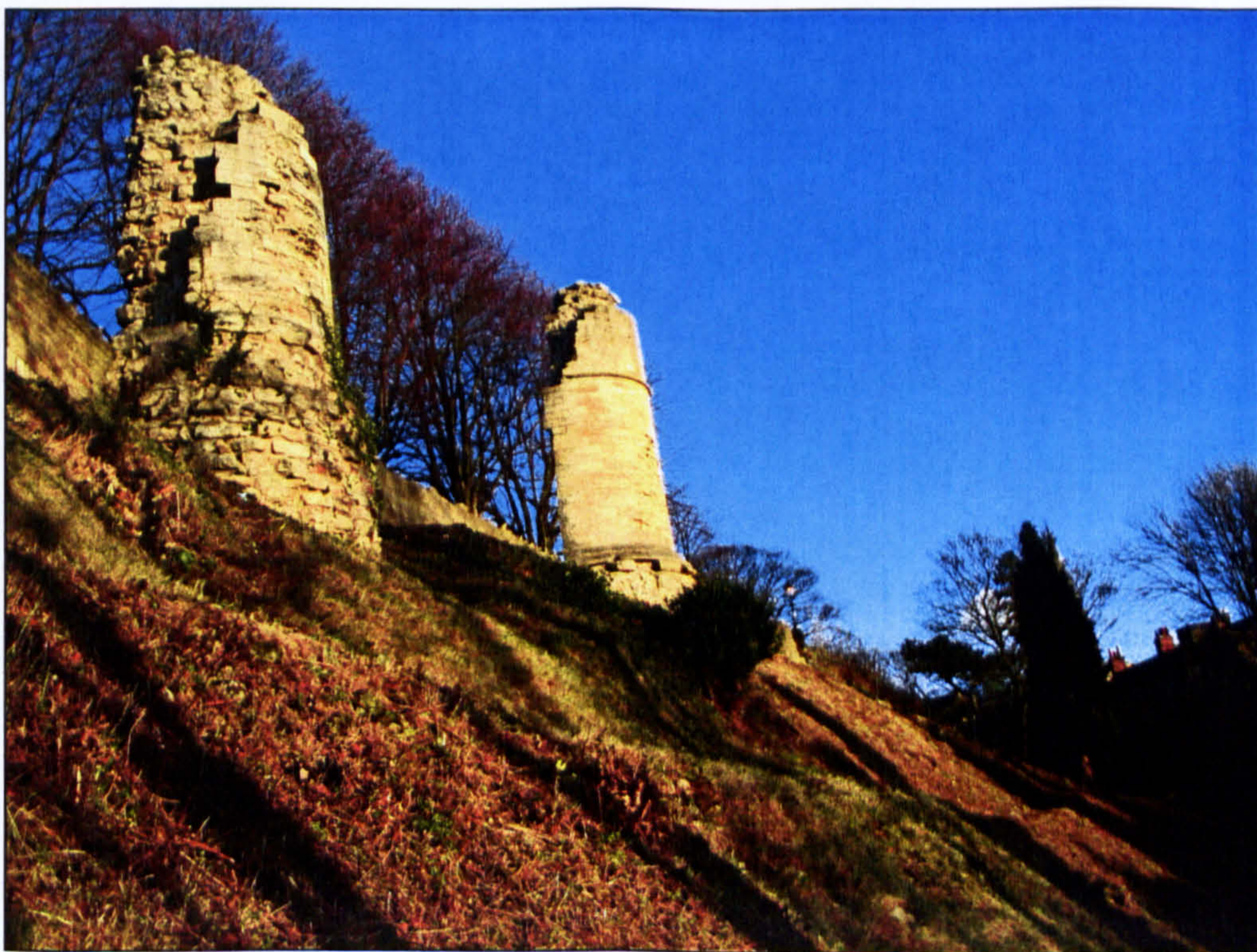
Figure 4.27 Steep incline of cliffside along T2 and T1.
