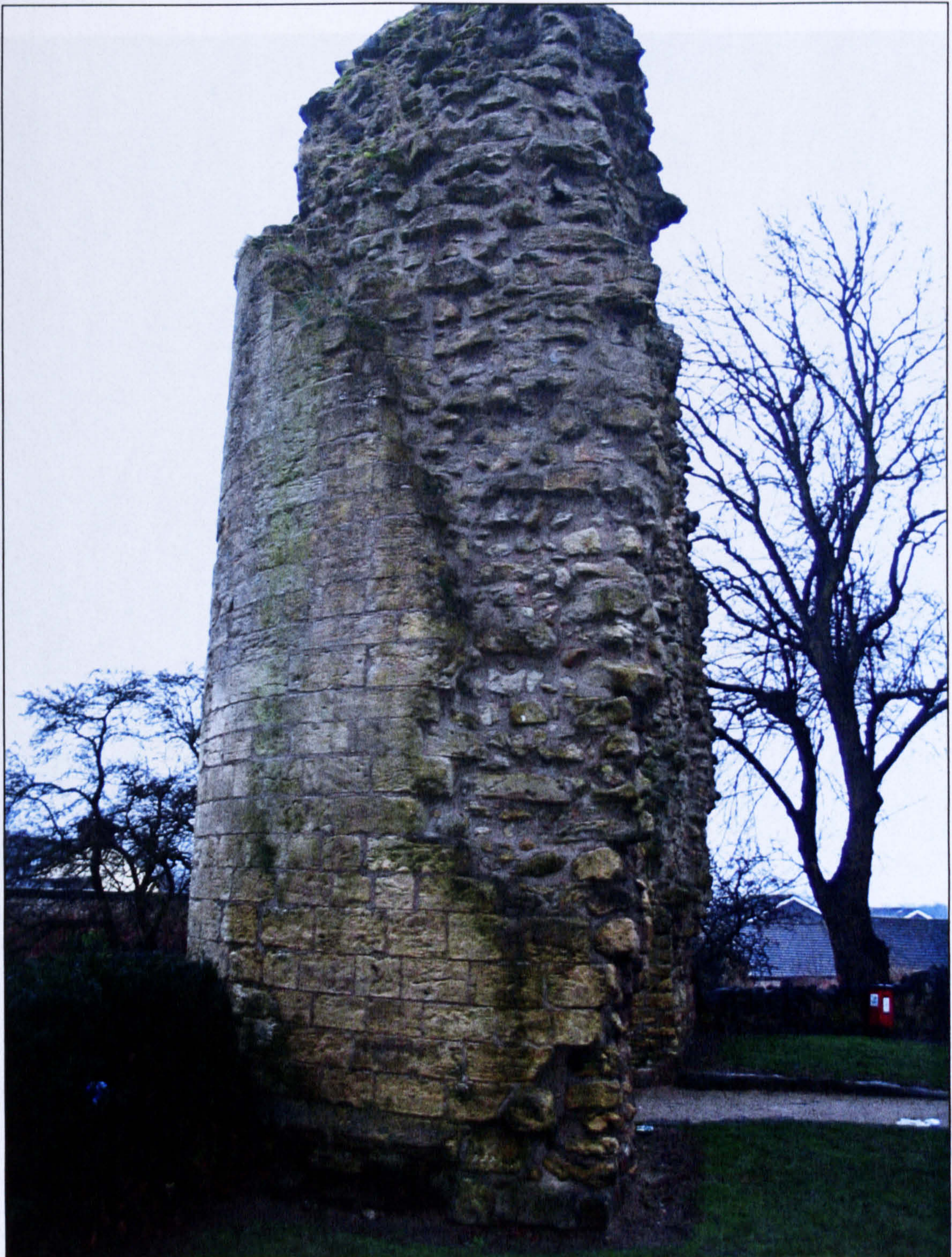
Figure 4.13 Outside view of G2.
