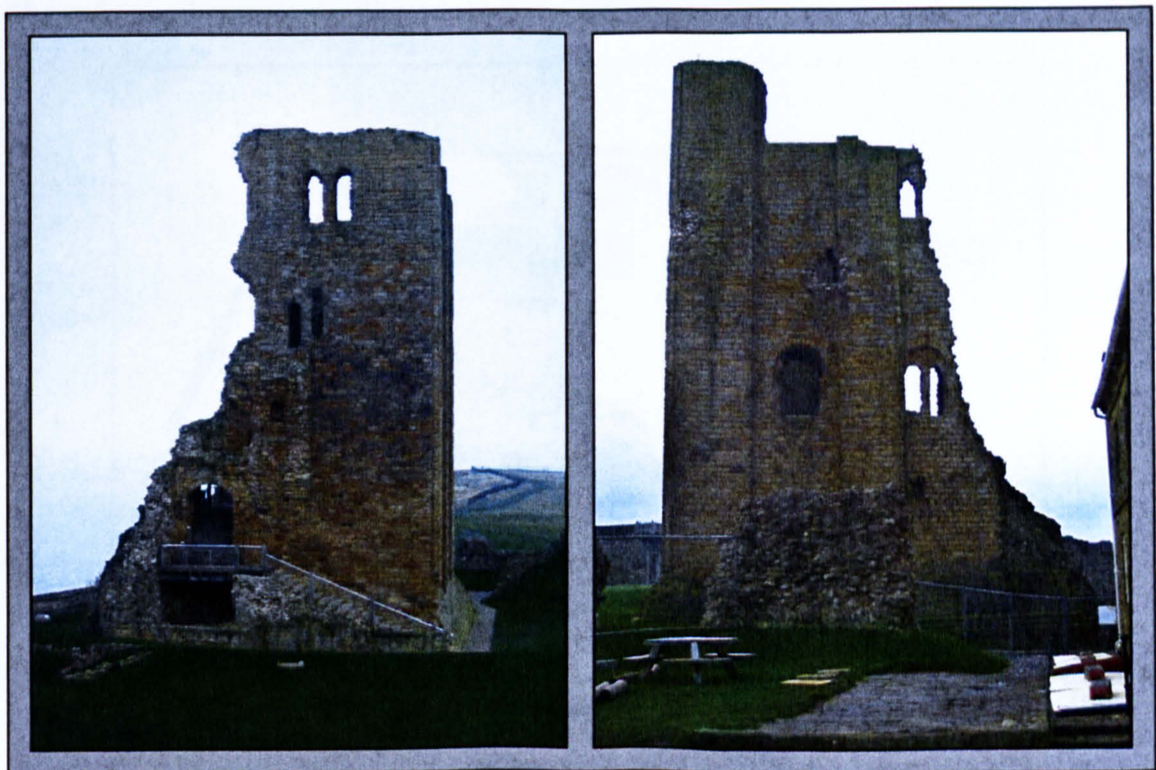
Figure 5.70 Profile views of Scarborough Castle Keep showing the destruction pattern of the remaining fabric. Left : Looking north. Right : Looking south.
