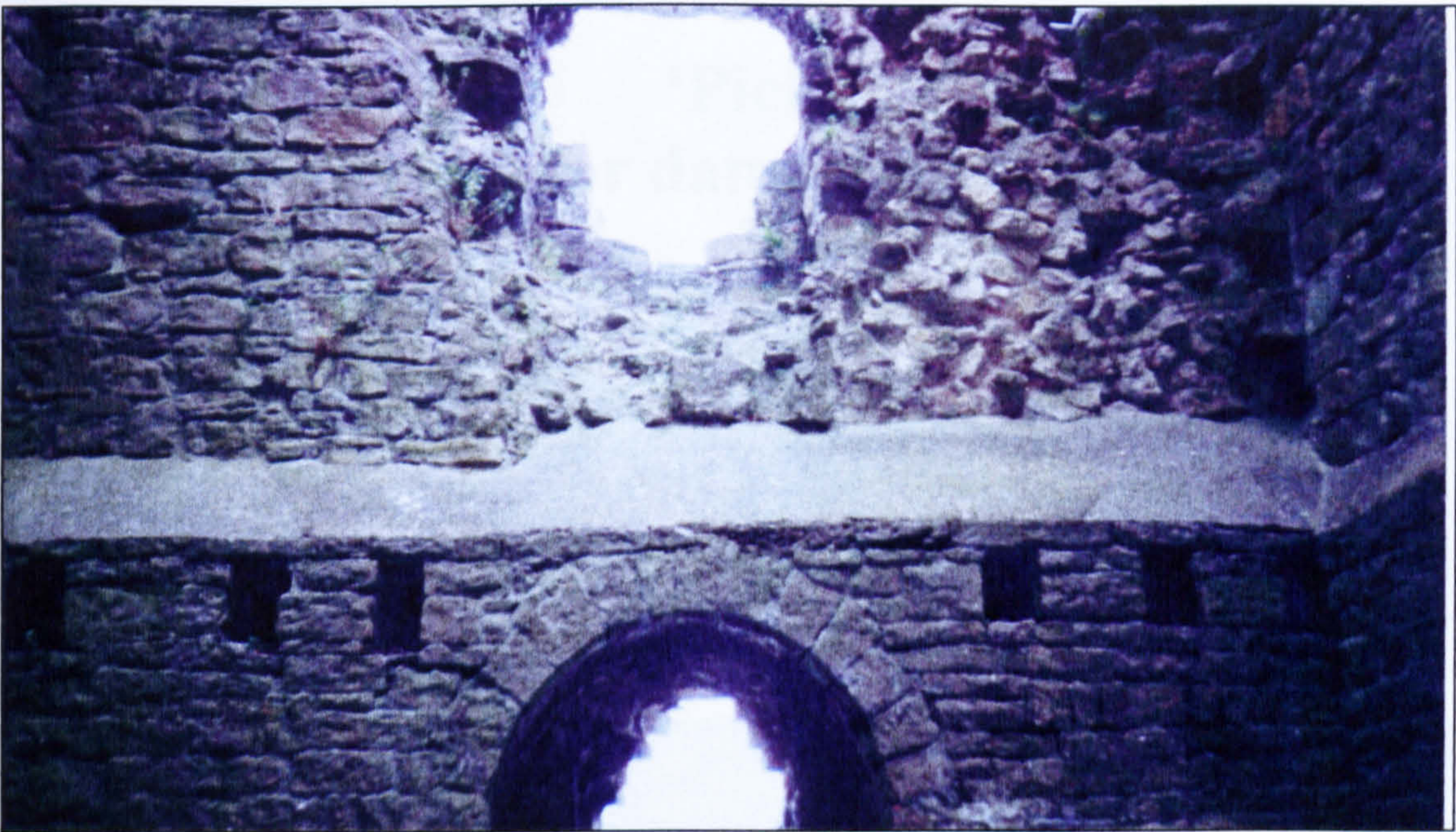
Figure 3.17 Interior of Clitheroe Castle Keep, showing use of cement in past conservation work.
