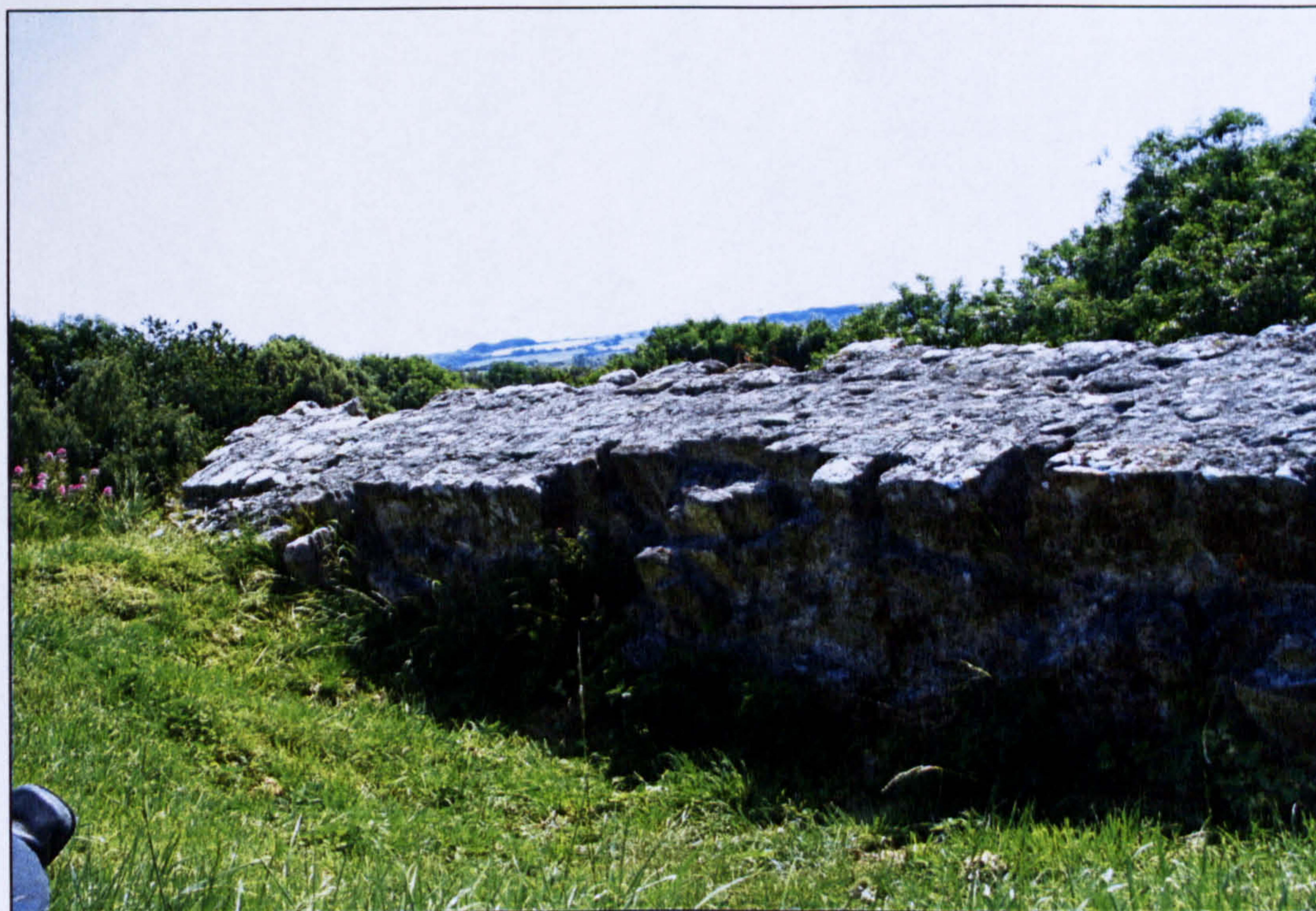
Figure 5.13 Overturned section of curtain wall on southwest side.
