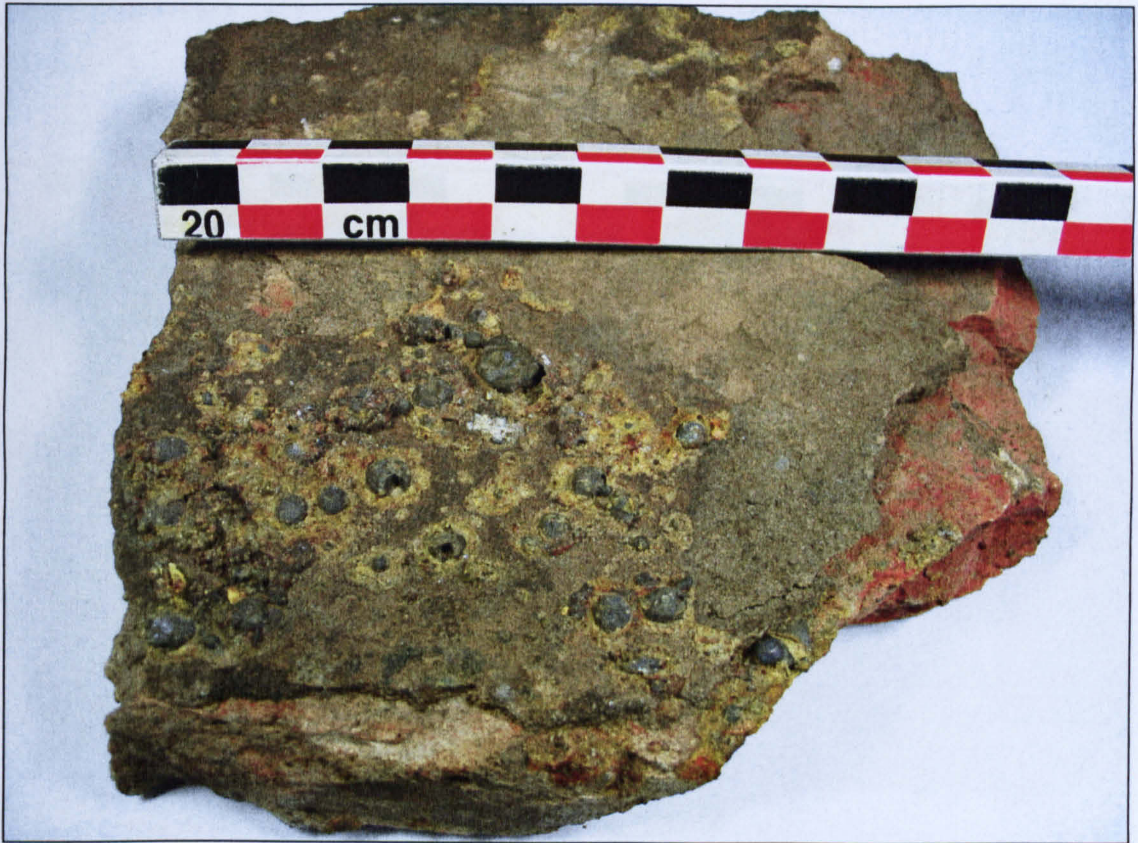
Figure 3.8 Fire damaged tile with melted drops of lead attached (Allerton Castle).
