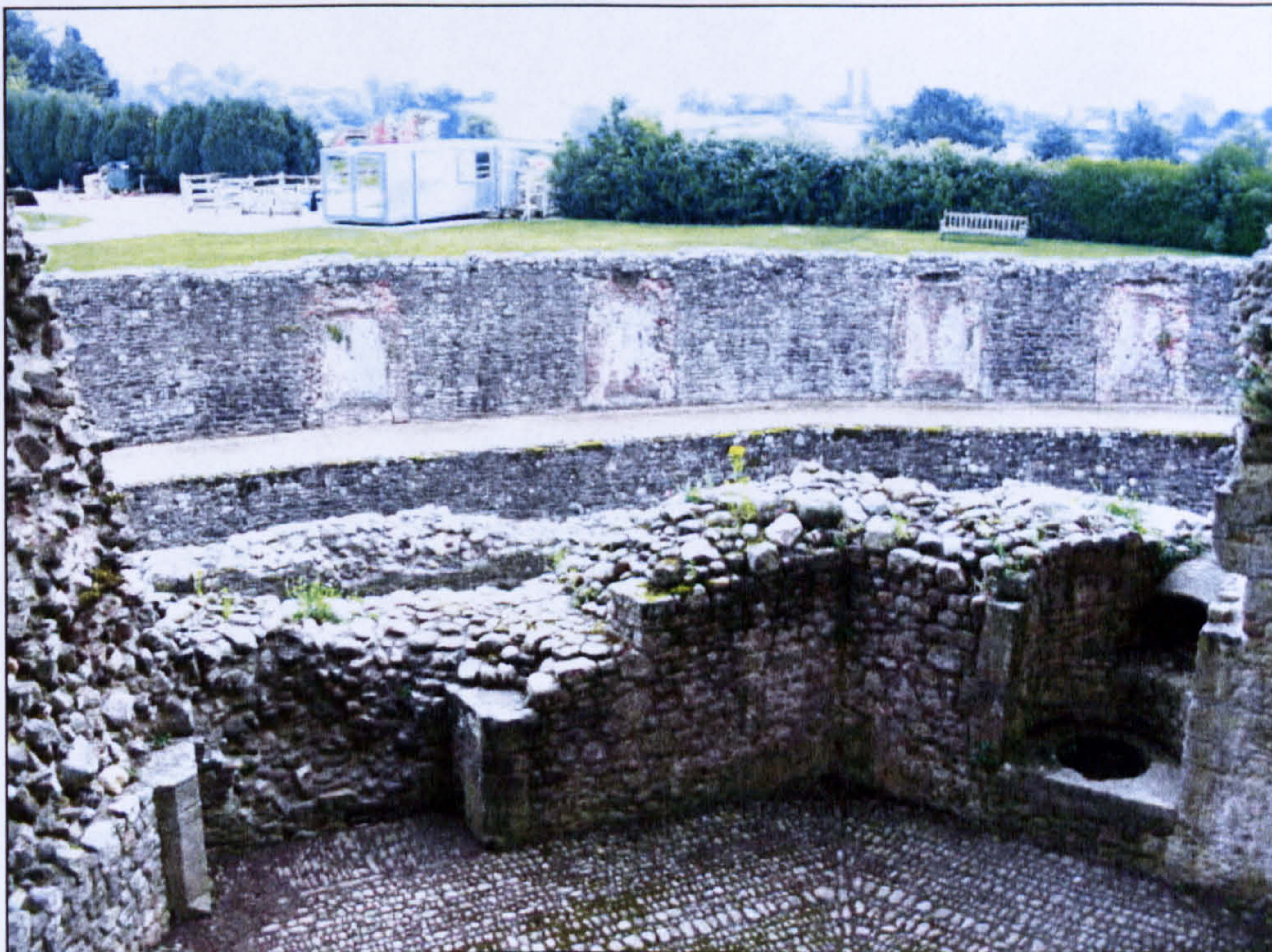
Figure 5.42 The remains of the damaged wall, showing two structural voids in the form of a fireplace (left) and well (right).
