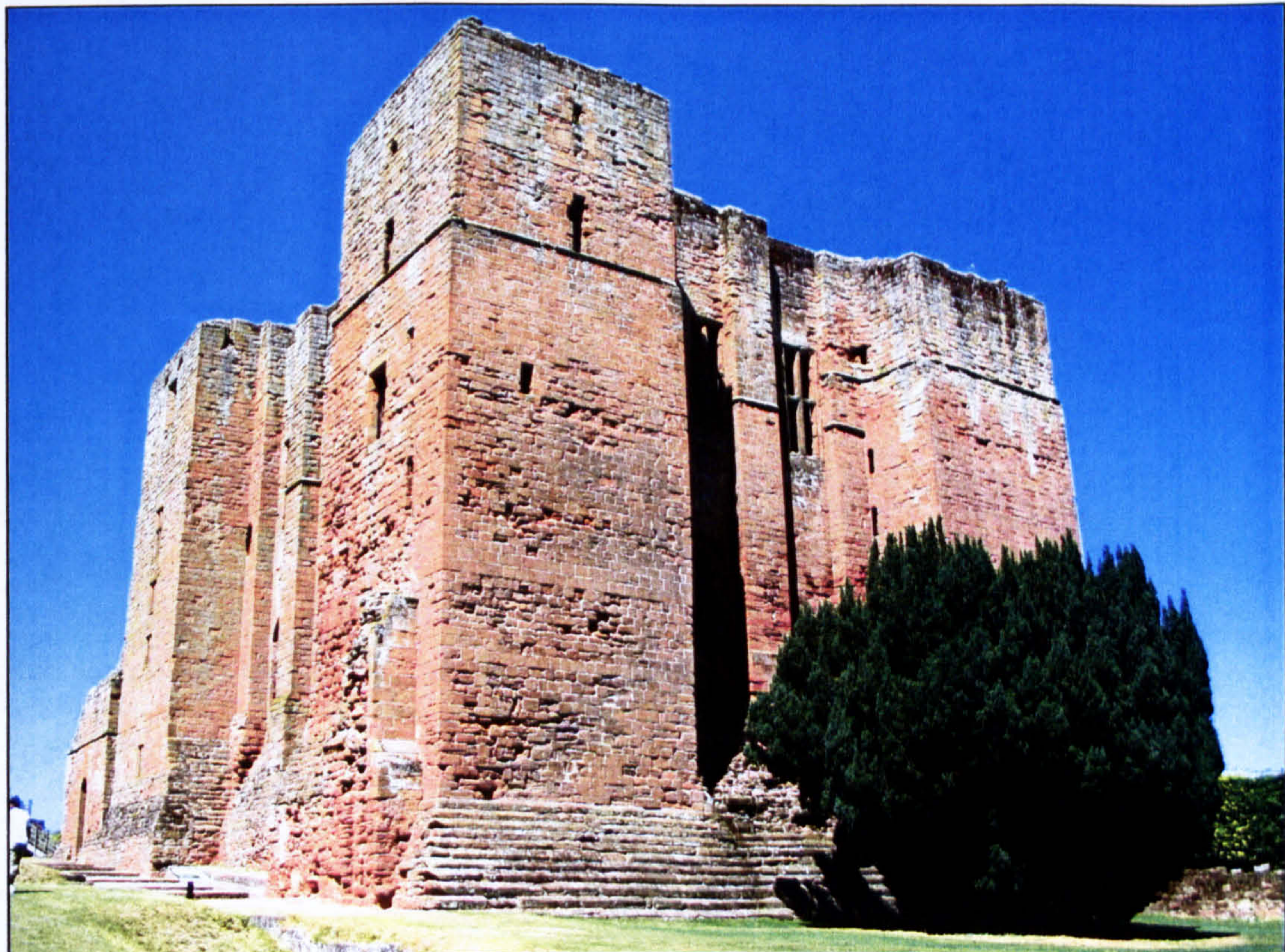
Figure 6.19 The keep from the southeast, showing its solid Norman construction and corner turrets.
