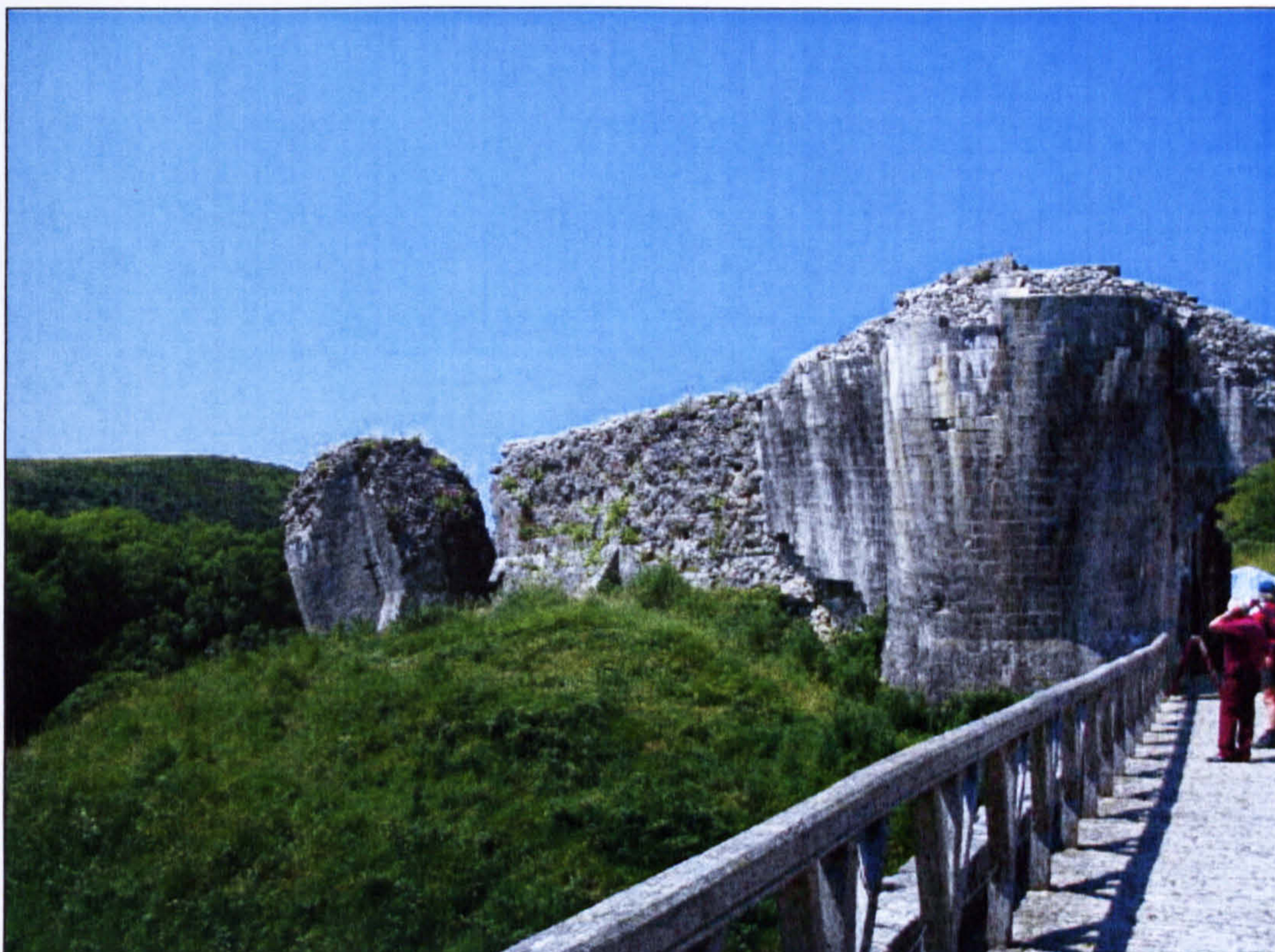
Figure 5.6 The western half of the Outer Gatehouse [13] and the First Tower [1], looking northwest.
