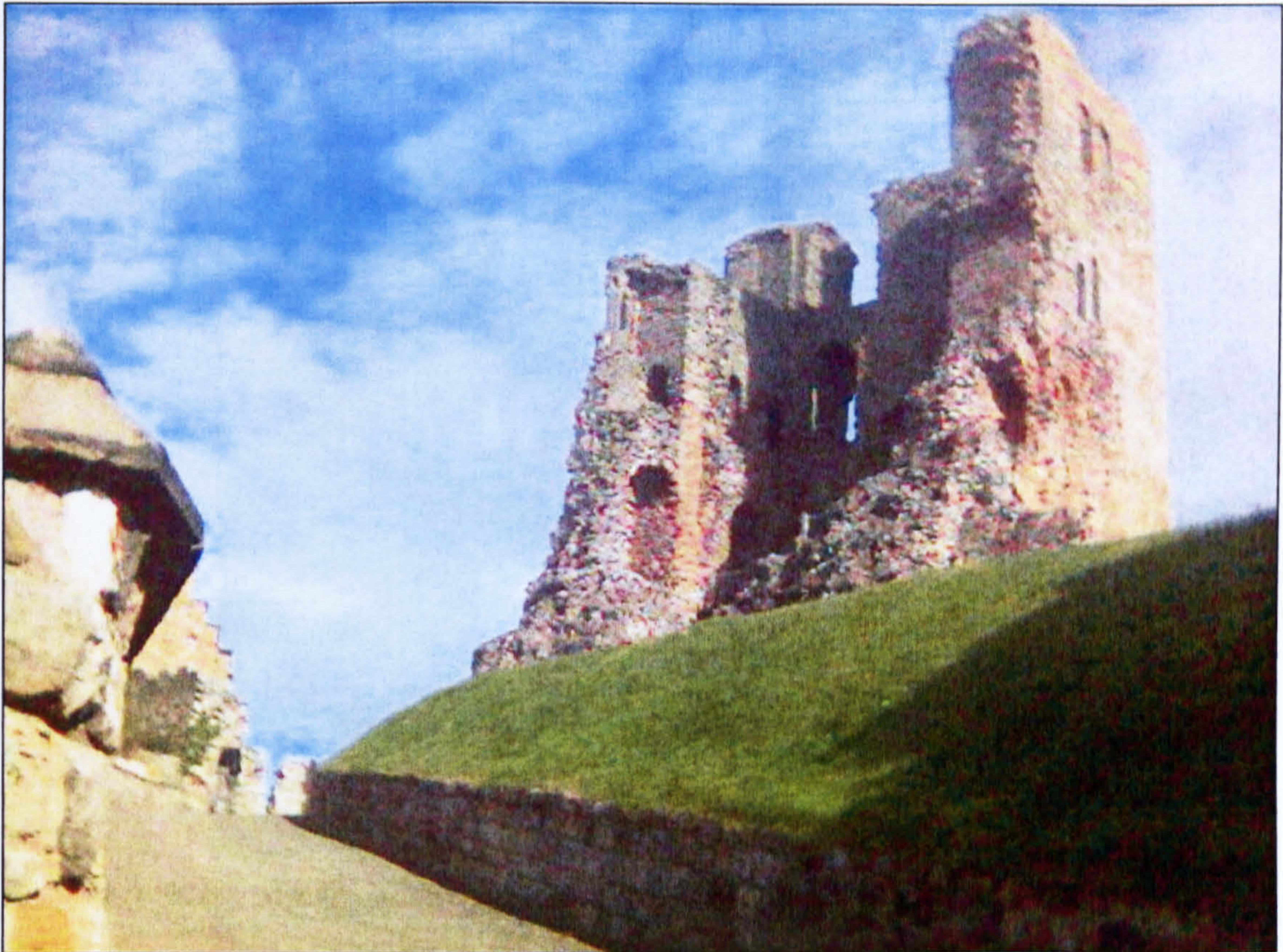
Figure 5.65 The collapsed west wall of Scarborough Castle Keep (Yorkshire), looking northeast.
