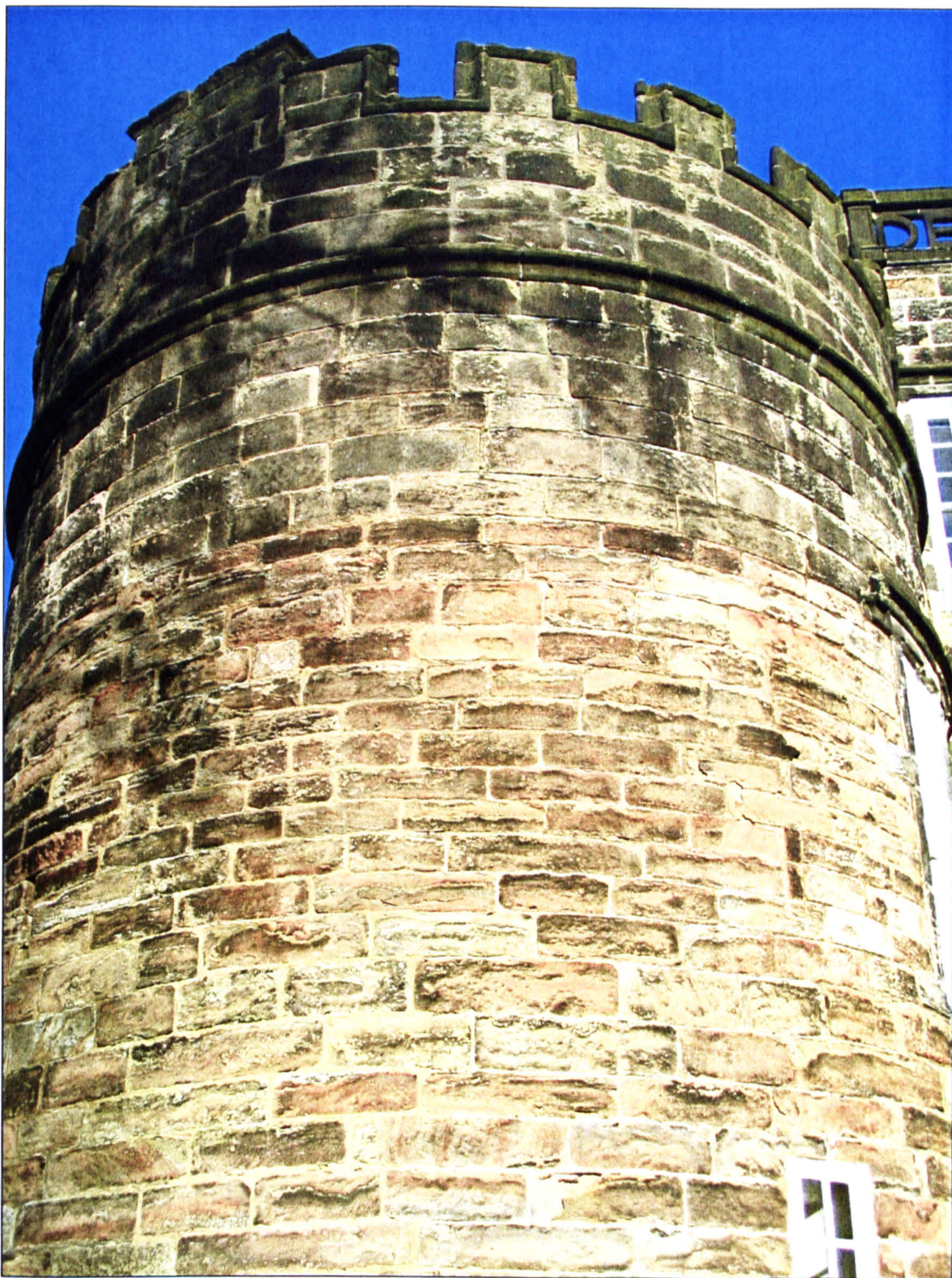
Figure 4.2 Close-up of the left turret of the Outer Gate, Skipton Castle, detailing pre- and post-slighting construction.
