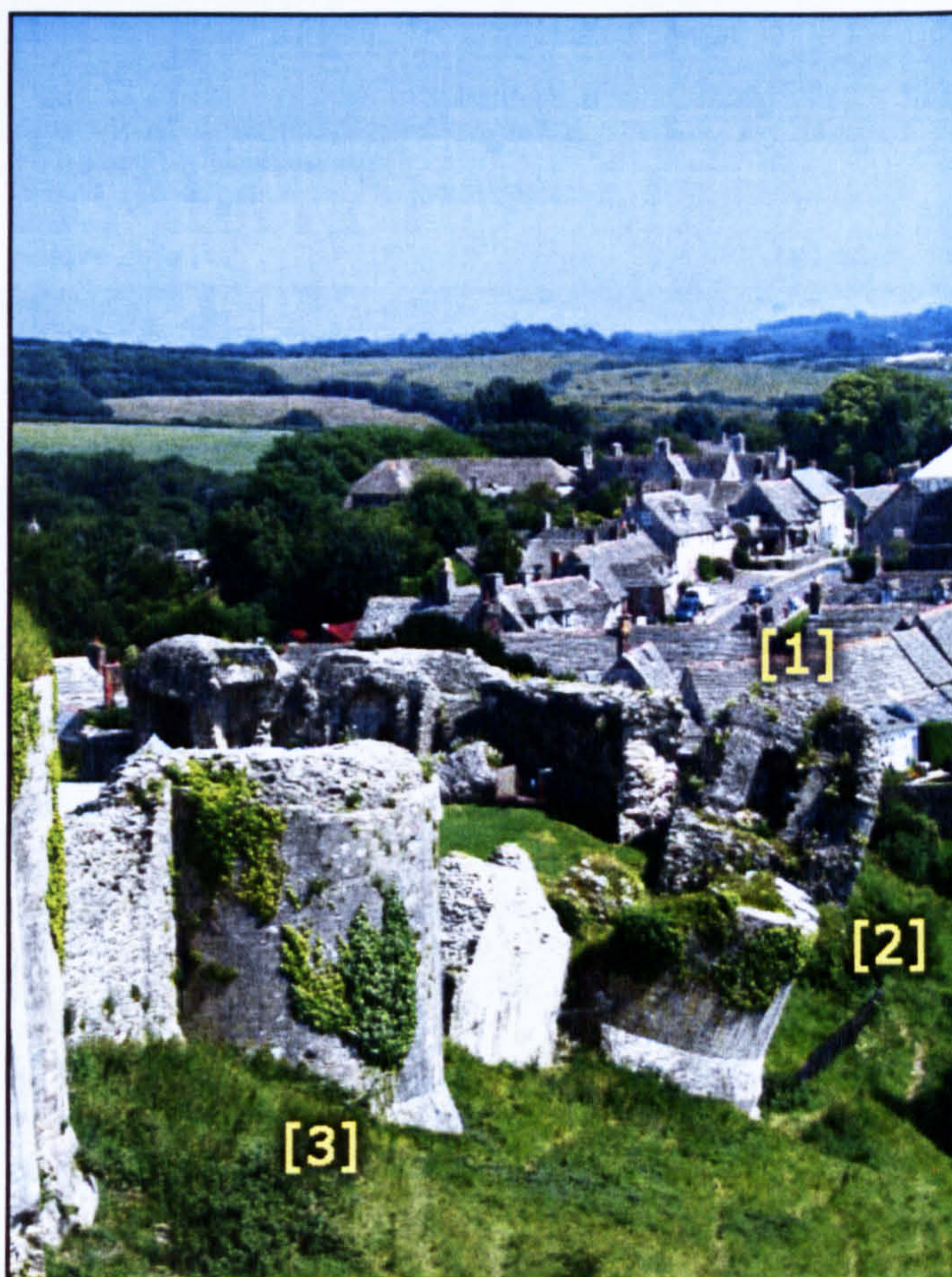
Figure 5.7 The southwestern curtain wall and towers, showing the First Tower [1], the Second Tower [2], and the Third Tower [3].
