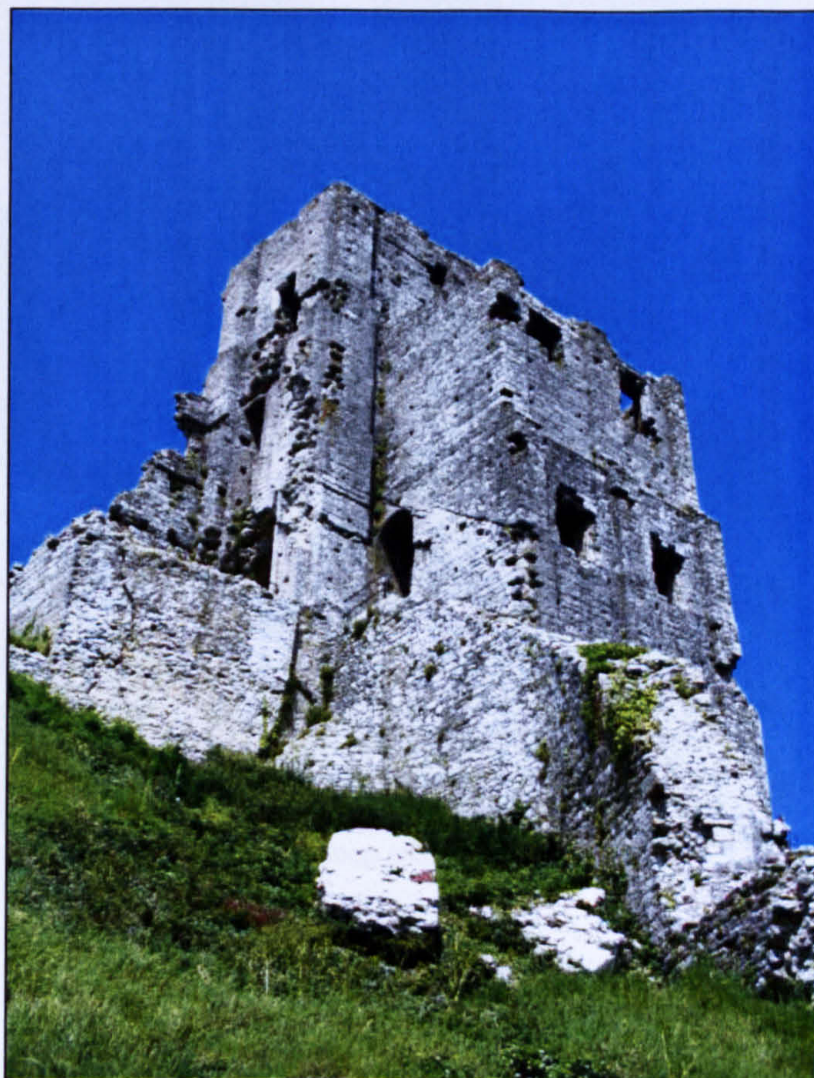
Figure 5.25 Southwest elevation of Corfe Castle Keep.
