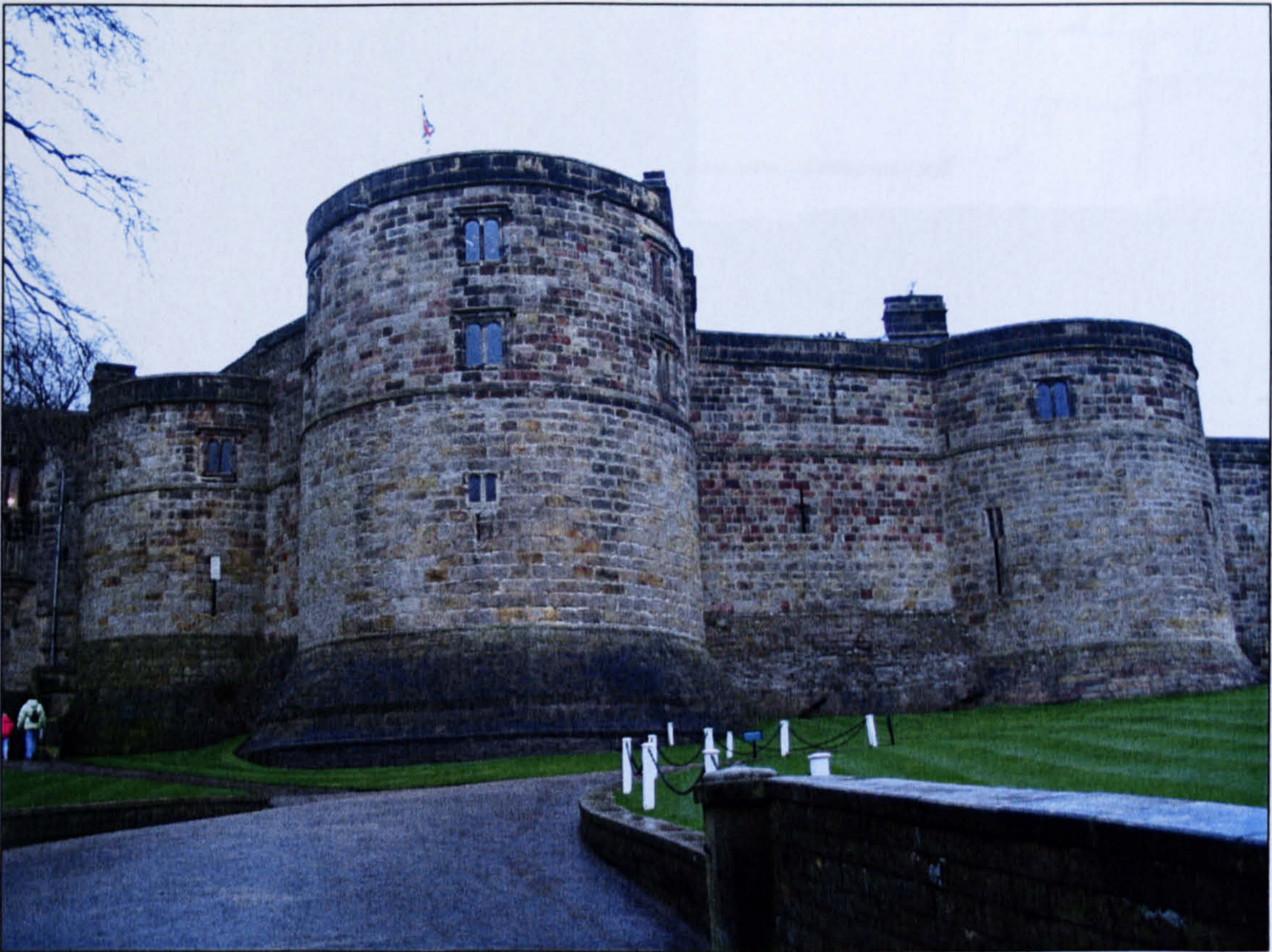
Figure 4.3 The outside of the watchtower, Skipton Castle, with the larger windows and different stonework of the re-build visible in the upper courses.
