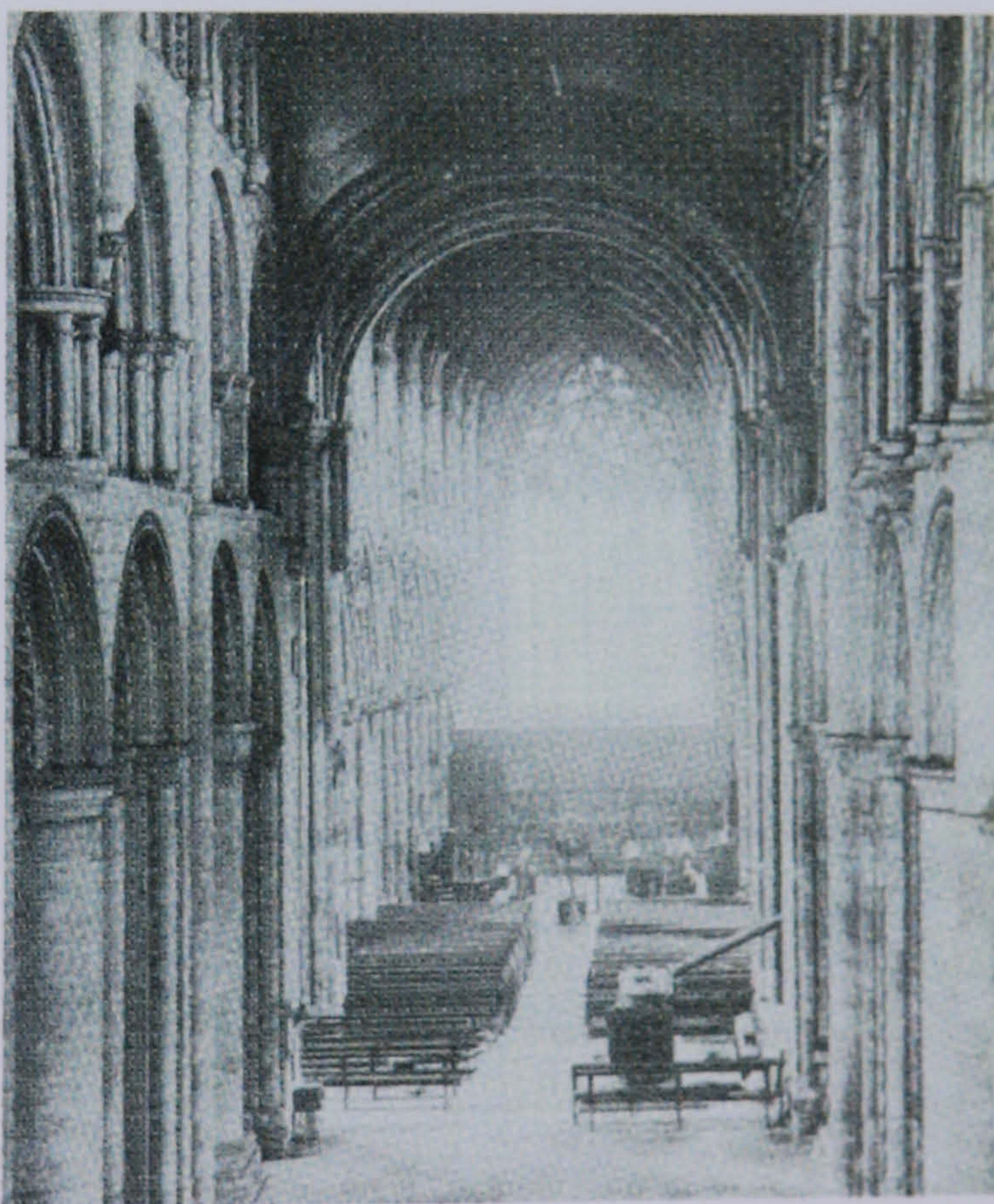
Figure 6.13 Nave of Selby Abbey looking east in the 1870s
