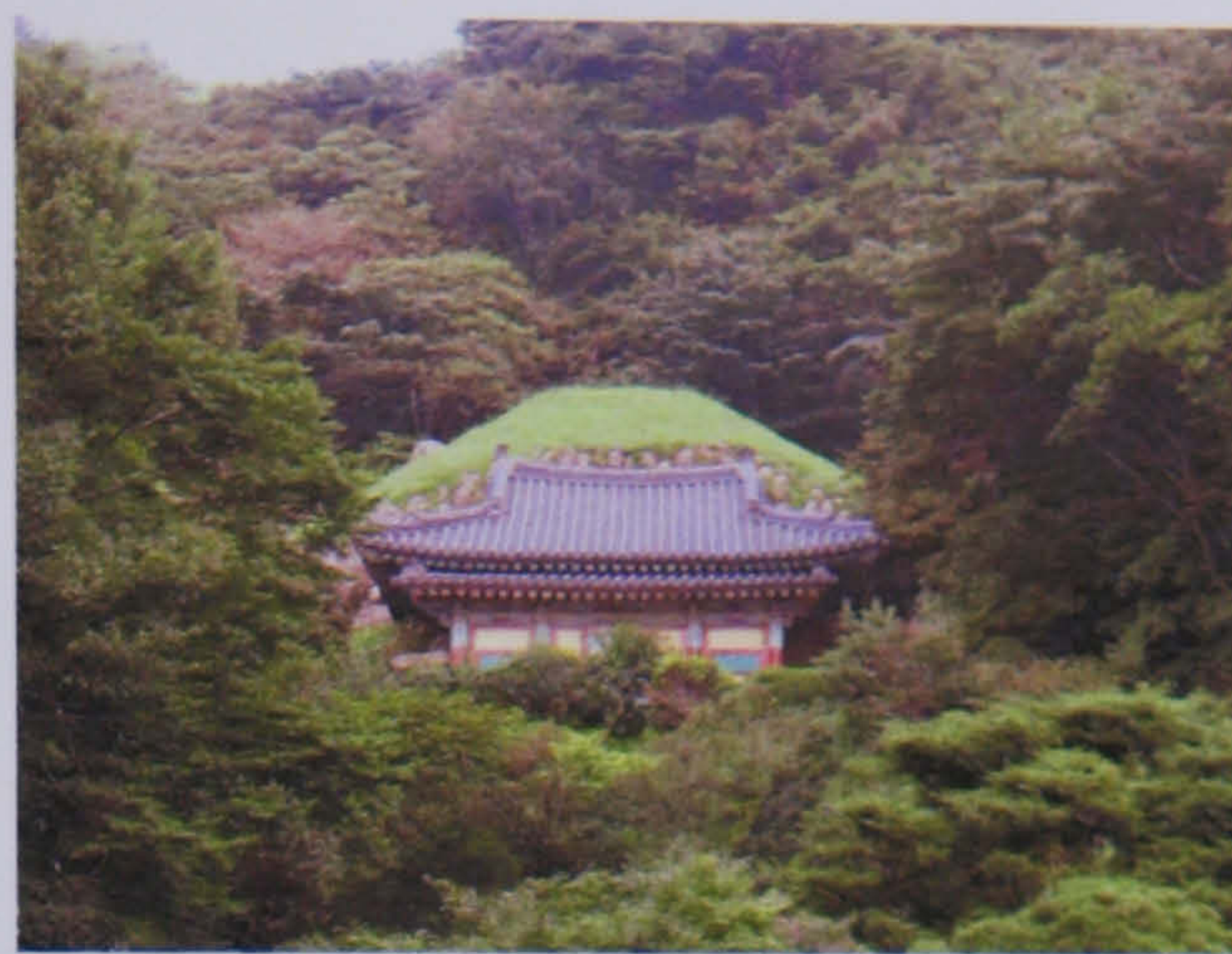
Figure 5.23 Present wooden structure of Seokuram which was added in the 1960s
