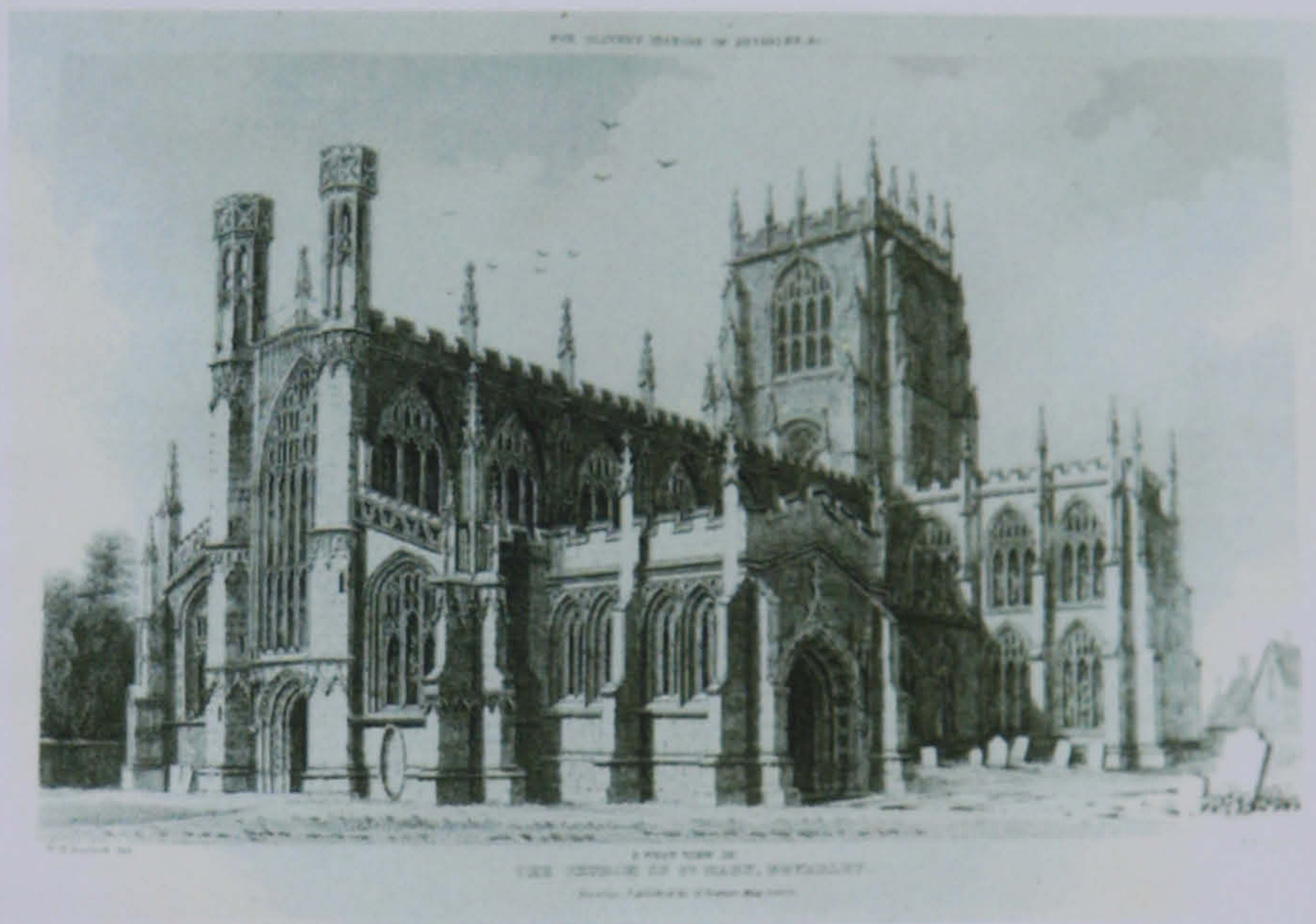
Figure 6.42 St Mary's Church before Pugin's restoration
