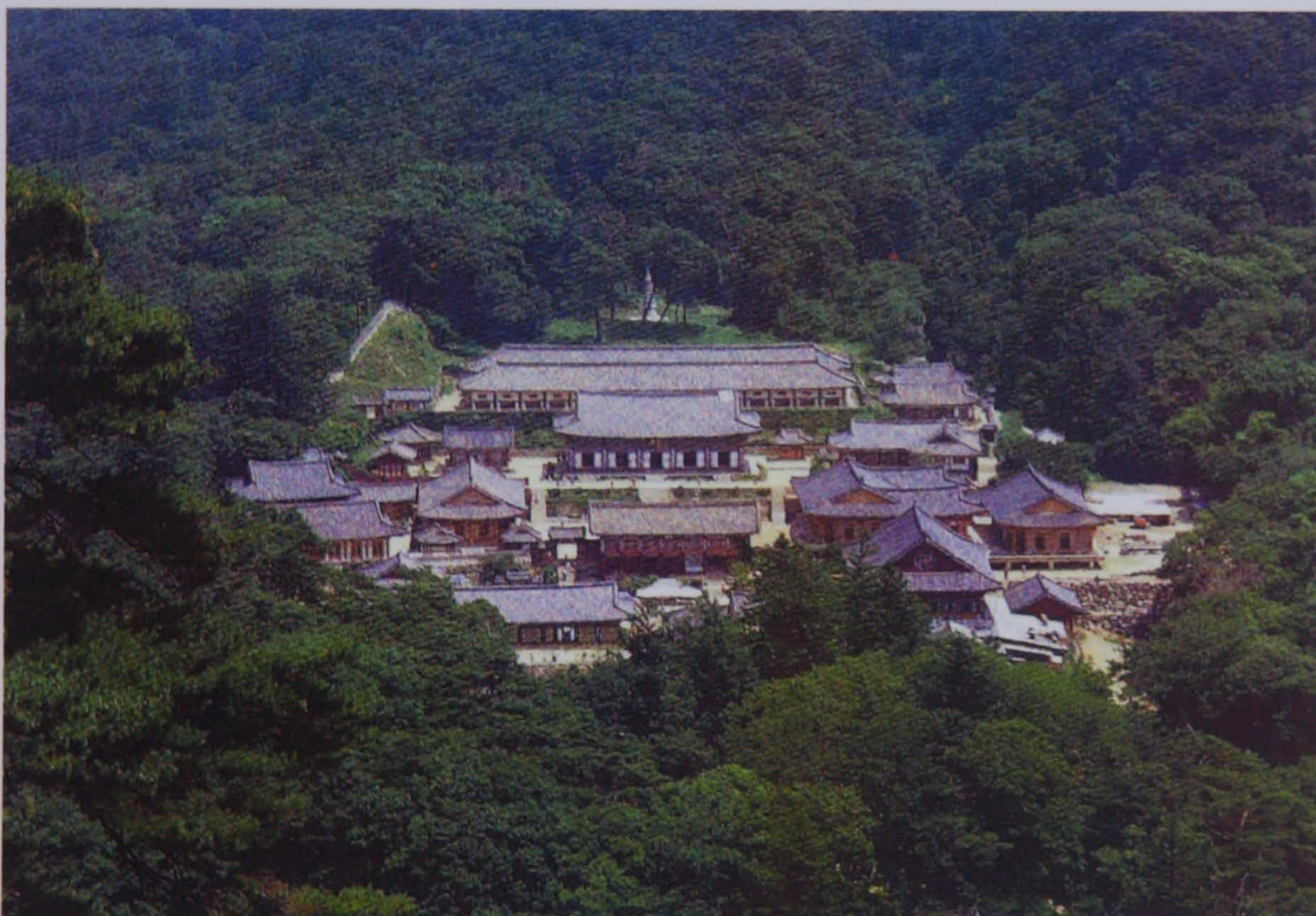
Figure 3.21 Aerial view of Haeinsa
