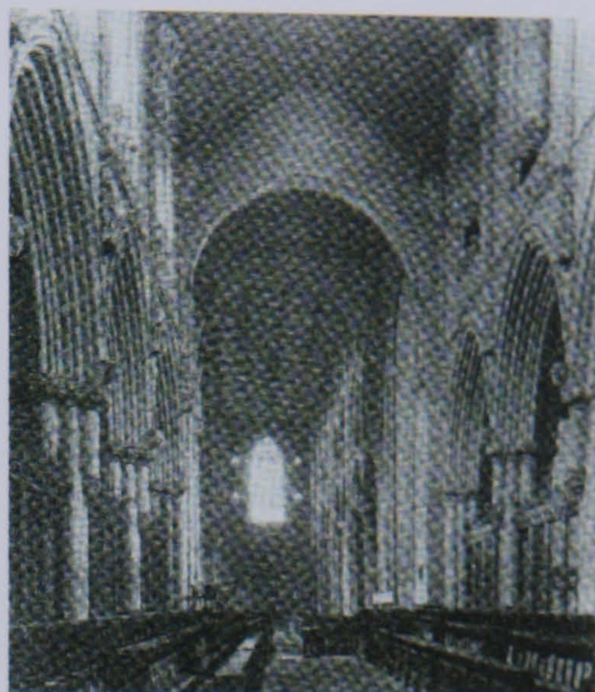
Figure 6.17 The ceiling of crossing of Selby Abbey showing the restored wooden vault
