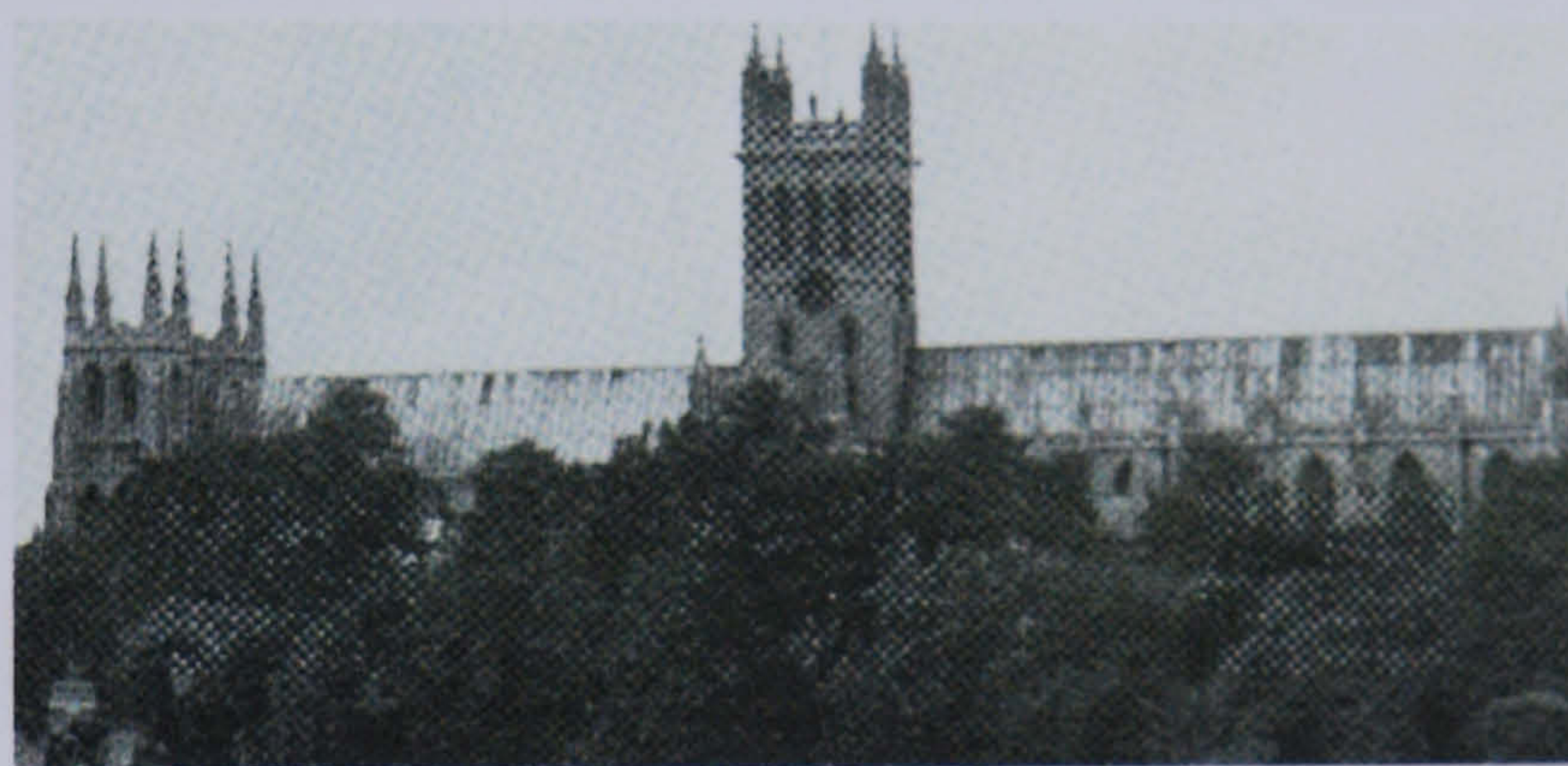
Figure 6.7 South front of Selby Abbey after rebuilding the central tower in 1909
