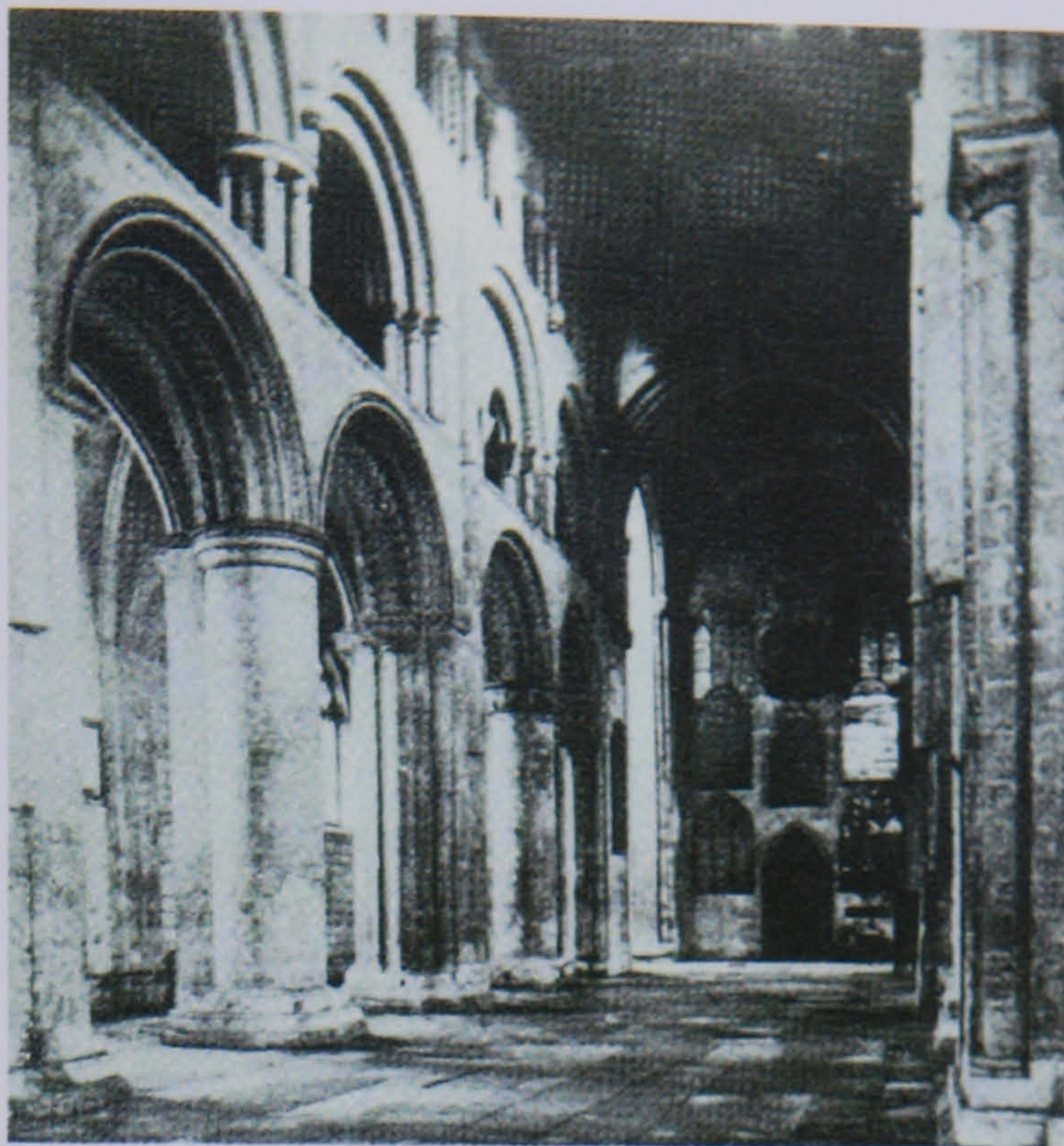
Figure 6.12 Nave of Selby Abbey looking east in the 1860s
