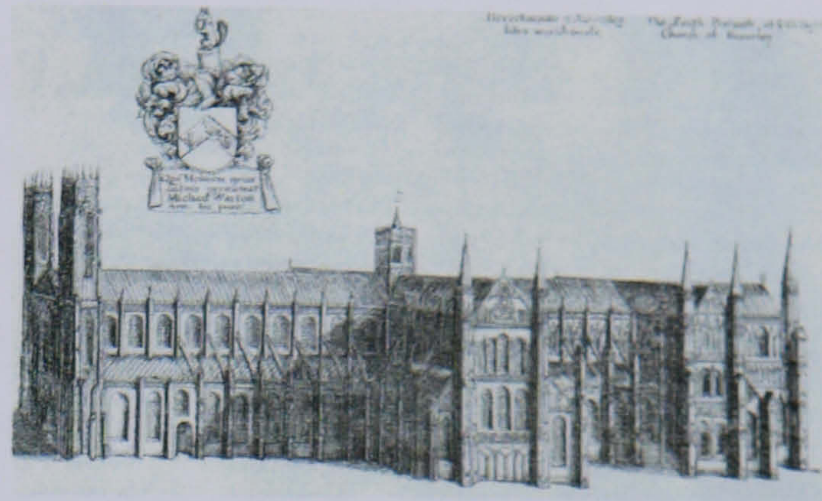
Figure 6.23 Lantern tower in the 17 th century in Beverley Minster
