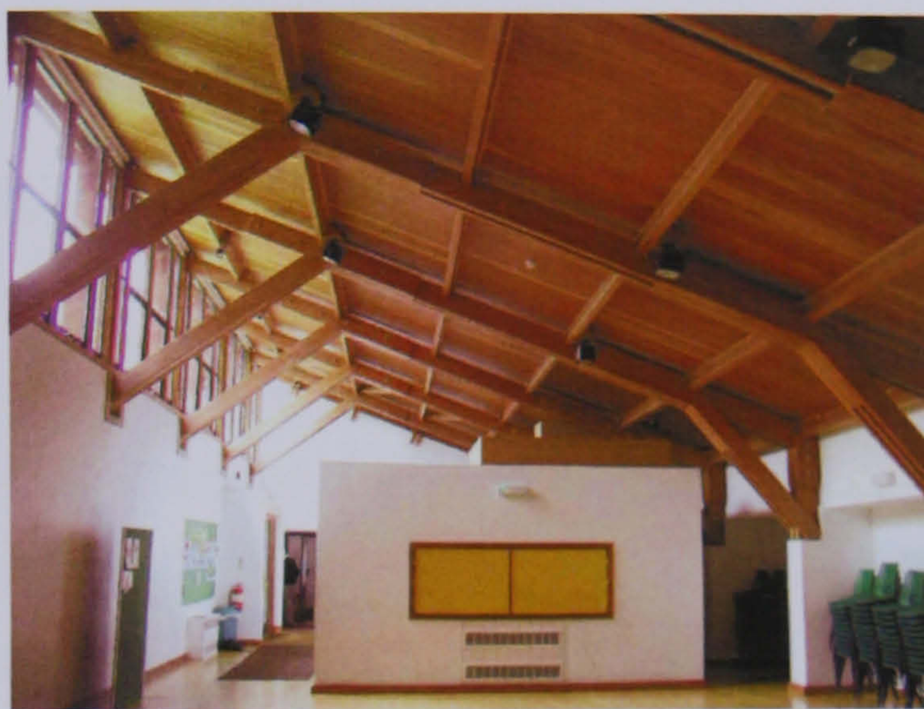
Figure 5.56 Interior of the parish hall of St Mary’s, Beverley
