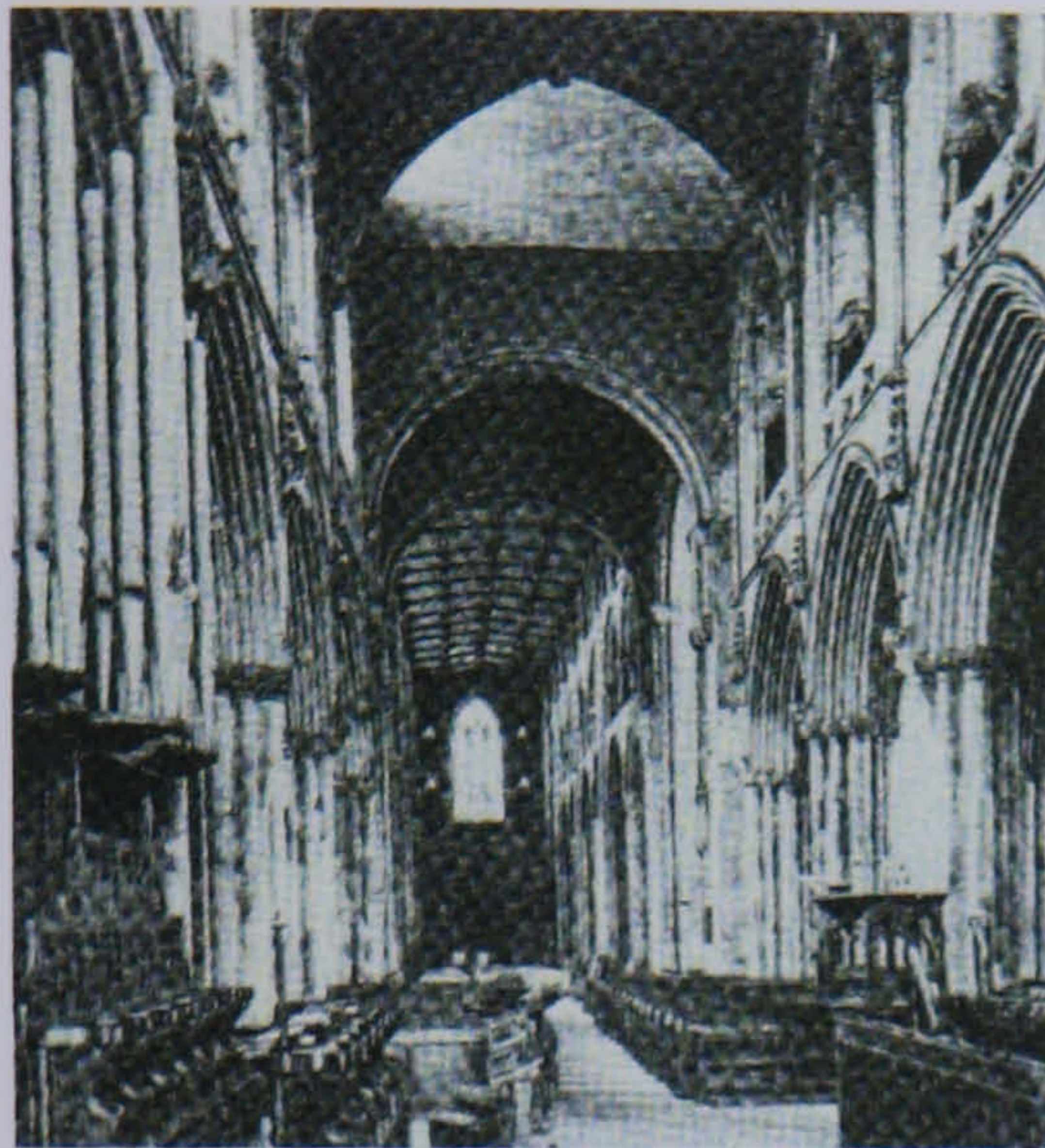
Figure 6.16 The ceiling of crossing of Selby Abbey before it was opened
