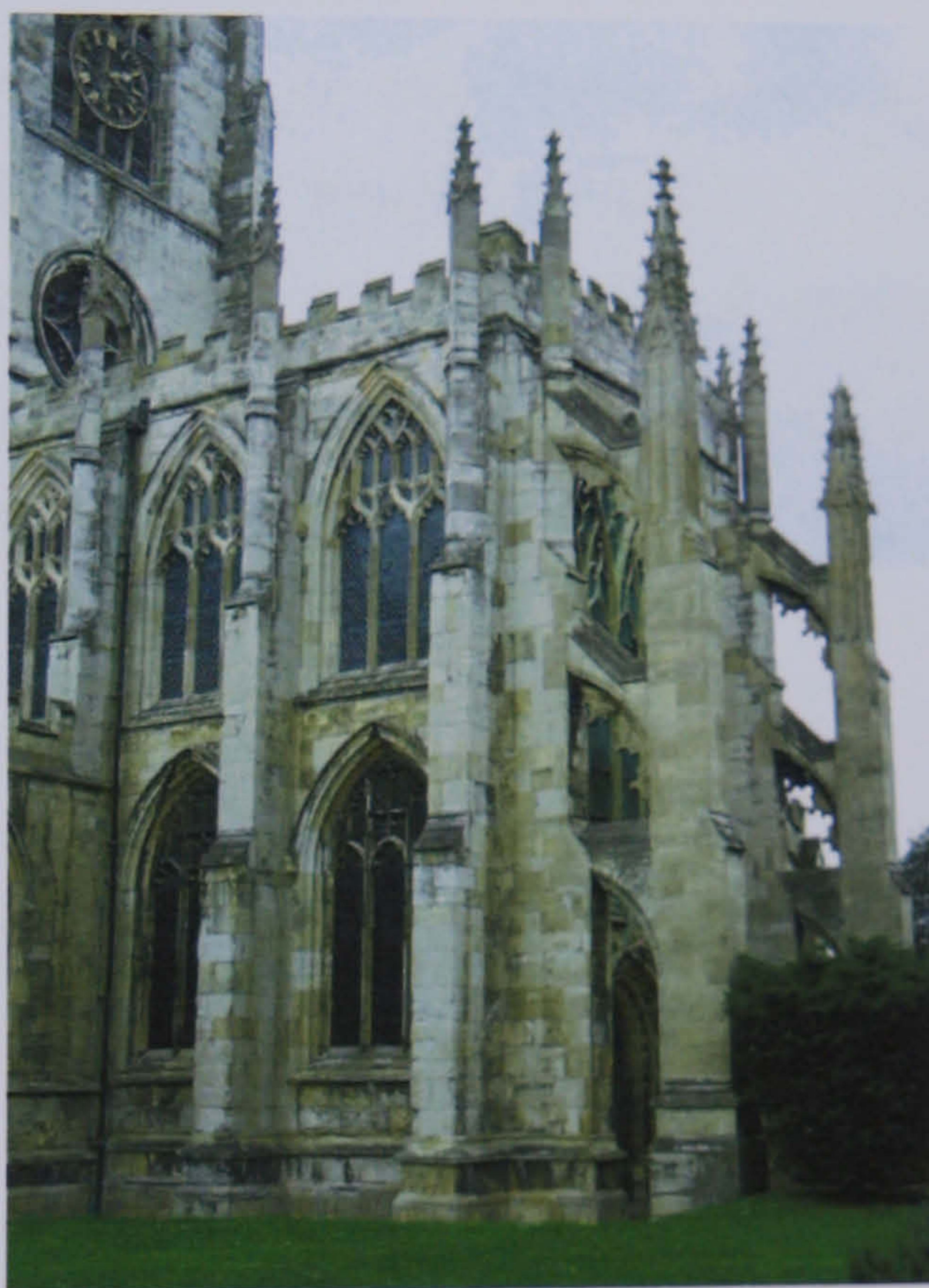
Figure 6.44 Flying buttress to the end of south transept of St Mary's Church
