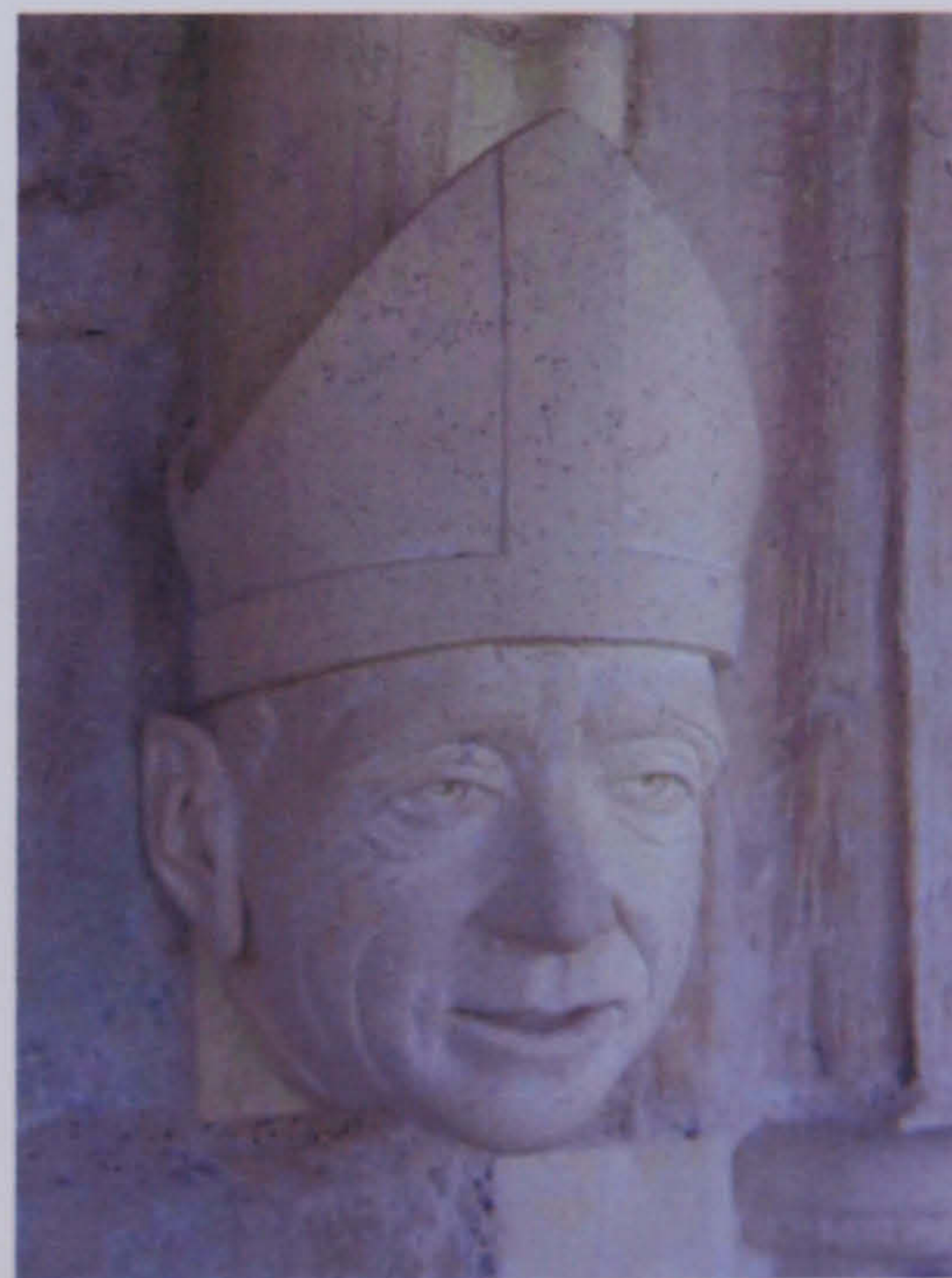
Figure 3.5 A new label stop of the former Archbishop of York in Selby Abbey
