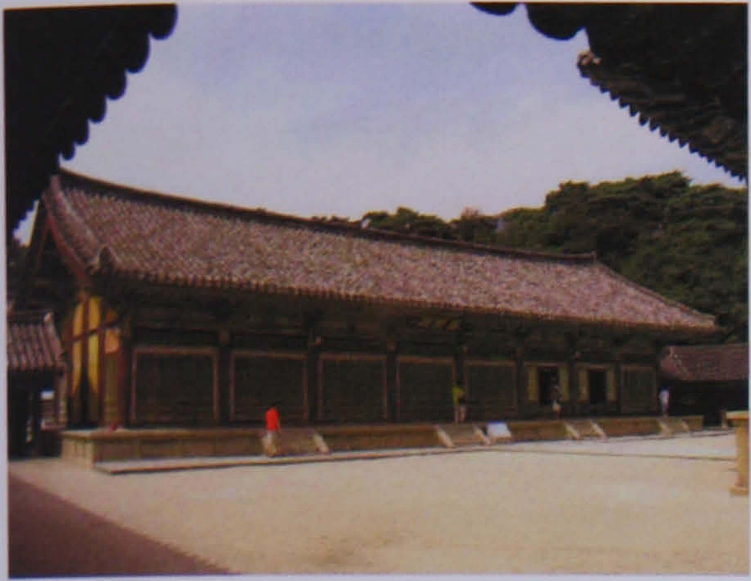
Figure 5.38 Museoljeon of Bulguksa after construction
