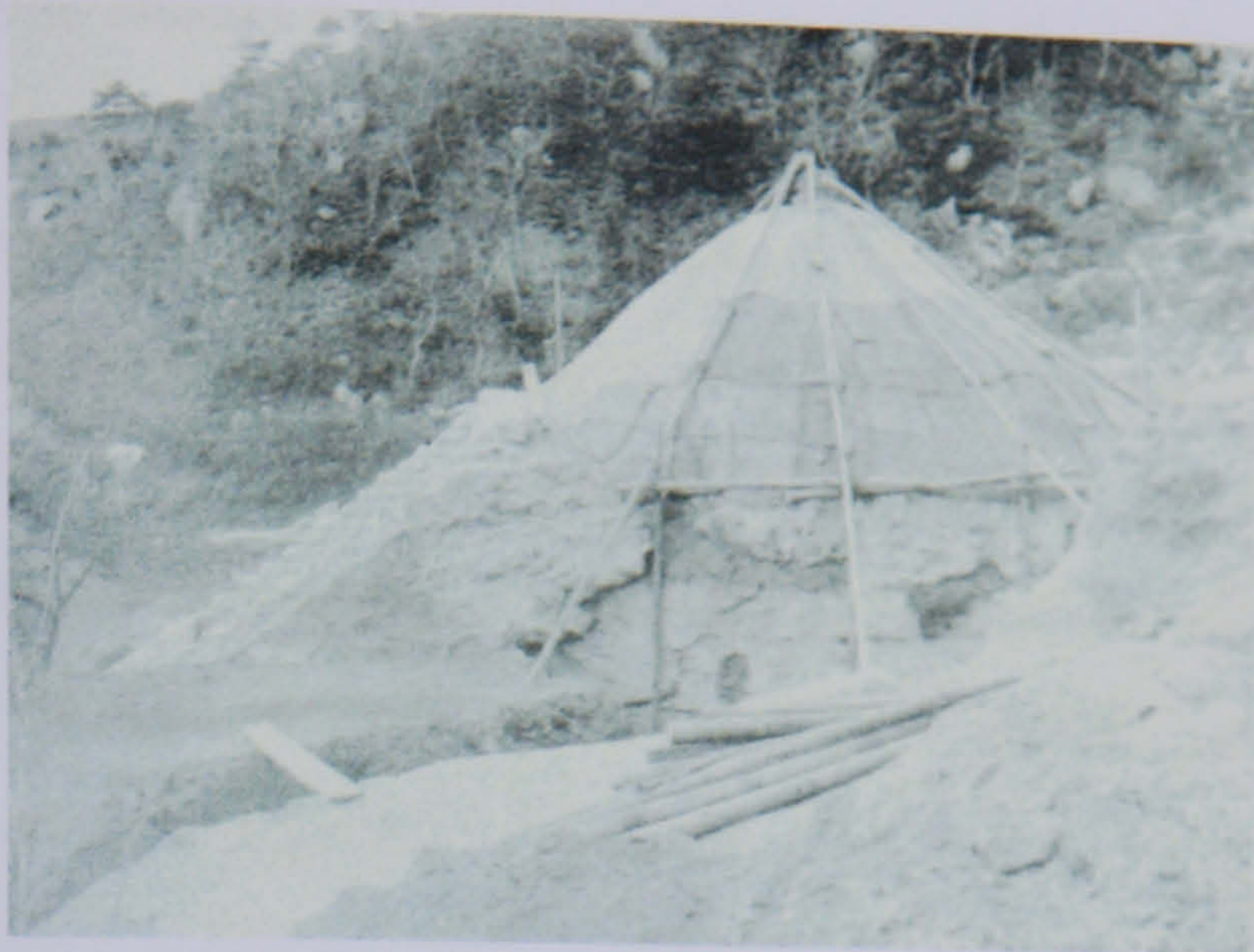
Figure 6.58 Cement reinforcement on the dome of the main chamber of Seokuram during Japanese restoration
