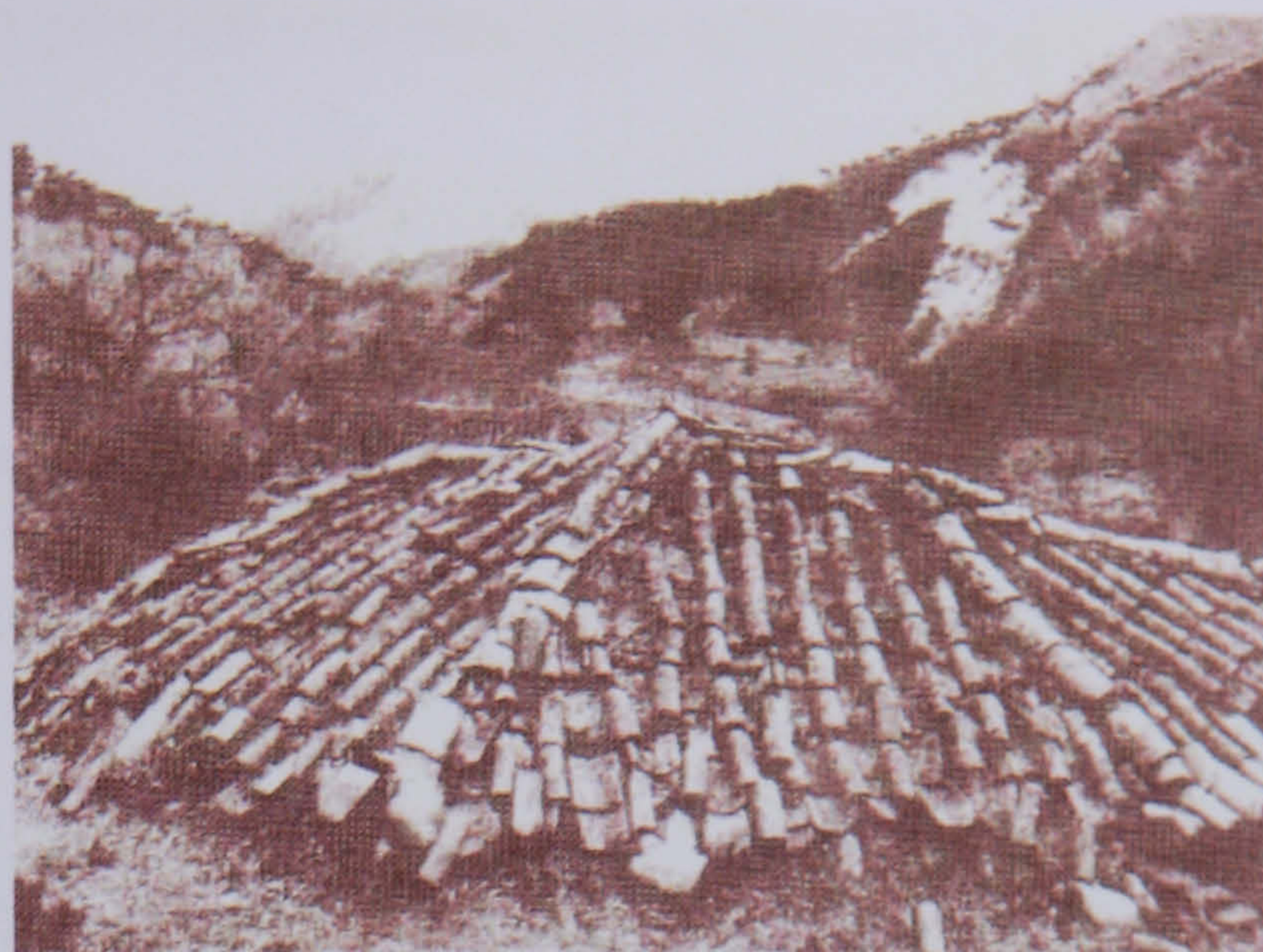
Figure 5.27 Roof tiles on the dome of the main chamber before the 1910s restoration
