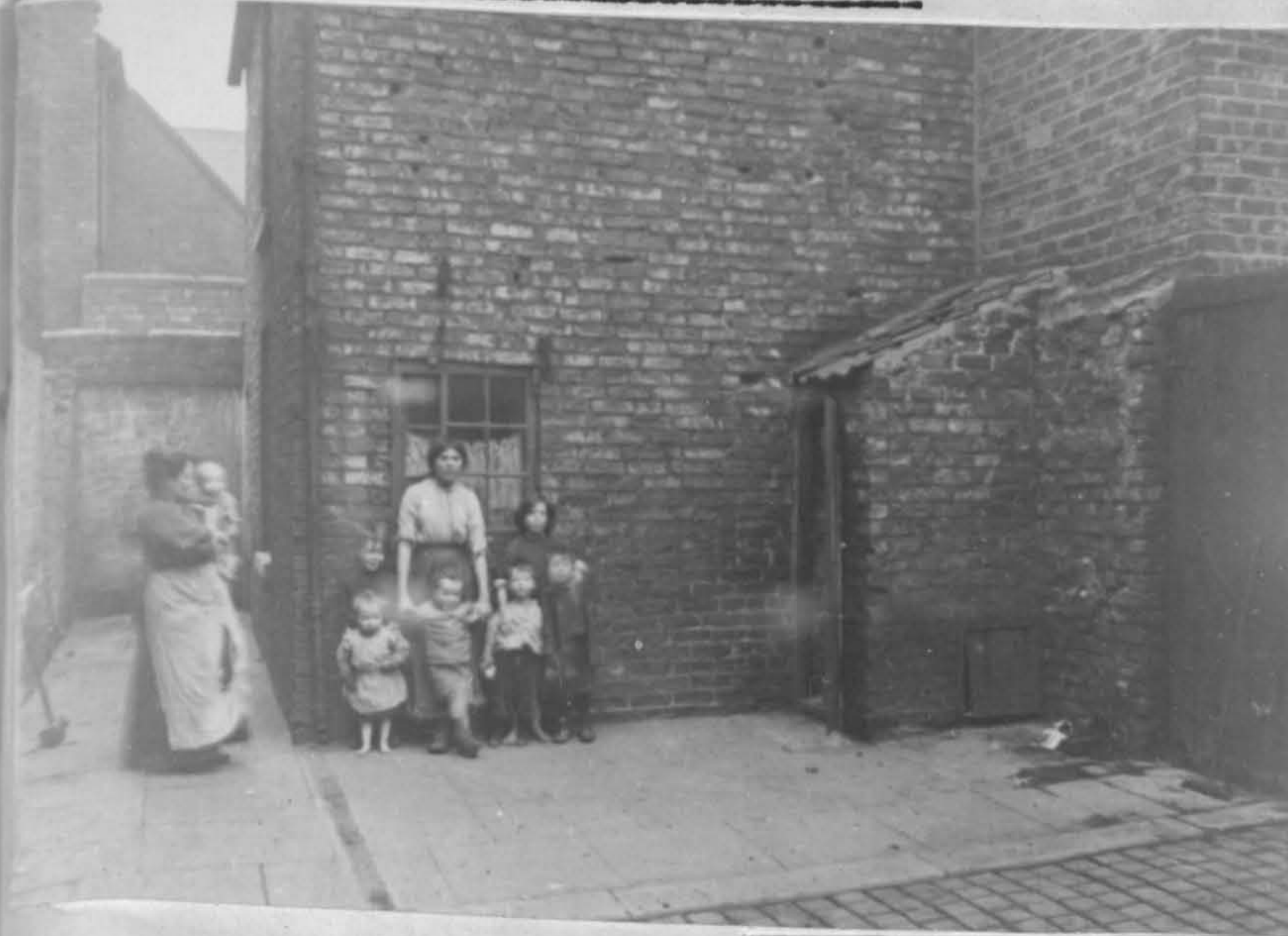
Plate 21. Robinson's Buildings off Lower East Street. This, and the two succeeding photographs, illustrate the presence, if not the prevalence, of slums around the south-east corner of the town. Thus the contrast with the north-west corner is only relative. A very careful look at the brick-work of this house will reveal the random nature of the courses, where no normal bonding system was followed, and where stretchers and headers appear in a most arbitrary manner. Such chaotic building was common in the town in the mid-nineteenth century
