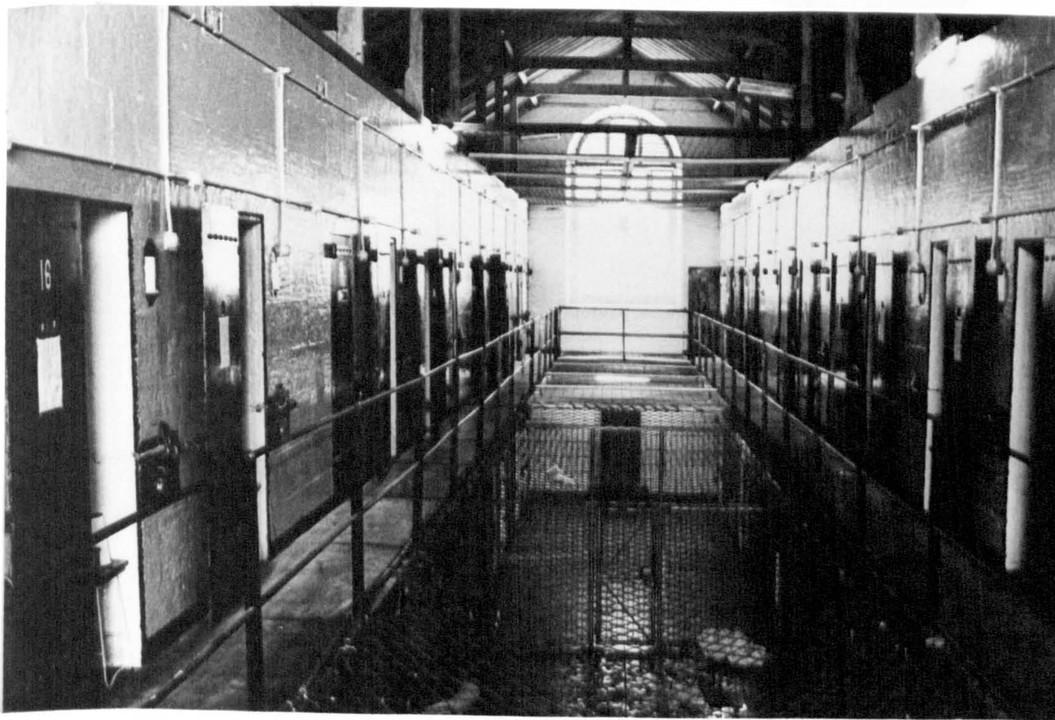
Plate 13. Maitland Gaol, NSW. Interior of 'A' wing, upper gallery level from entry end showing the same masonry, roof and fittings (except doors) as plate 12. Later doors are slightly higher than the original ones. Neg. N o JSK 75-6-6.
