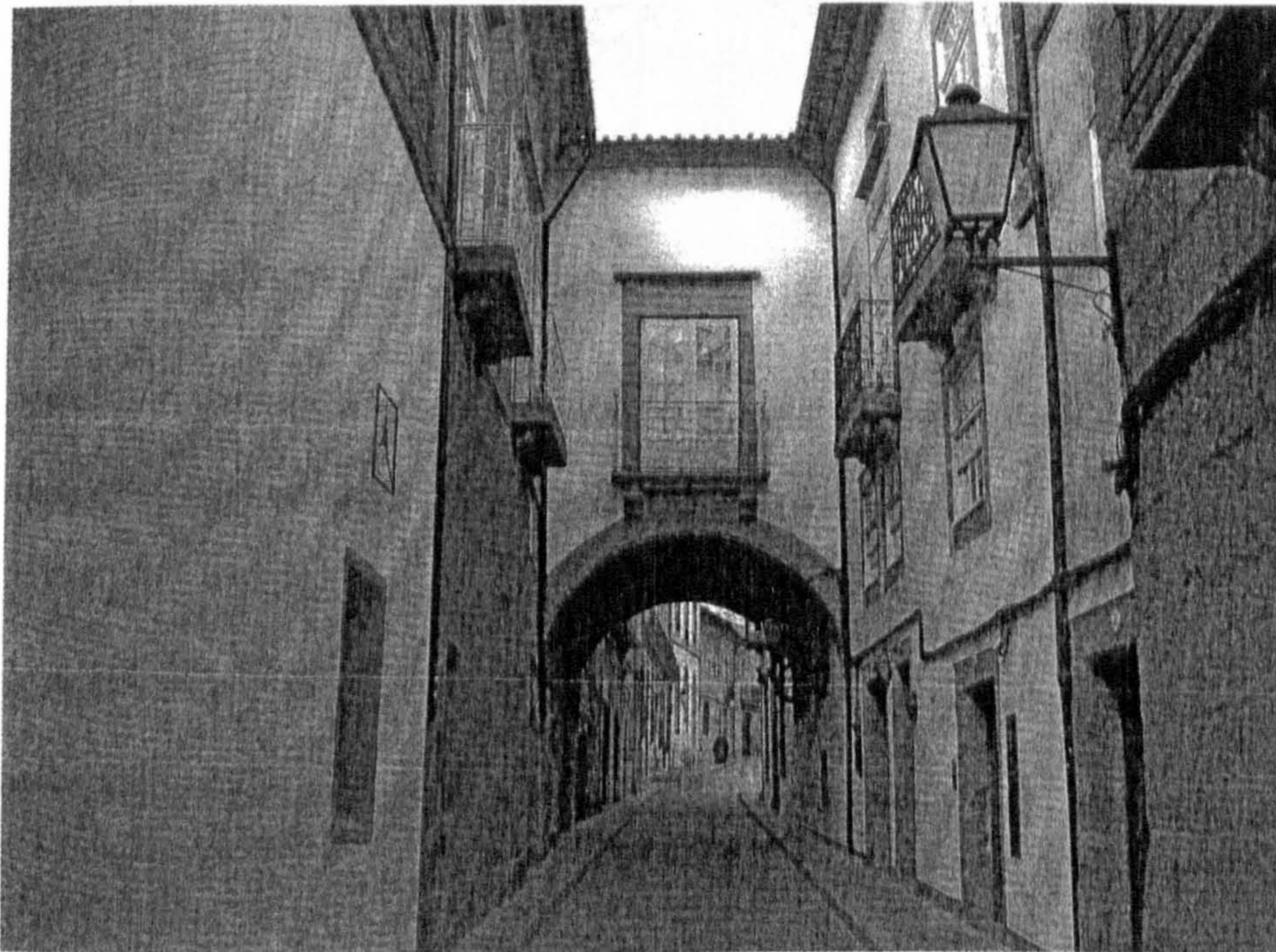
Figure 10. Passadico or bridge across a street in Guimarães with barrel vault below.
