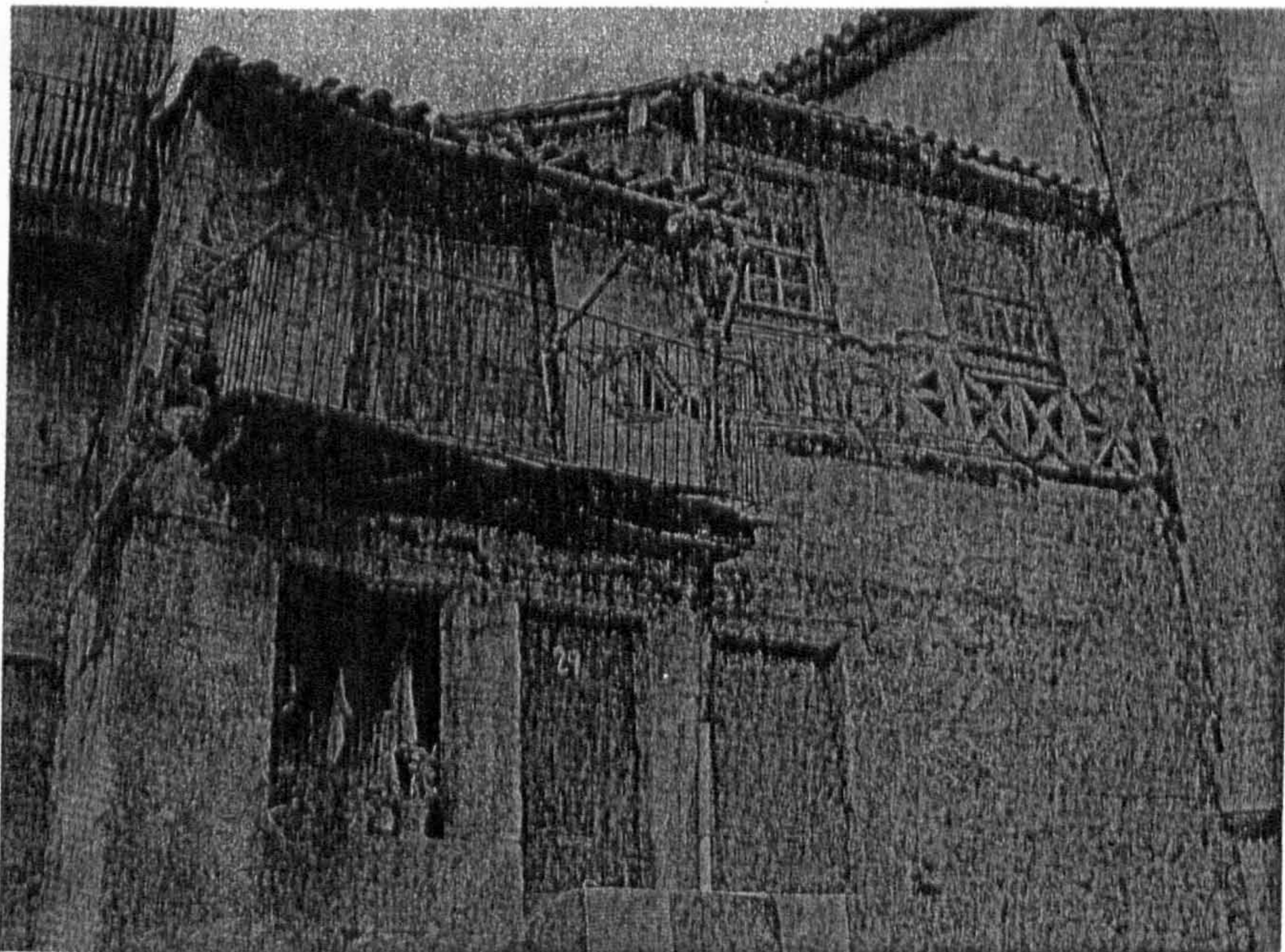
Figures 6a (above) and 6b (below). Taipa de rodizio : elaborate timber framing concealed behind plaster (now decaying to show the underlying frame), Guimarães.
