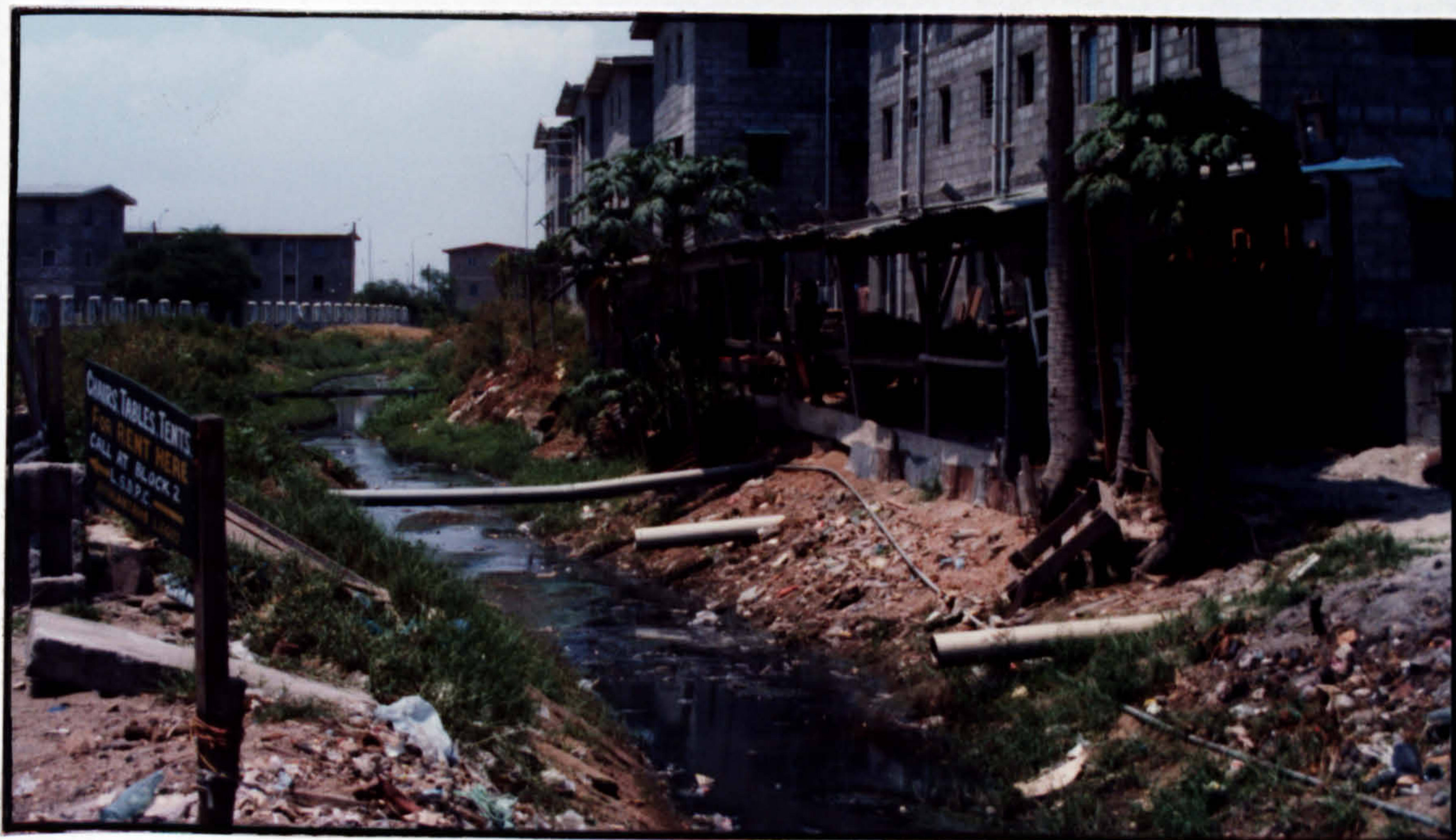
Figure 098. Drainage Channel Between Dolphin Phase 1, Stages A and B.
