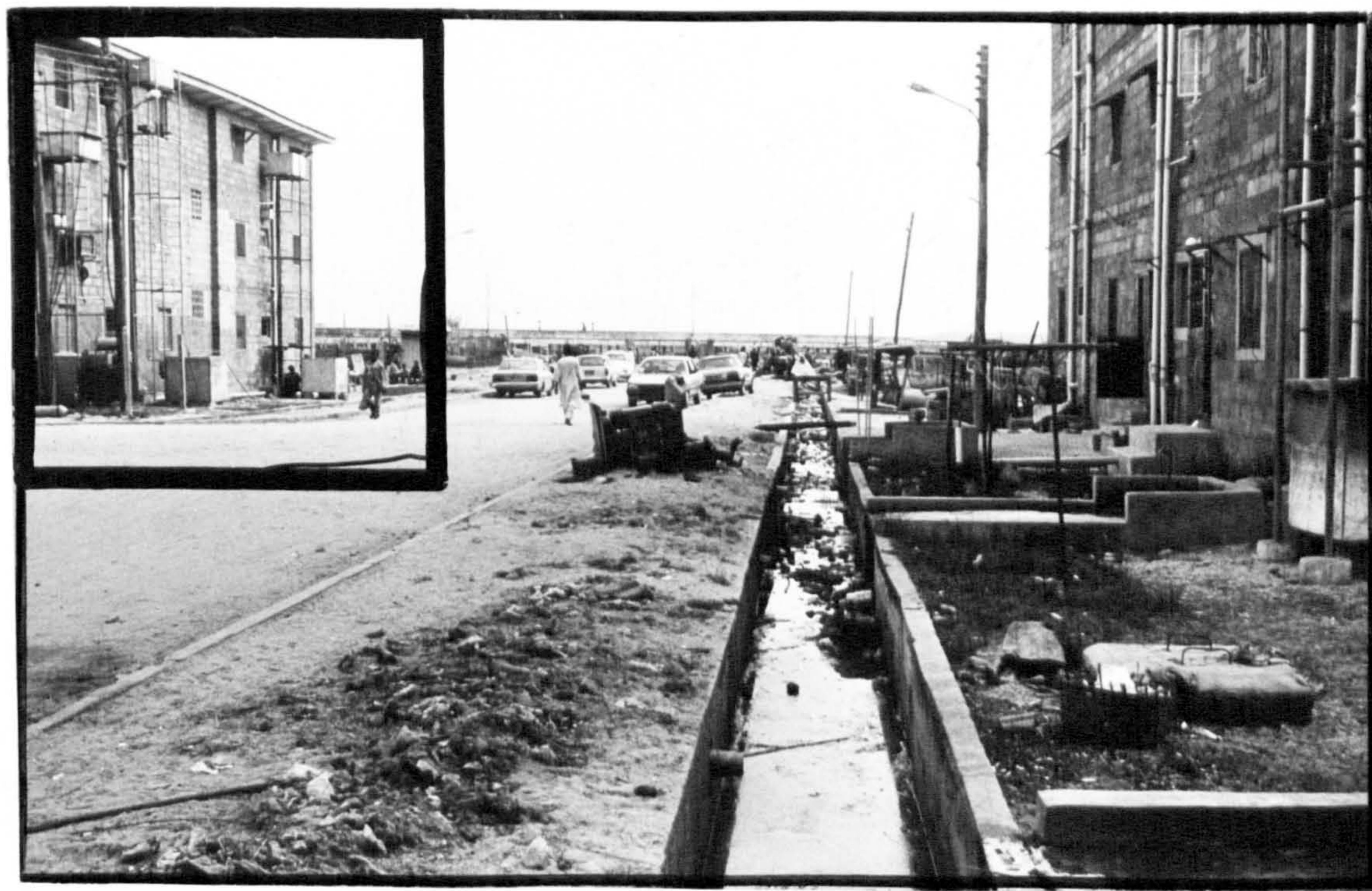
Figure 043. Water Tanks And Towers Provided By Individual Inhabitants To Overcome The Irregular And Low Pressure Water Supply, Dolphin Phase 1.
