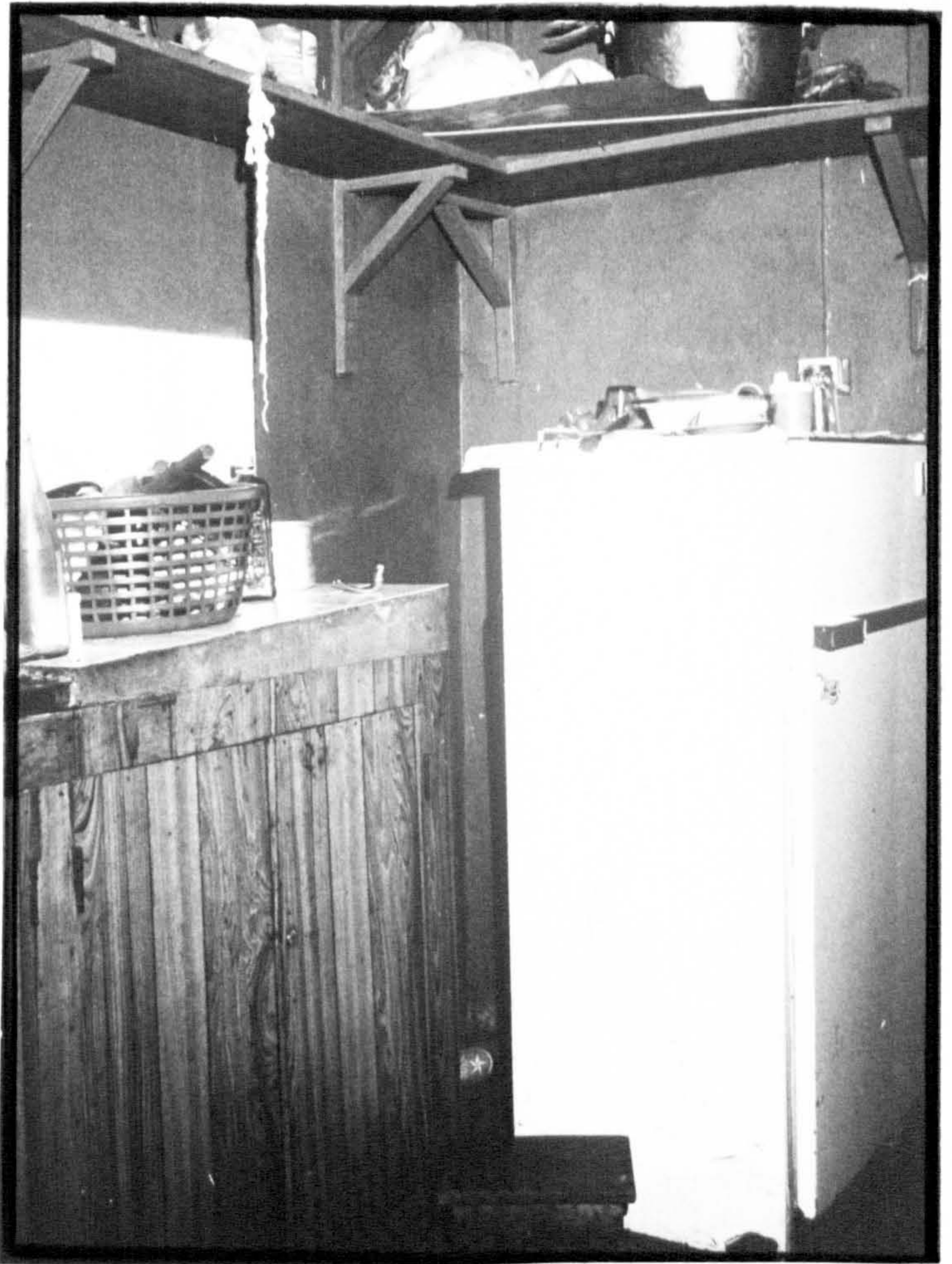
Figure 052. Well Serviced Kitchen Of a Flat in the Low Cost Housing Estate Dolphin Phase 1.
