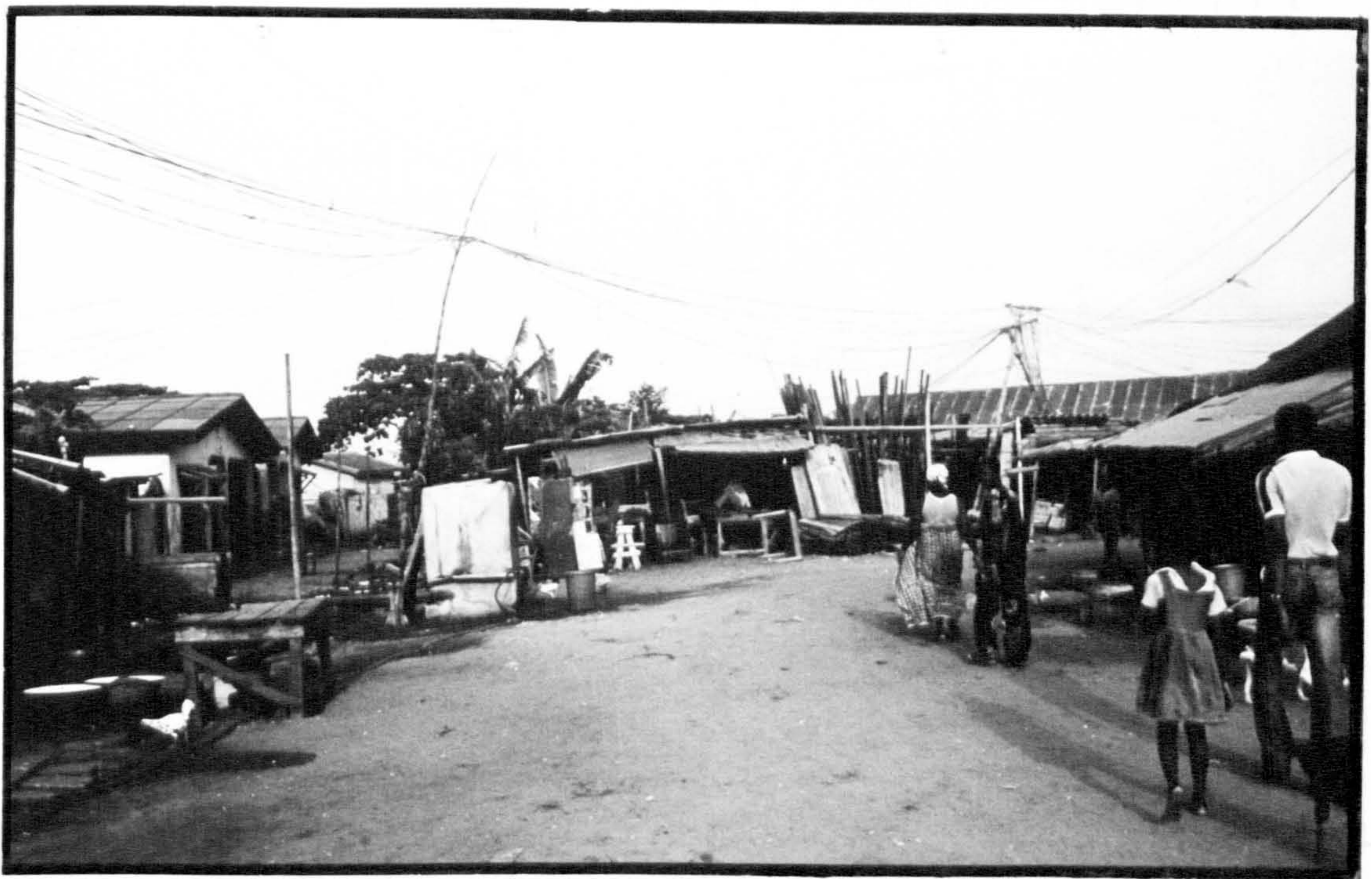
Figure 056. Private Electricity Power Lines, Maroko.
