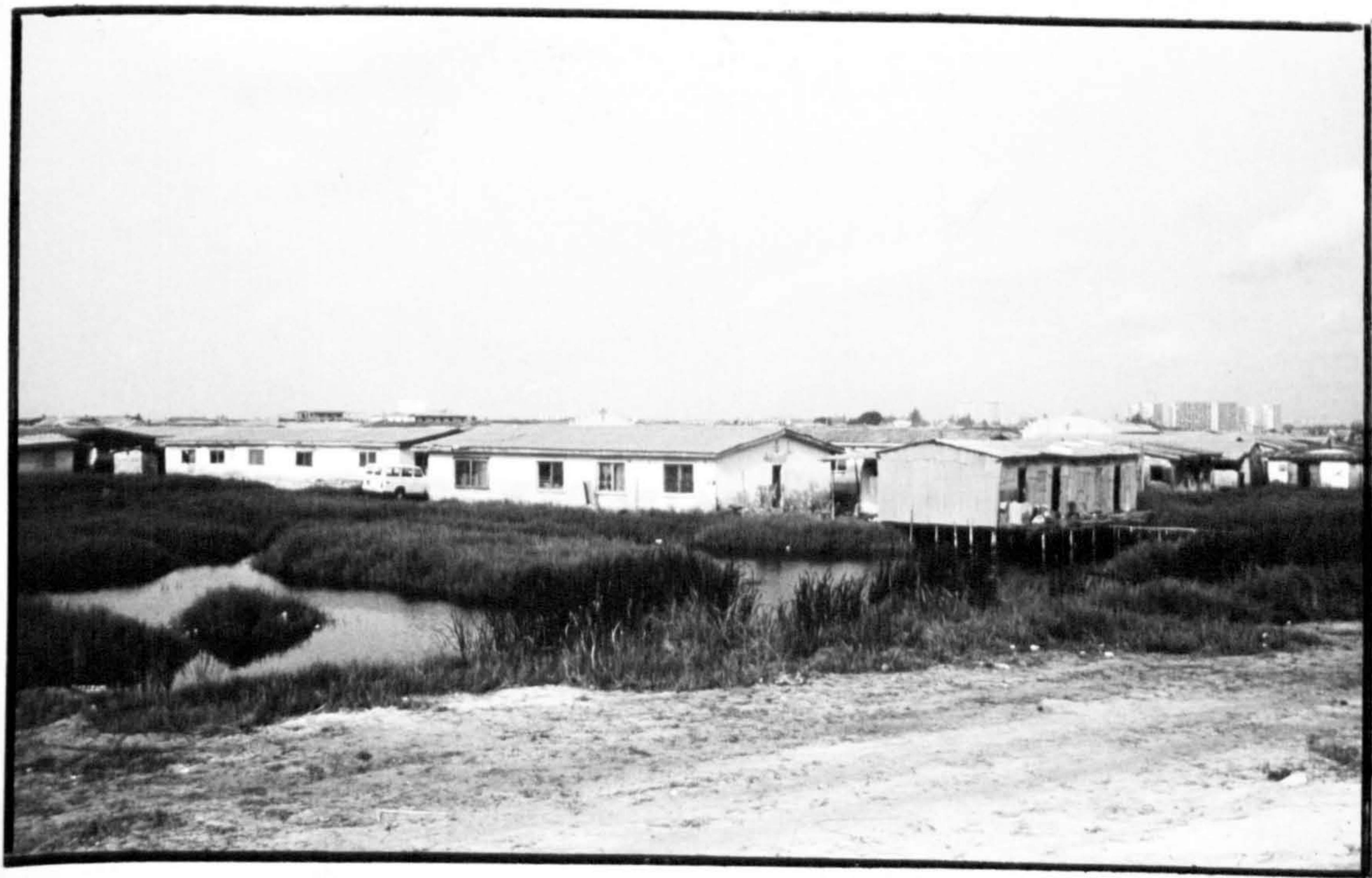
Figure 034. Flooding caused by heavy rainfall and poor drainage.
