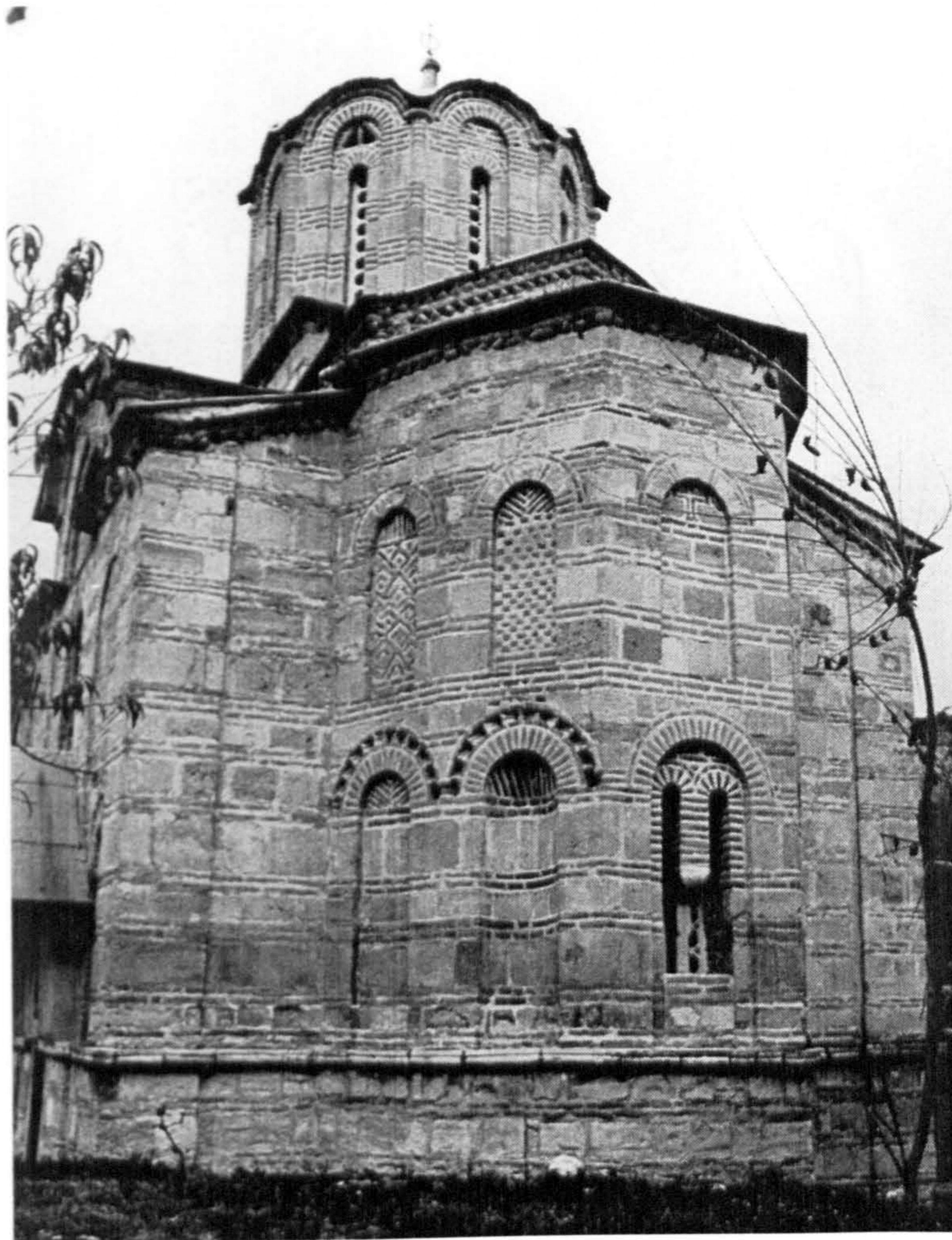
Figure 4.34 St. Dimitrija, v. Susica. Eastern facade
