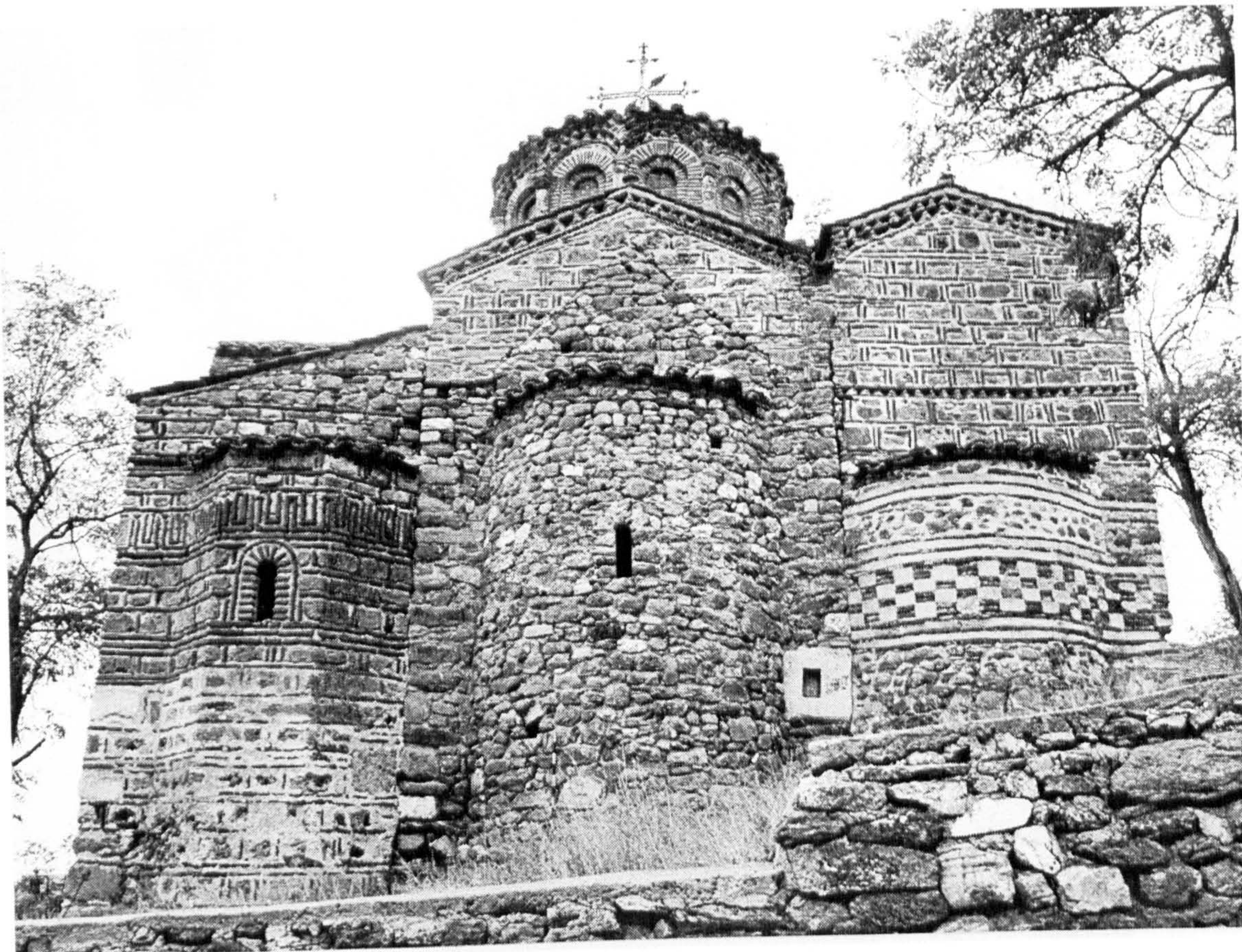
Figure 4.26 St. Dimitrija, Varos. Eastern facade
