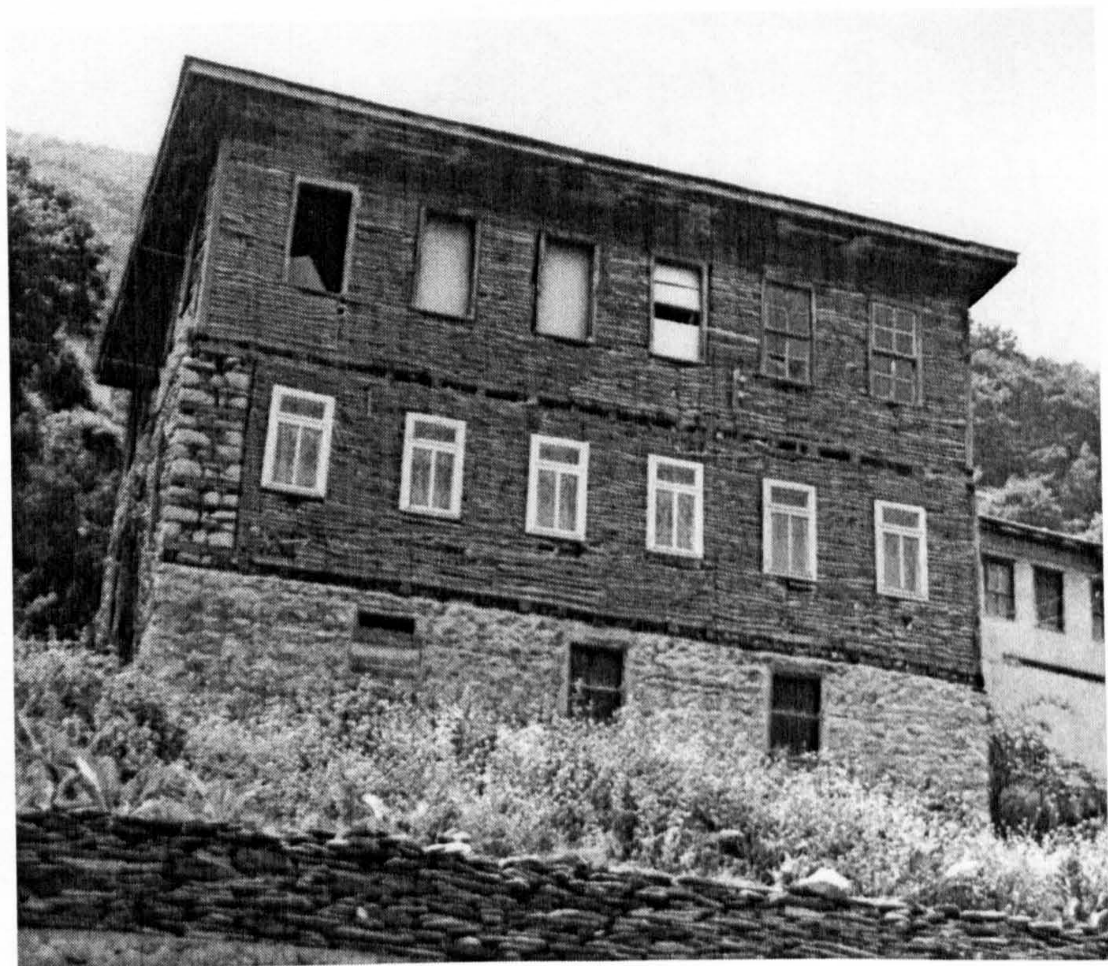
Figure 3.35 Rural house - village Gari, Rostusa
