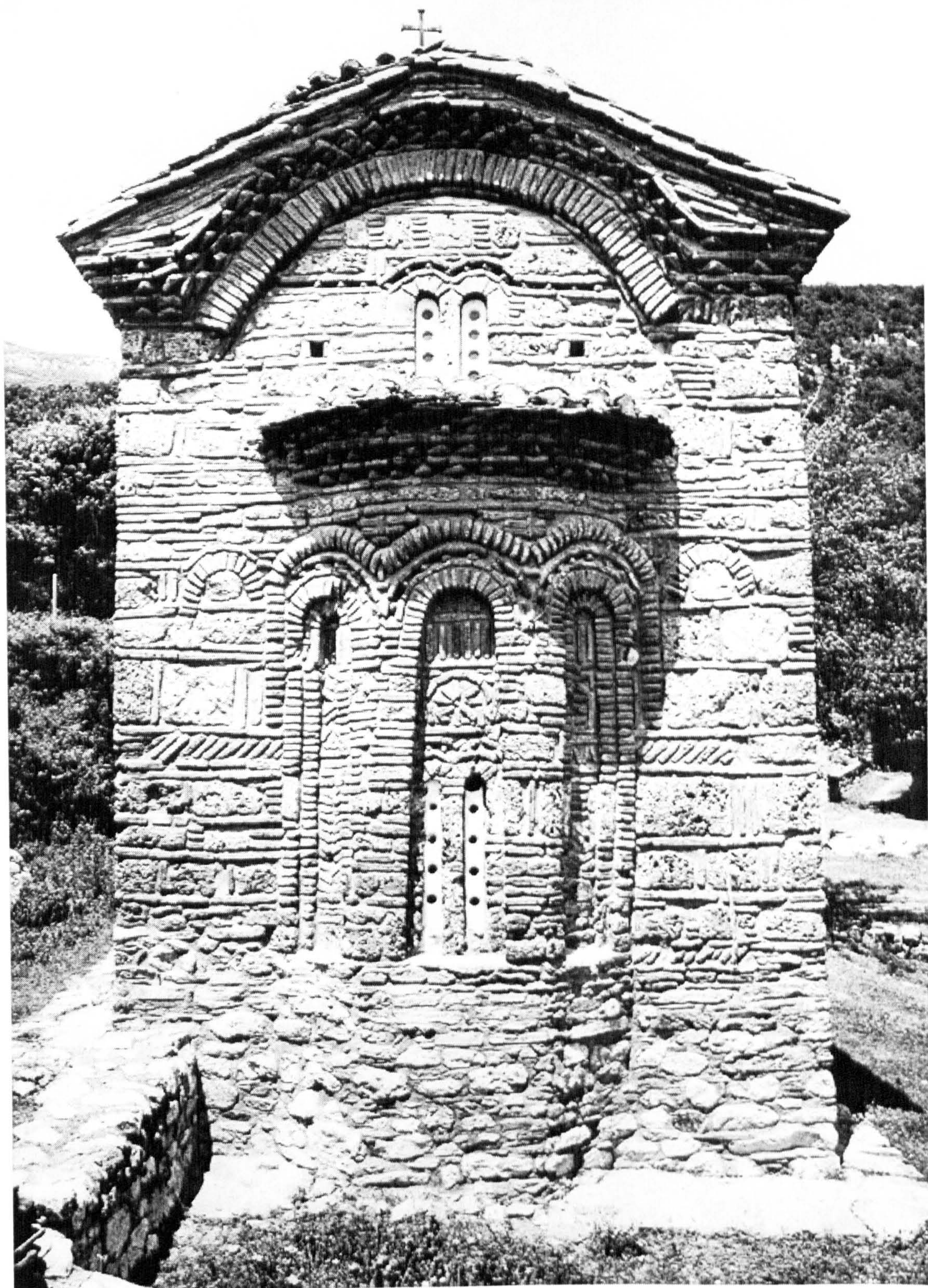
Figure 4.42 St. Georgi Poloski. Eastern facade
