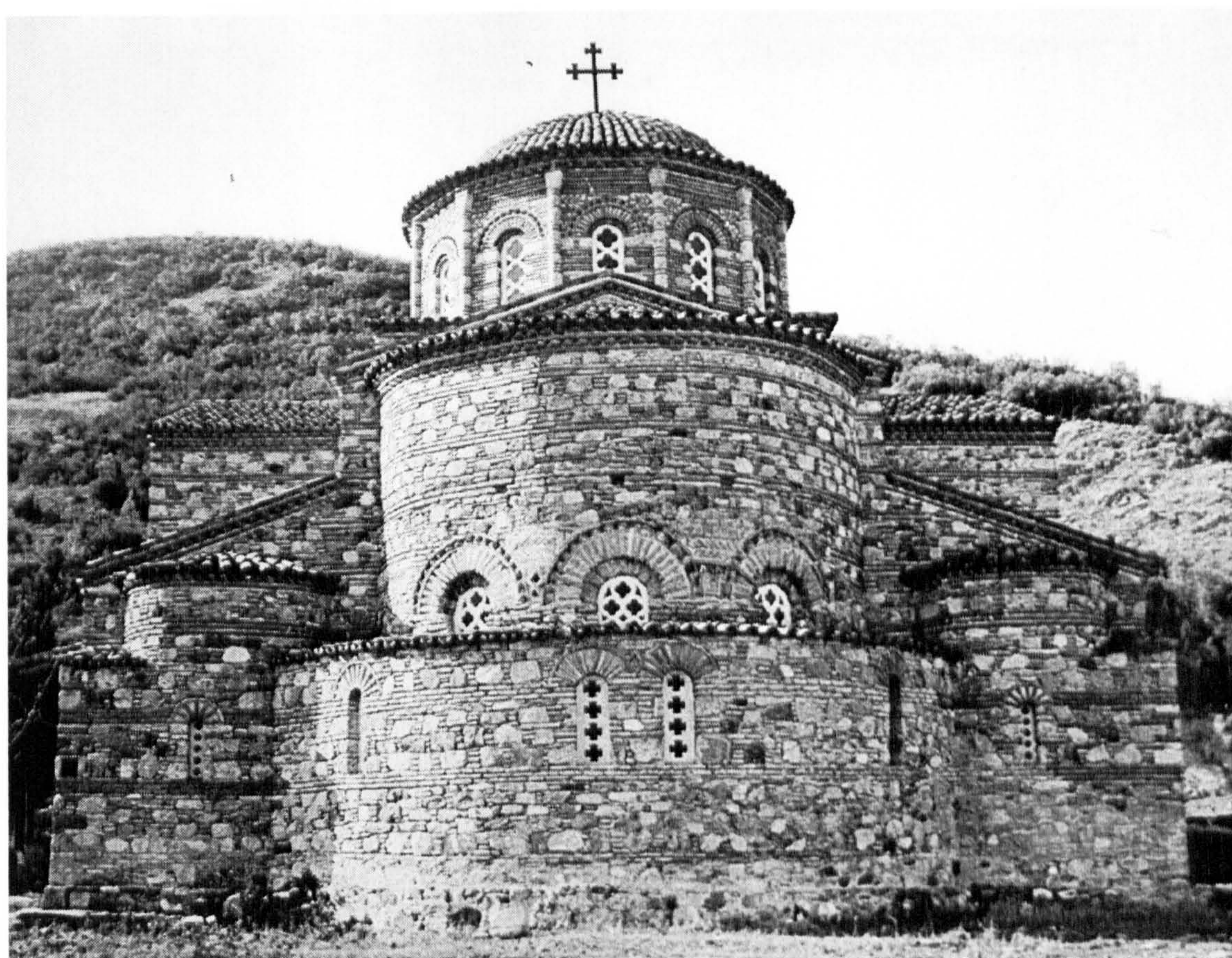
Figure 4.69 St. Leontie, v. Vodoca. East facade - after reconstruction
