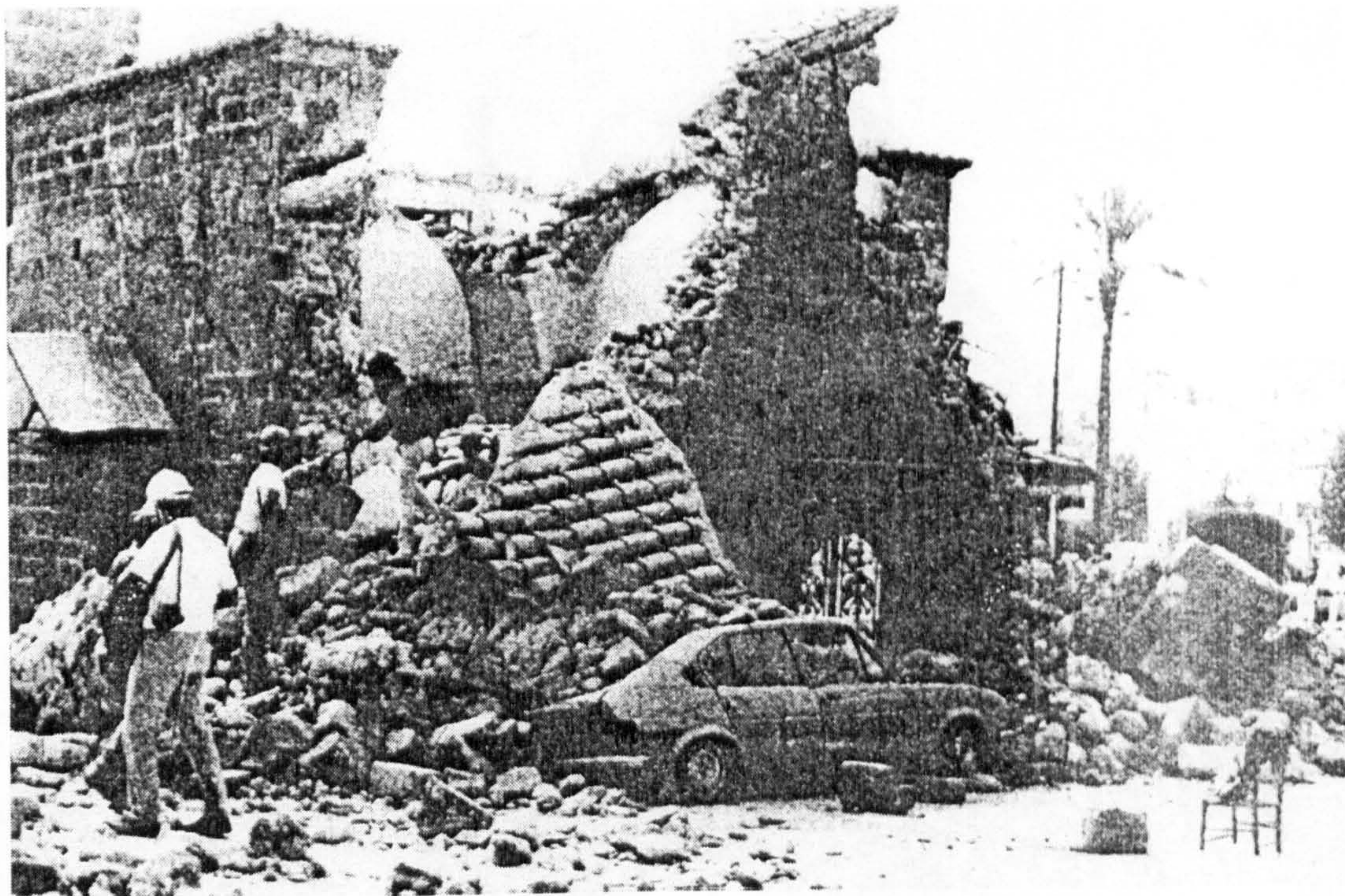
Figure 4.90 Church of the Holy Apostles, Kalamata. Damage pattern. Source: Voziatzis et.al 1990
