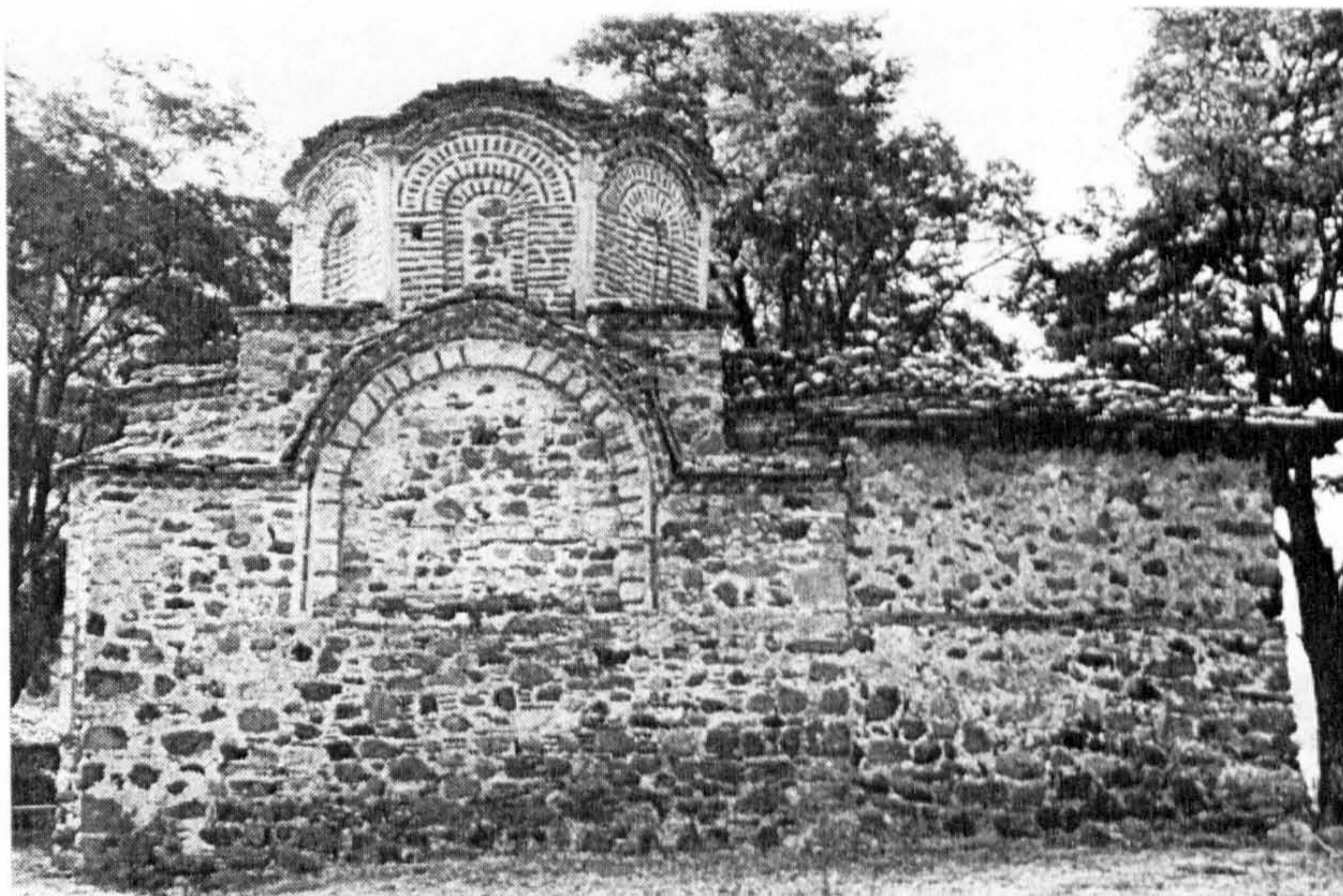
Figure 4.87 St. Christ, v. Mborje near Korca, Albania. North facade after restoration.
