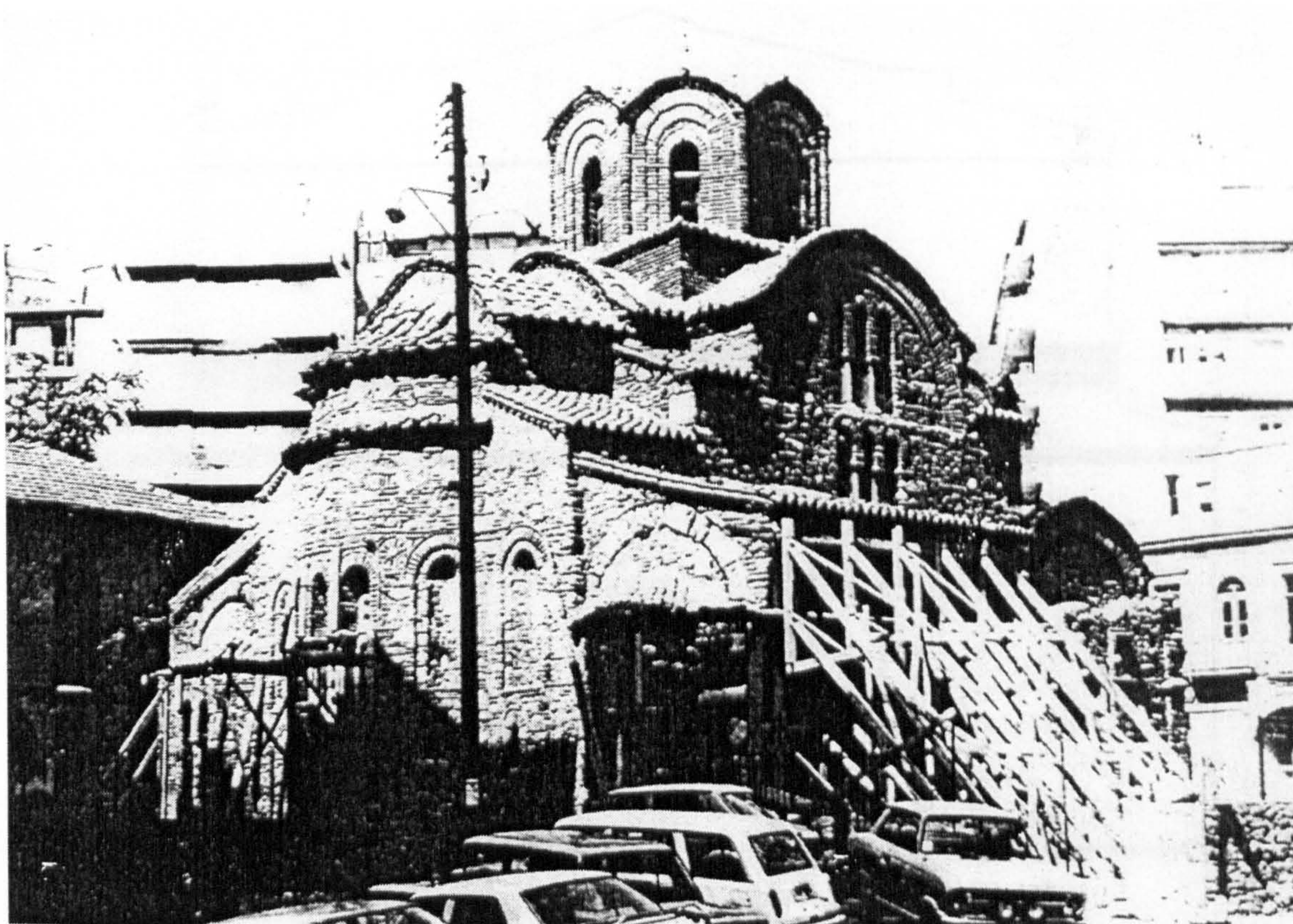
Figure 4.92 St. Panteleimon, Thessaloniki. Temporary supporting of Northern wall.
