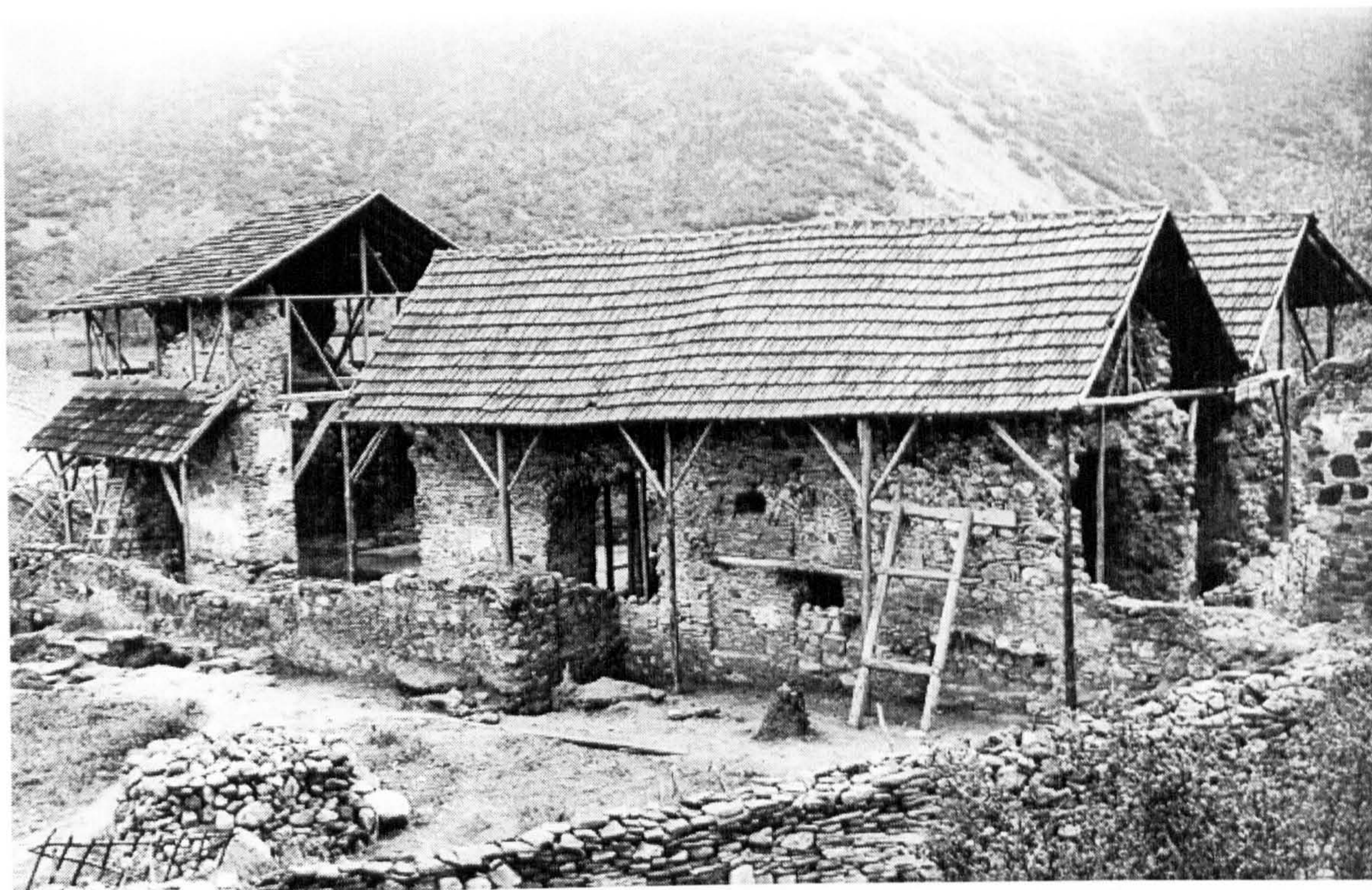
Figure 4.66 St. Leontie, v. Vodoca. North facade - before reconstruction
