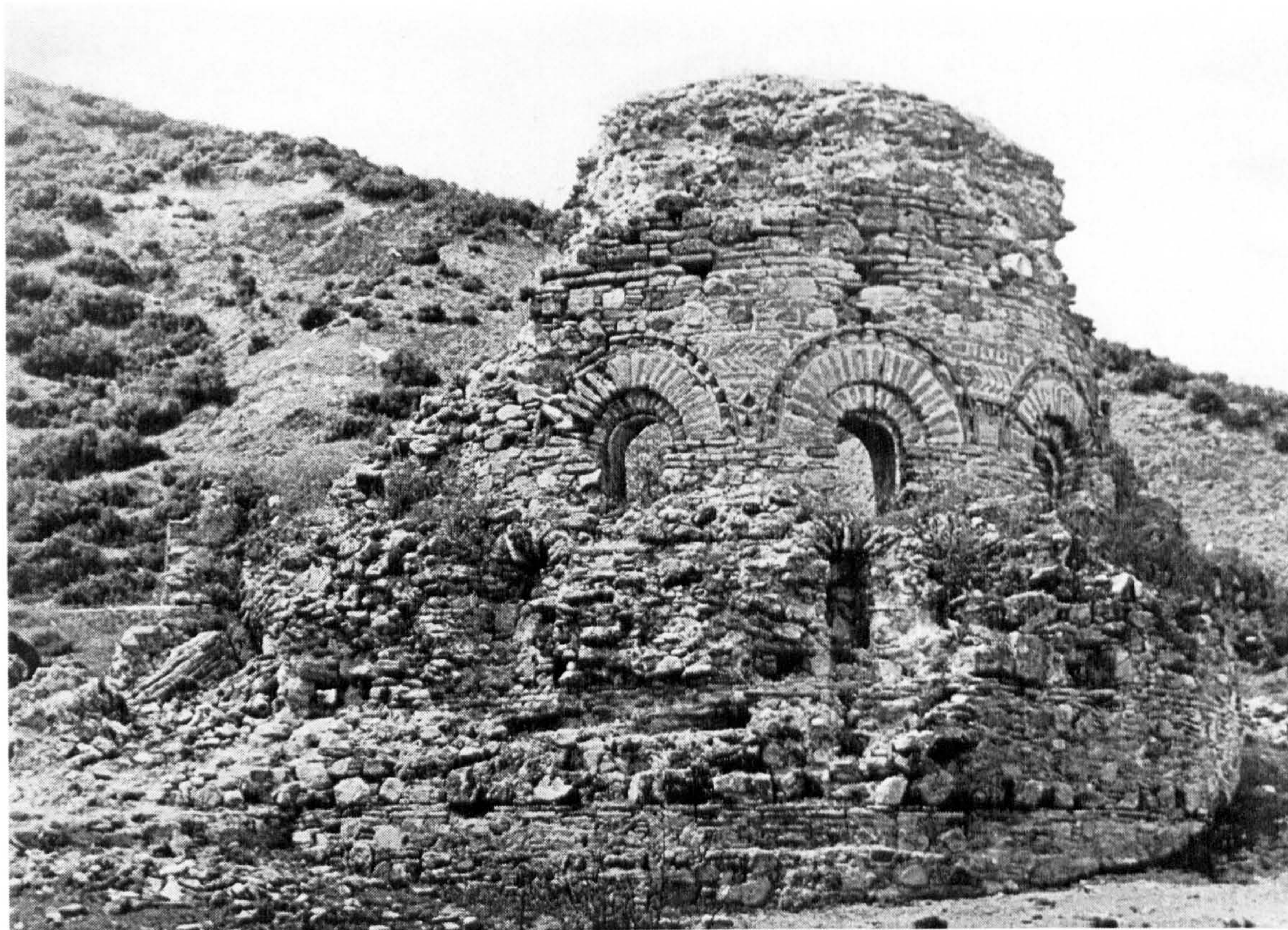
Figure 4.68 St. Leontie, v. Vodoca. East facade - before reconstruction
