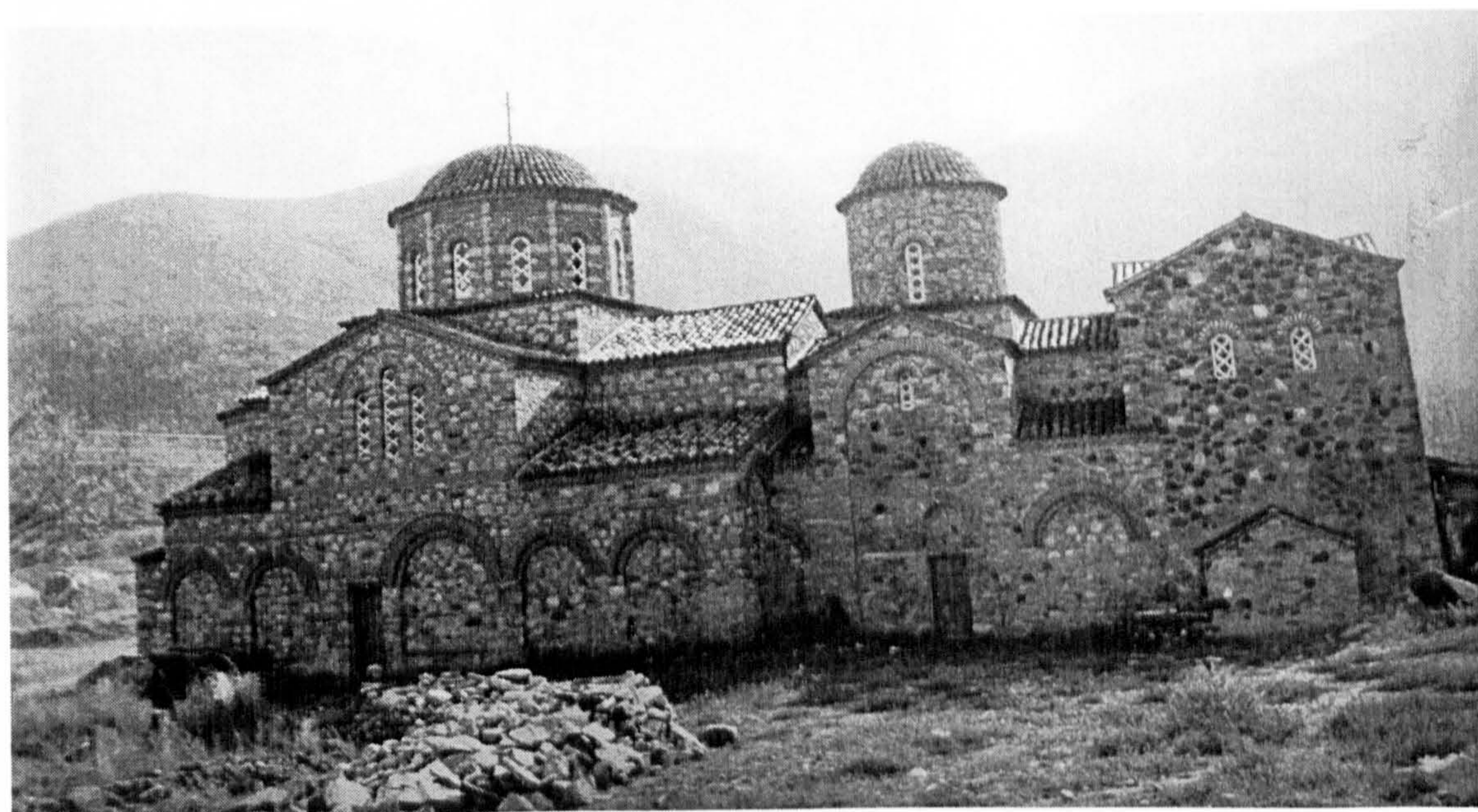
Figure 4.67 St. Leontie, v. Vodoca. North facade - after reconstruction
