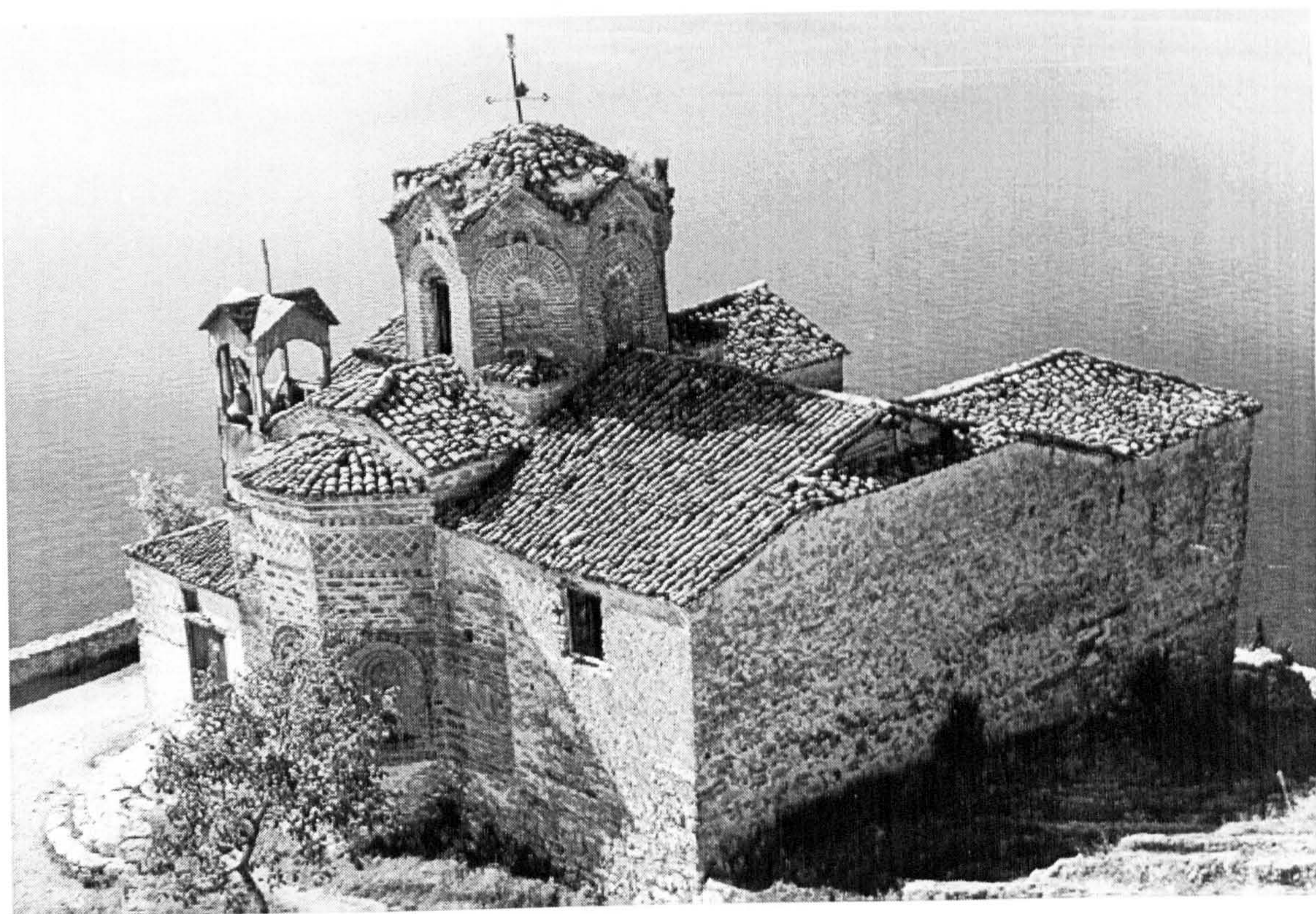
Figure 4.57 St. Jovan Kaneo, Ohrid. Before the restoration
