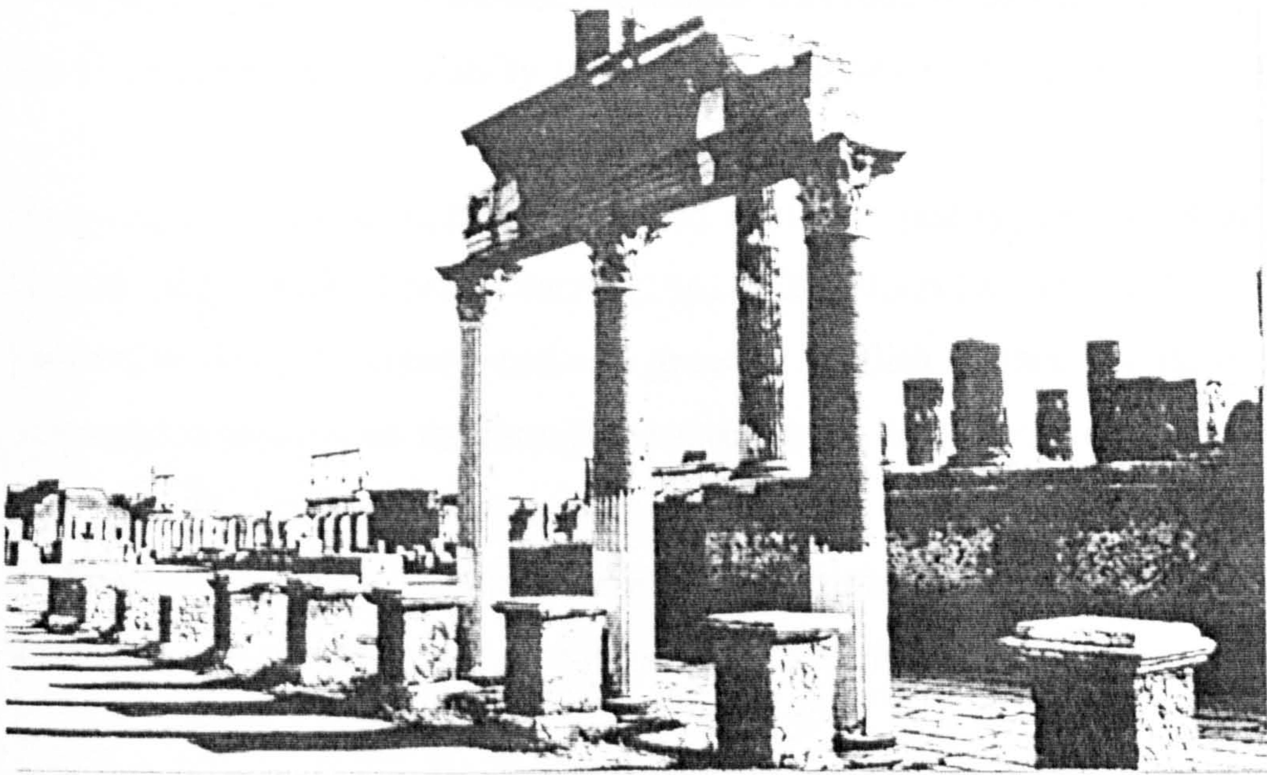
Fig. 2.13 The forum at Pompeii showing partial restoration
