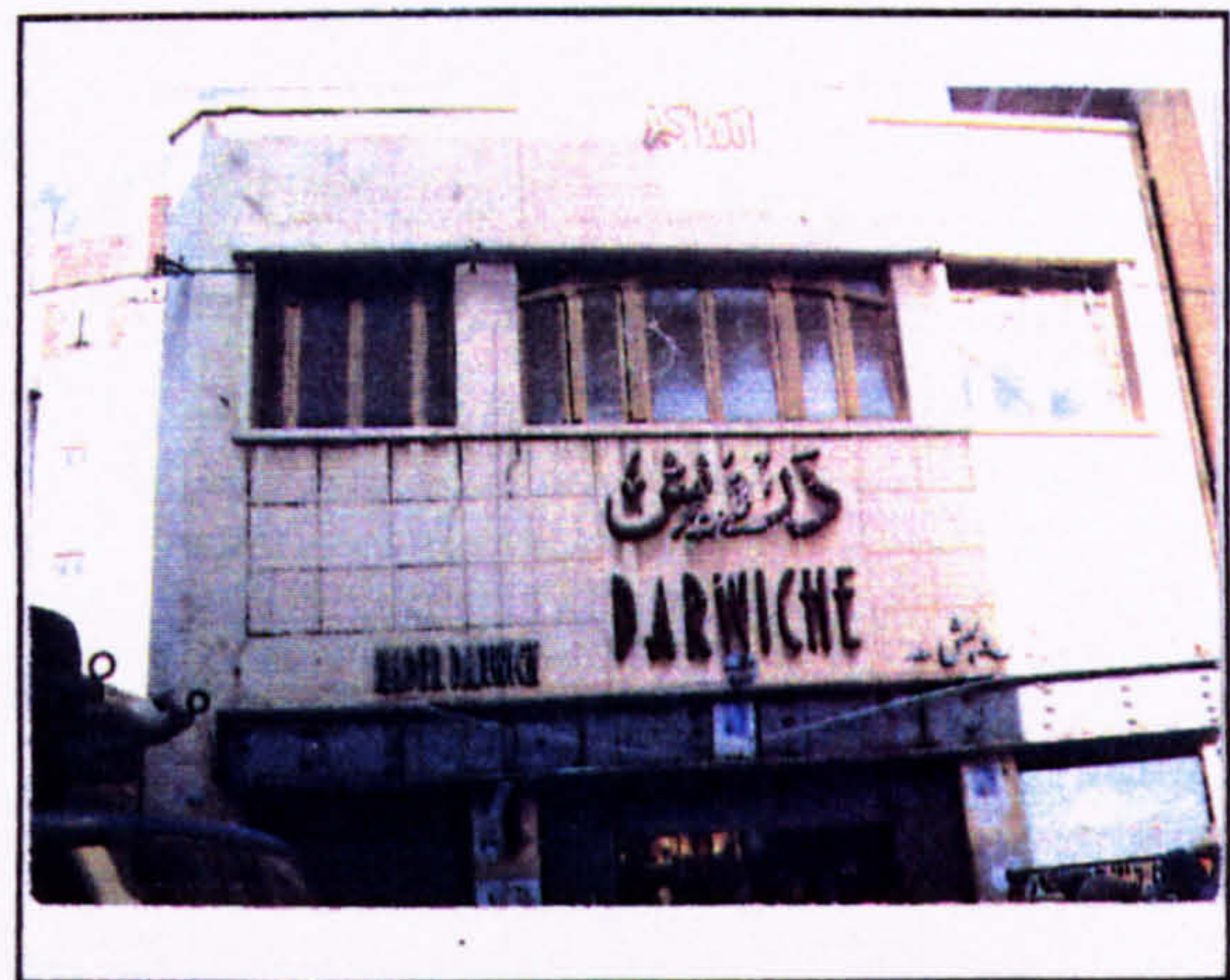
Fig.8-18, the street facade; a unique example of very "early-modern" architecture in Alexandria
