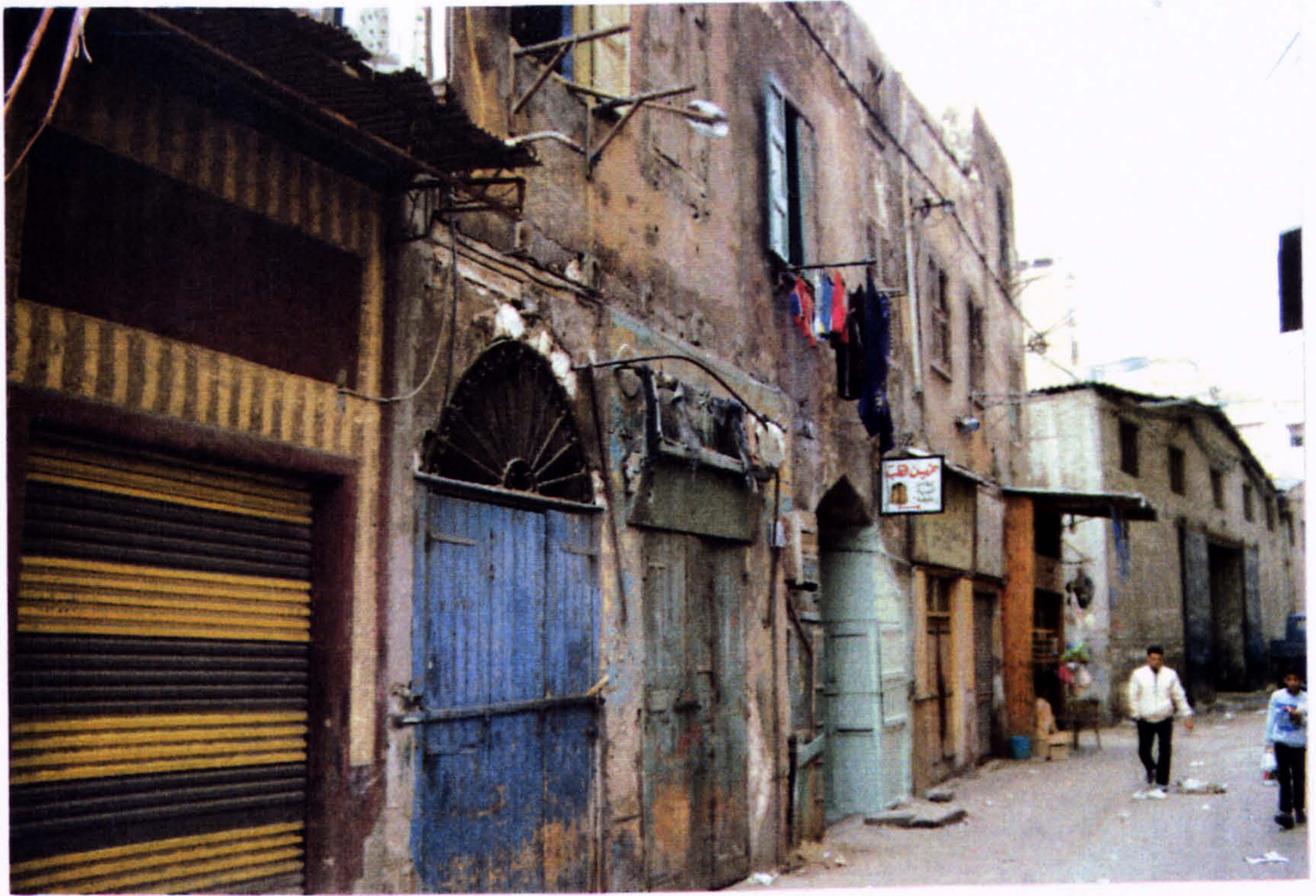
The building as seen from the street
