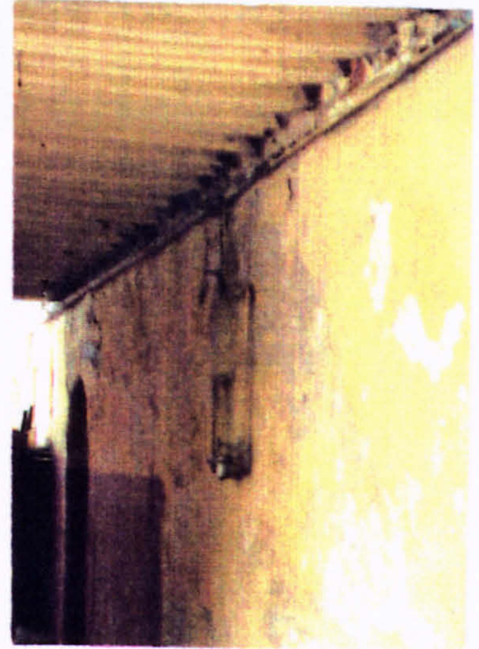
Fig.8-14, Right, inadequate installation for water supply and drainage leading to damp stains; unsightly wiring for electricity supply; Left, stone masonry; badly deteriorating timber tie-beams.
