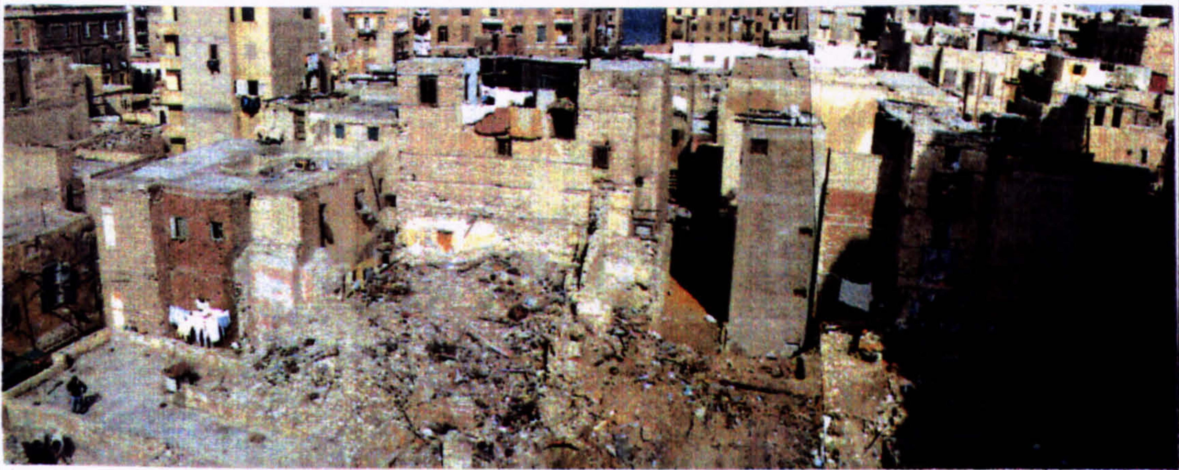
Fig.8-24, Waqf Gemaiee, the present condition: a real waste of resources
