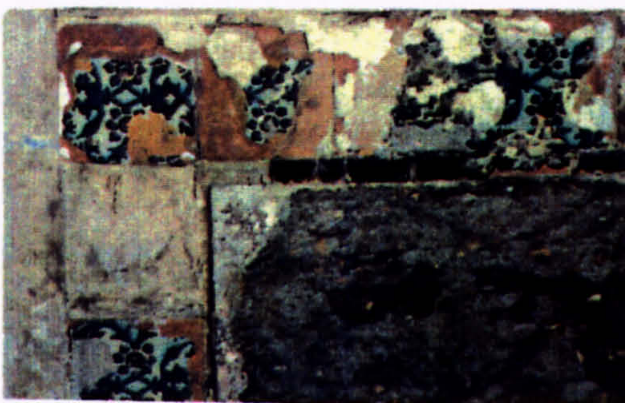
Fig.8-15, Right, improper repair and replacements of tiles; Left, badly deteriorating tiles with problems of salt crystallisation, causing scaling and powdering of the surface; marble tiles, in the middle, are showing undesirable discolouring and the loss of hardness and polish of the surface layer.
