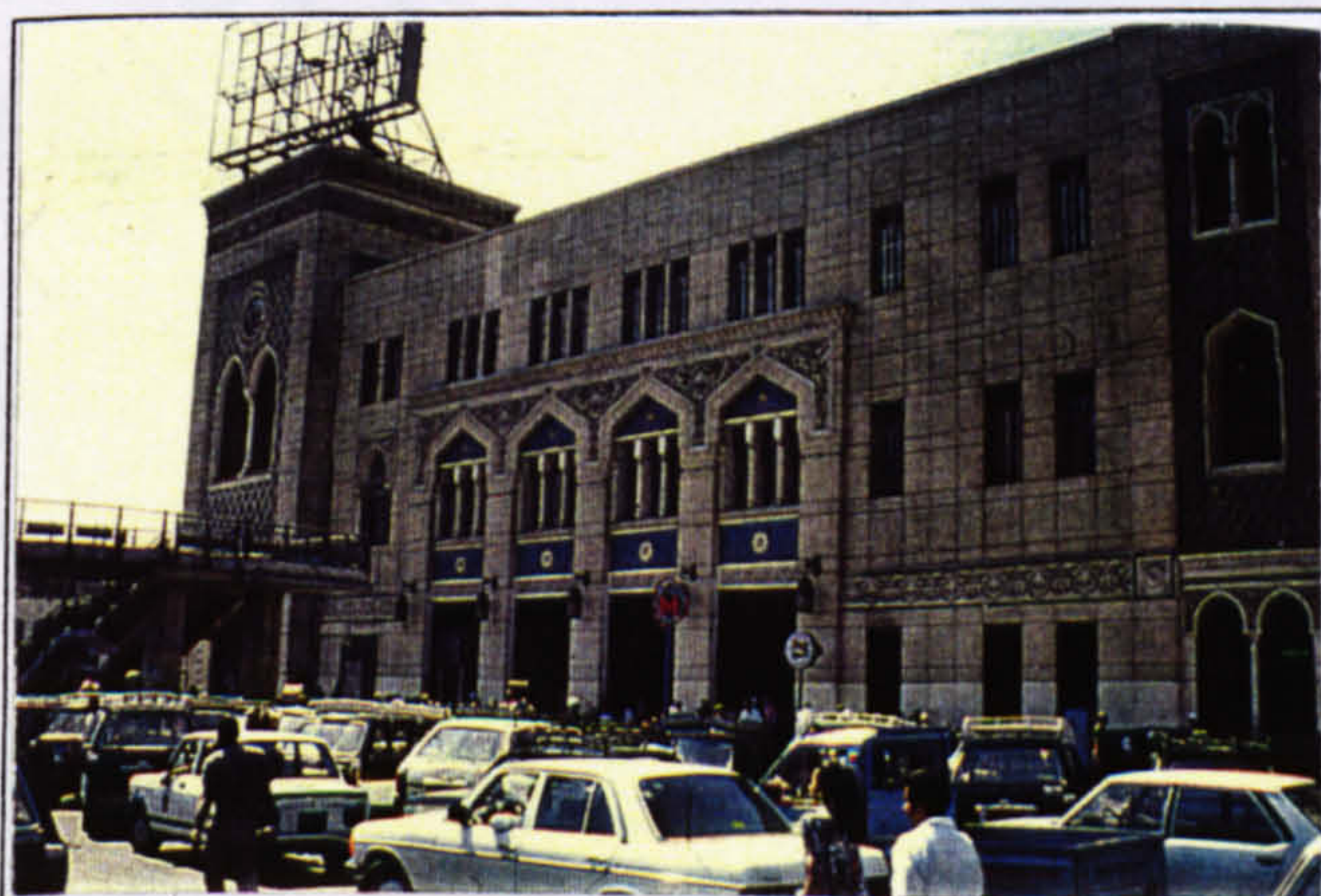
Fig. 98 Ramses Railway Station, south-east elevation.
