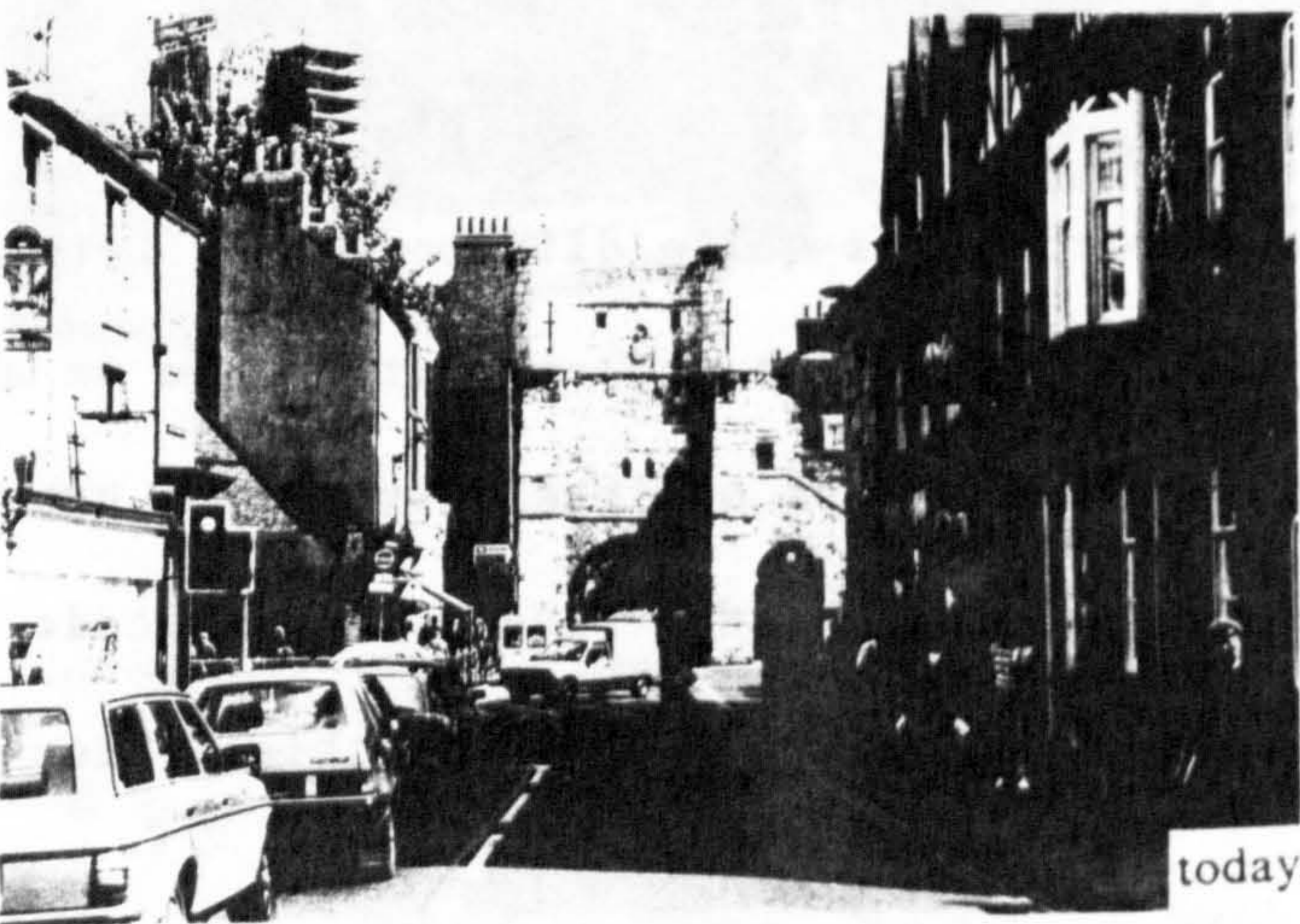
Fig.6.34 - Bootham Bar. Source: Palliser, 1979, & author.
