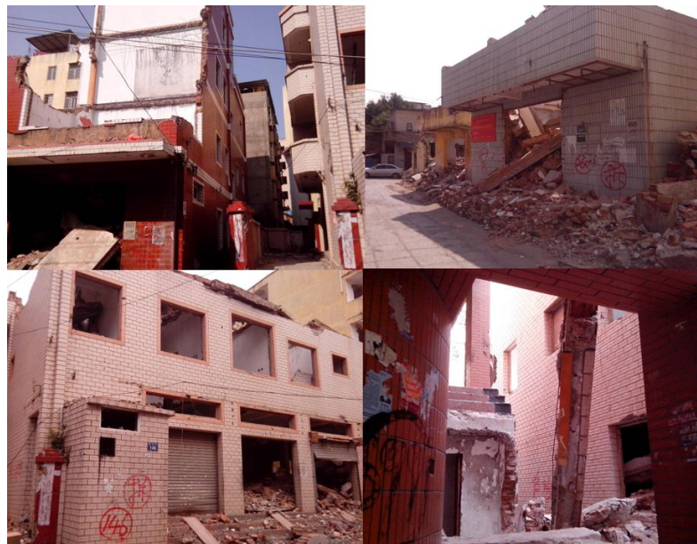
Image 7.3 Demolished houses at May 2013
