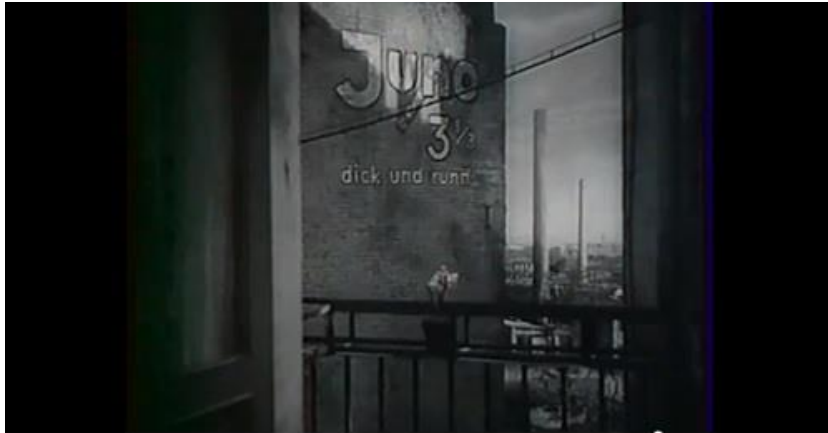
Figure 3: The lack of bomb damage in Unter den Brücken 59
