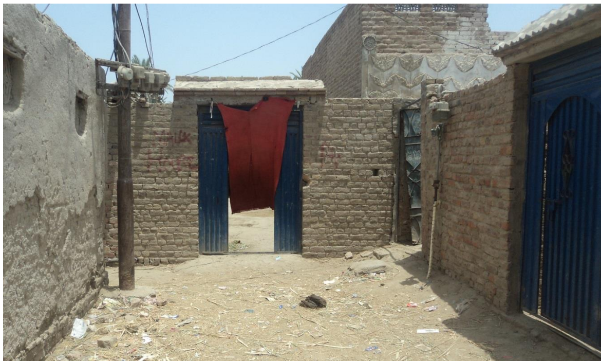
Figure 15: Houses Built very Close
