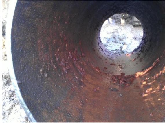
Figure 6.39: The TM-WB main was drained down during September 2012 to repair a leak. This allowed for the visual inspection of condition of the pipe wall. Part of the DI section is shown here.
