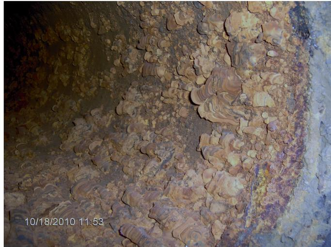
Figure 2.5: The internal surface of a  $\varnothing=350\text{mm}$  unlined *DI* trunk main, taken after the main had been drained down. Image supplied by Wessex Water.
