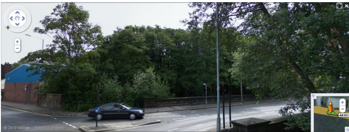
Figure 20: Malin Bridge before the work, from Holme Lane looking towards Burgon and Ball (photo courtesy of Google Streetview ©2010 Copyright Google Streetview/Bluesky)
