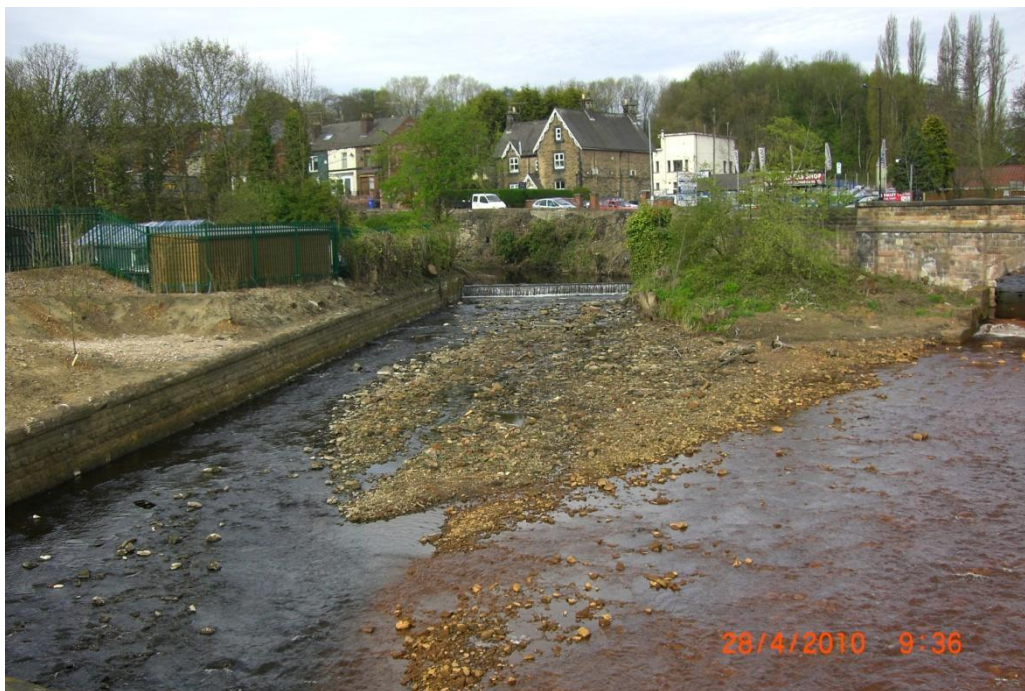
Figure 14: Malin Bridge (Photograph author's own)
