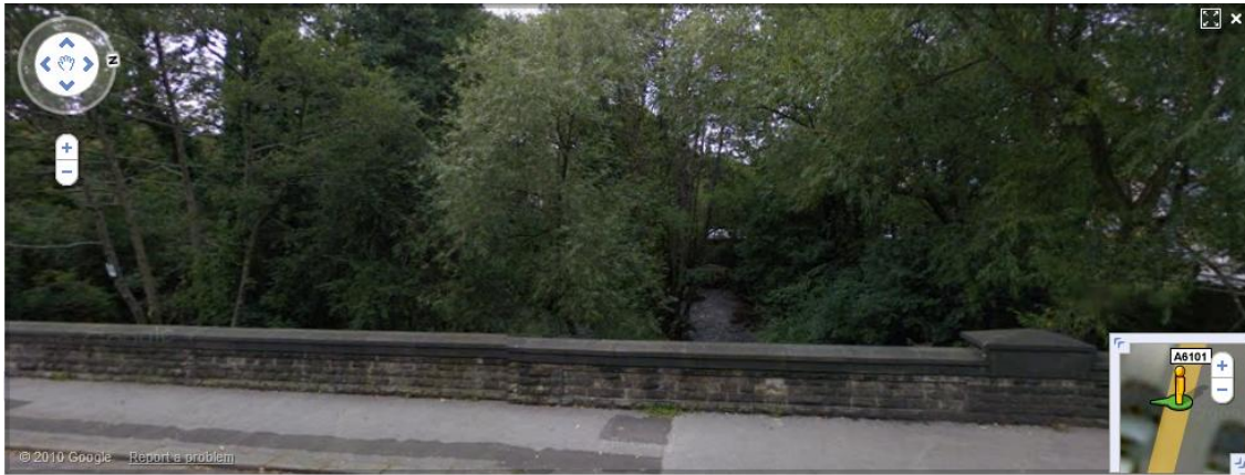
Figure 19: Malin Bridge before the work, from Rivelin Road overlooking the main site (photo courtesy of Google Streetview ©2010 Copyright Google Streetview/Bluesky)
