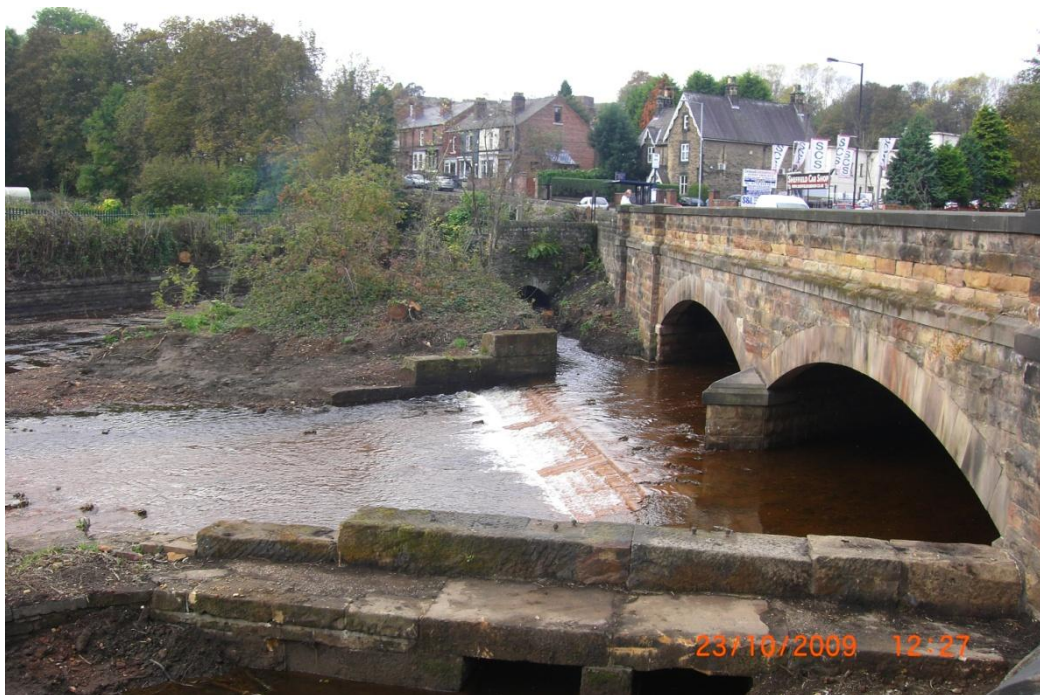
Figure 21: Malin Bridge (Photograph author's own)
